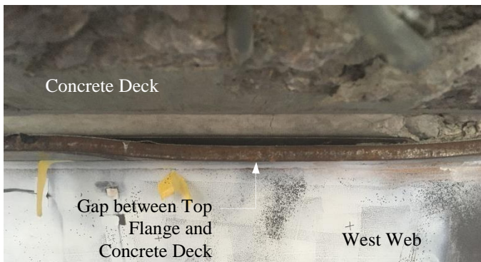
Figure 5-42 - Gap between Top Flange and Concrete Deck - Tub #3
