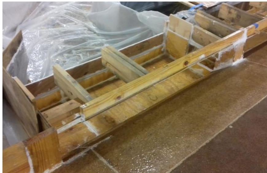
Figure 76: Front view of the box used to control tail water (Level A setup).
