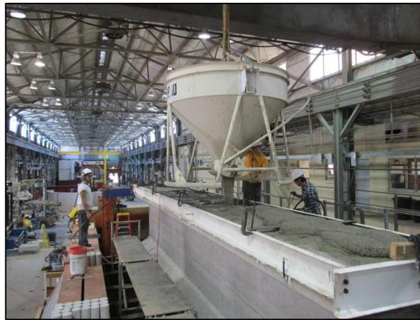
(b) Casting the deck concrete
