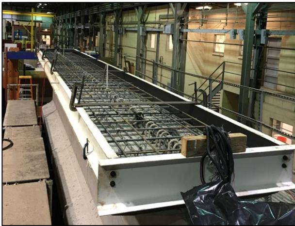
(a) Deck reinforcement and formwork
