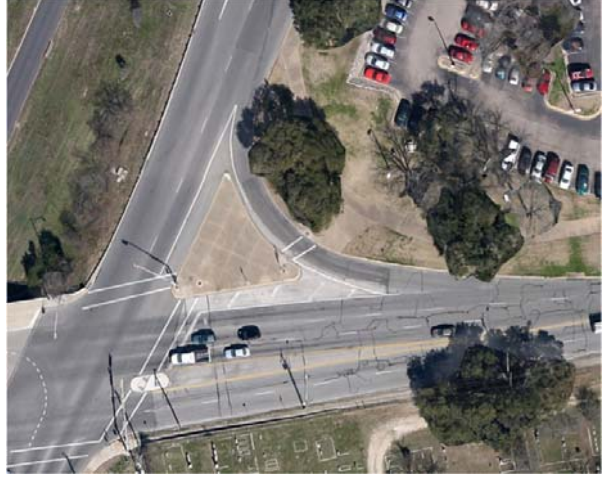
Figure 44: IH 35 NBFR and MLK Dr, Austin, TX (Google Maps, 2014)
