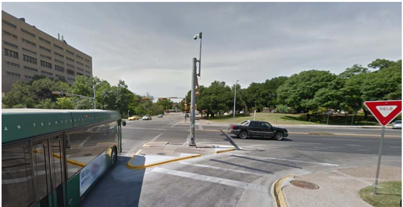
Figure 29: Channelized Right-Turn Lane at Northbound San Jacinto and Dean Keeton (Google Maps, 2014)
