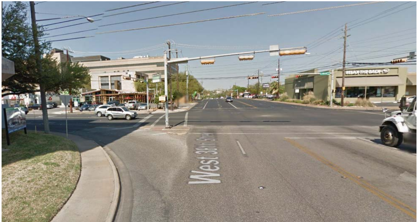
Figure 31: Channelized Right-Turn Lane at Northbound Lamar and 38th Street (Google Maps, 2014)
