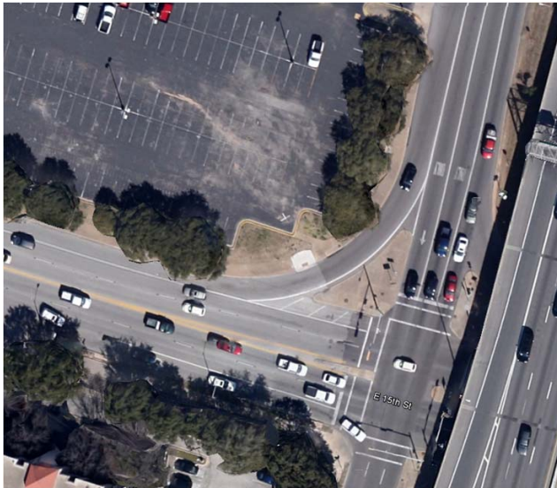
Figure 47: IH 35 SBFR and 15th St, Austin, TX (Google Maps, 2014)
