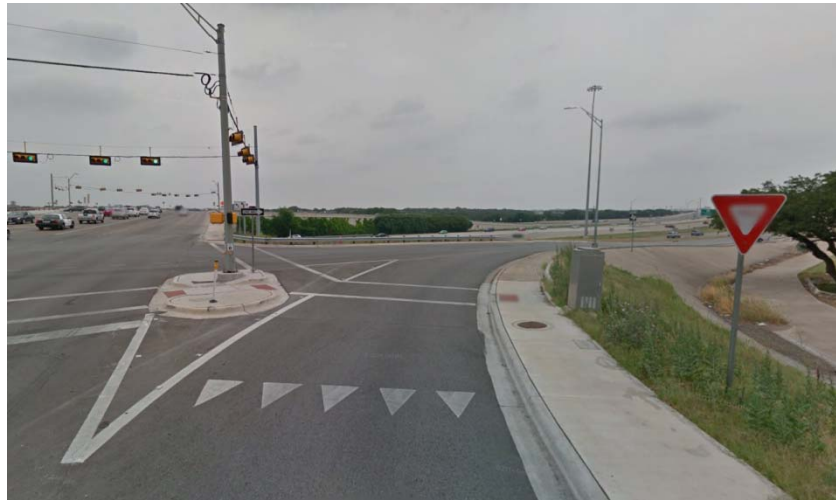
Figure 57: Parmer Lane and MoPac Expressway Northbound Frontage Road (Google Maps, 2014)
