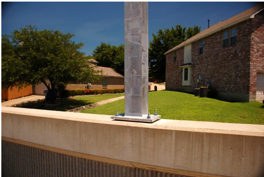
Figure 7.7 Noise wall installation detail on the east side (June 13, 2019)
