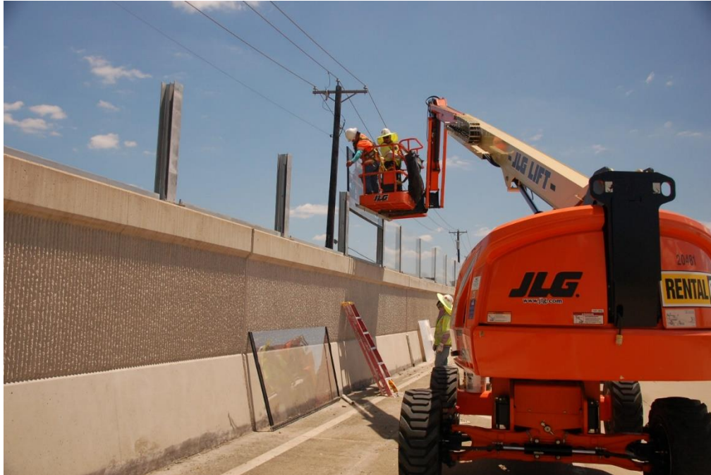
Figure 7.27 East side noise wall installation. Acrylic panel placement (July 24, 2019)
