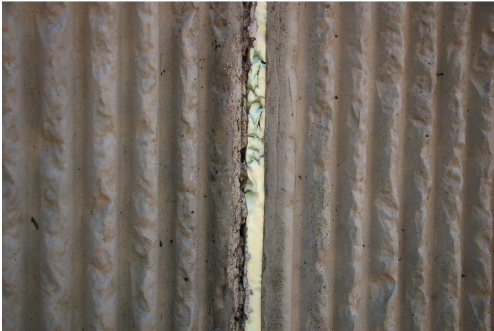
Figure 7.34 Expansion joint with sealant material in good condition
