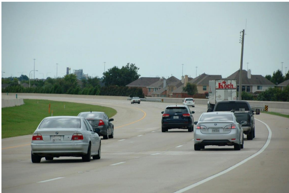
Figure 1.6 View of the southbound main lanes
