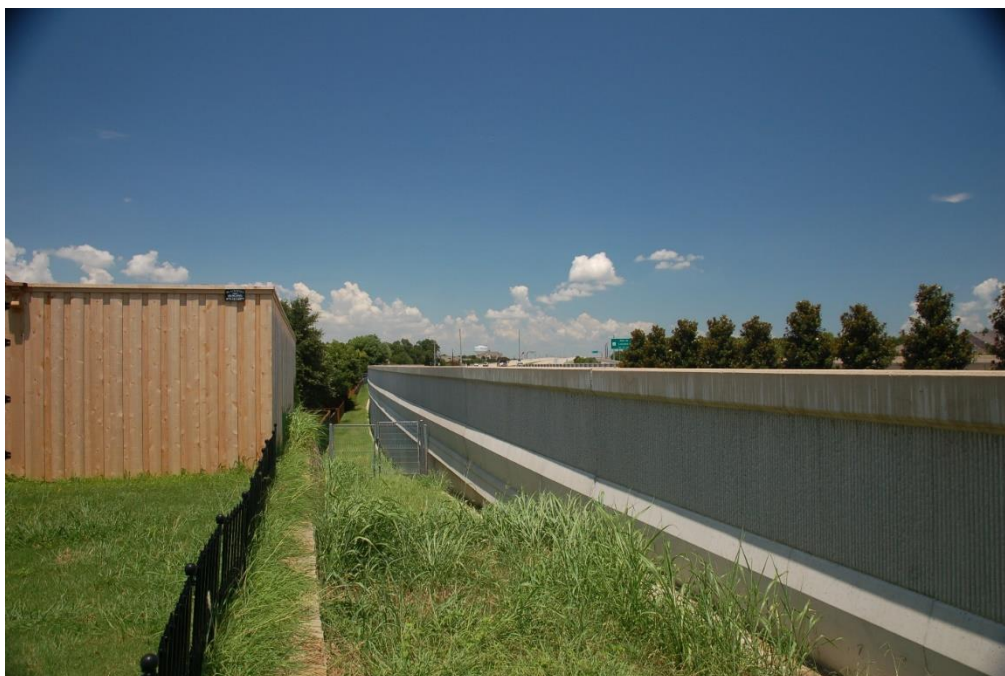
Figure 2.32 View of SH 190 and noise wall from Site #8: 4509 Meadowcove Drive
