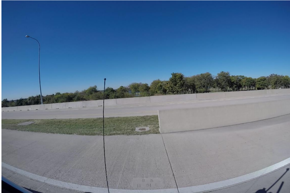
Figure 3.4 SH 190 Southbound main lane. Pavement cast on 9/10/2011 as indicated by inscription on the shoulder recorded by video
