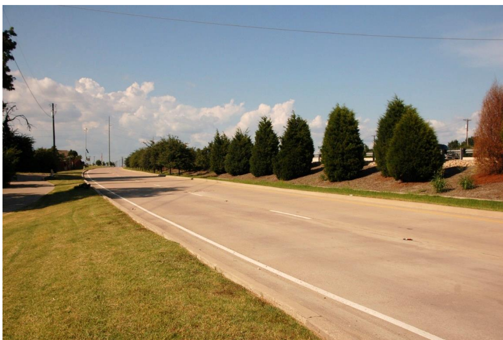
Figure 1.11 View of the southbound frontage road
