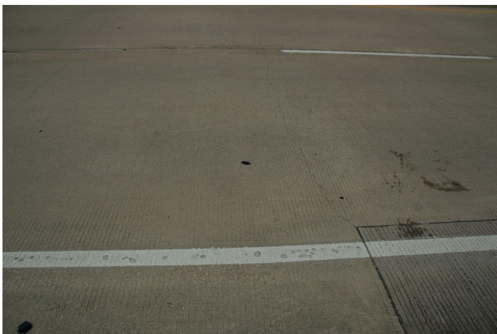
Figure 3.6 Northbound frontage road
