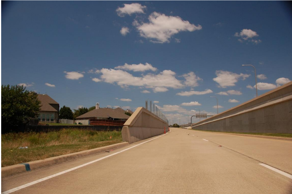
Figure 7.50 West side wall southernmost end
