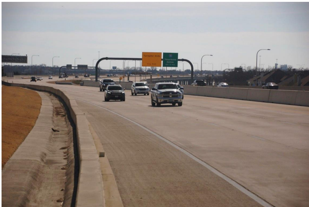
Figure 1.4 View of the northbound main lanes
