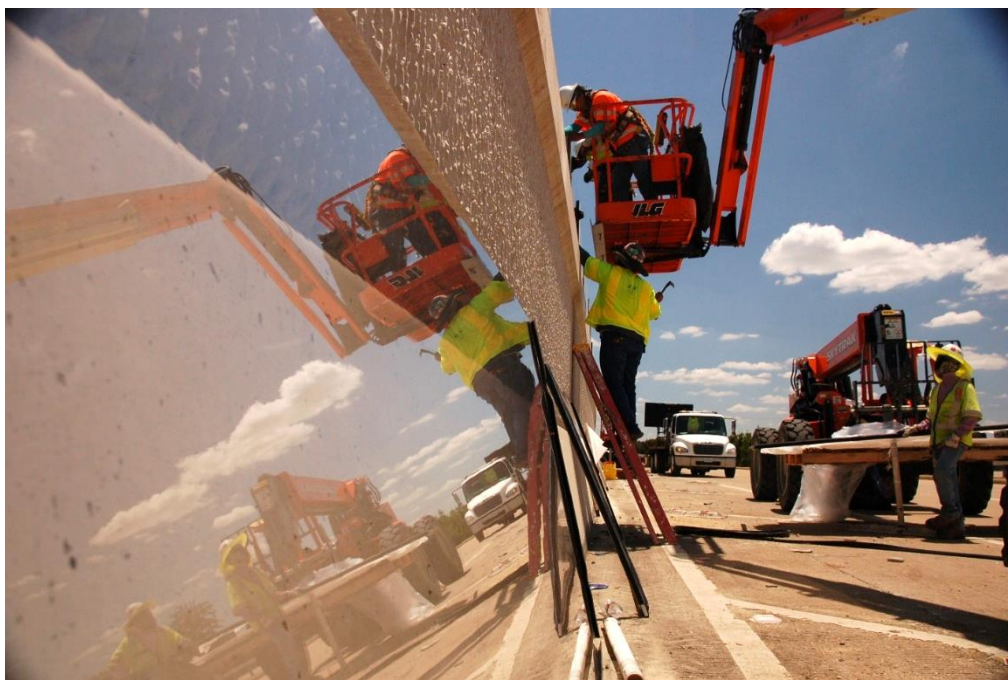
Figure 7.24 East side noise wall installation. Acrylic panel placement (July 24, 2019)
