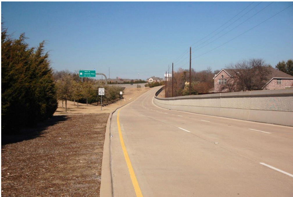
Figure 1.9 View of the northbound frontage road (transition from three to two lanes)
