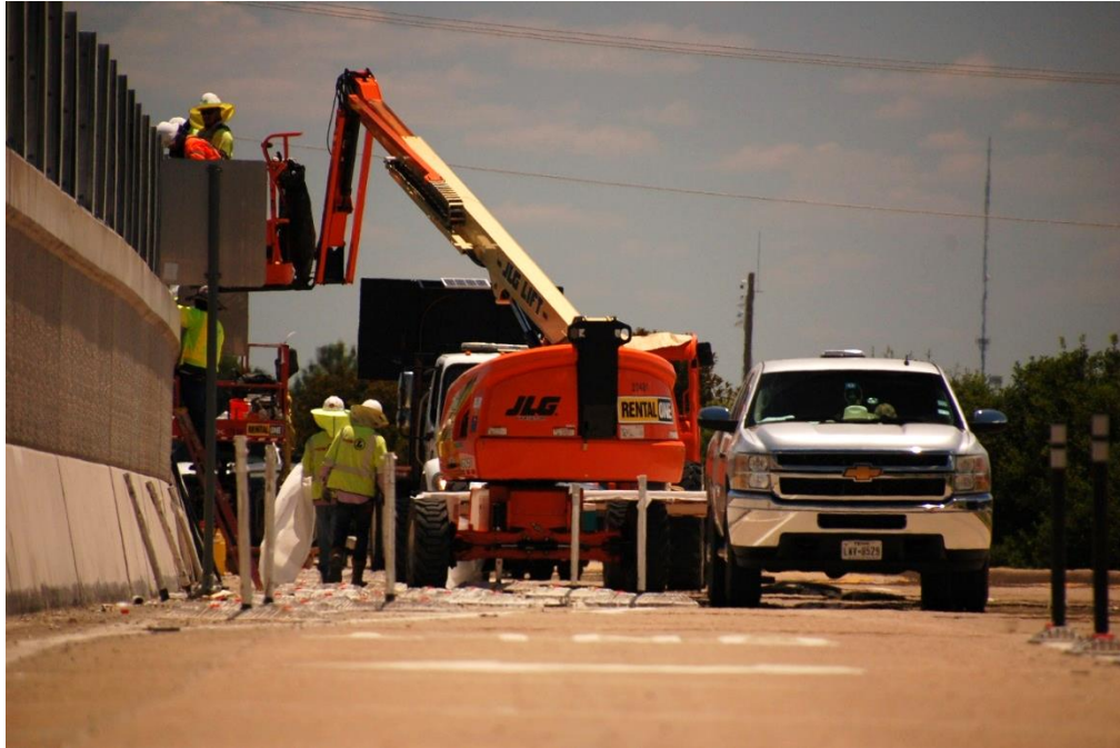
Figure 7.23 East side noise wall installation. Acrylic panel placement (July 24, 2019)
