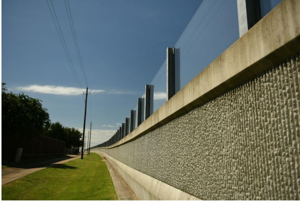
Figure 7.44 East side wall seen from neighborhood side
