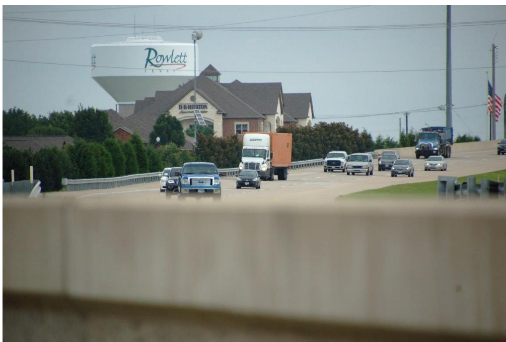
Figure 1.7 View of the southbound main lanes
