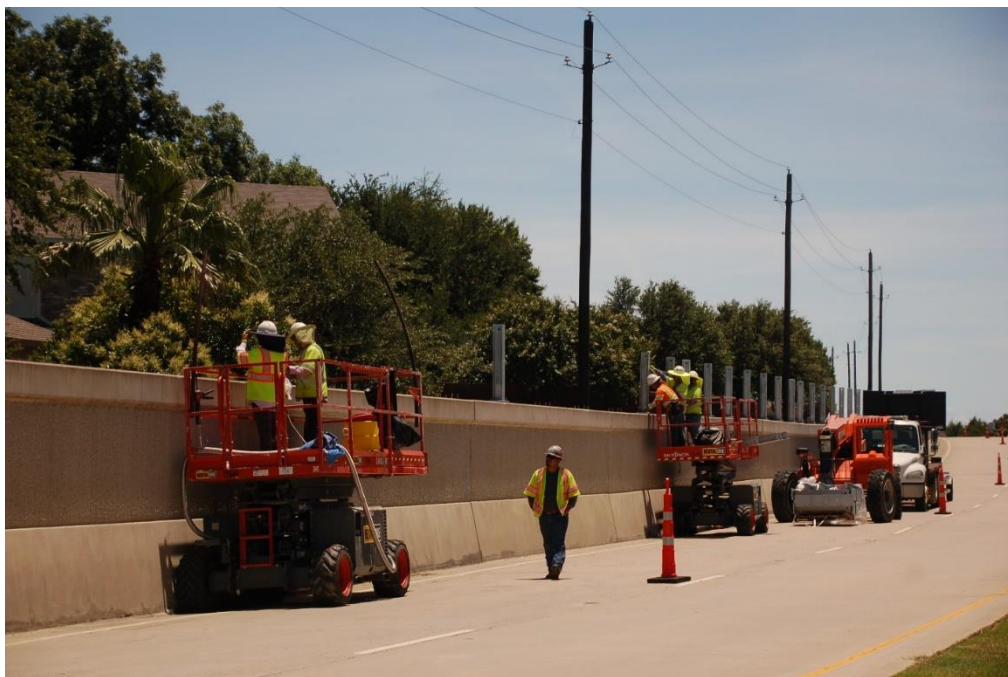
Figure 7.4 Noise wall installation on the east side (June 13, 2019)
