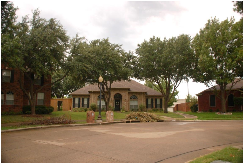
Figure 2.41 Front view of Site #4: 4902 Bayport Circle
