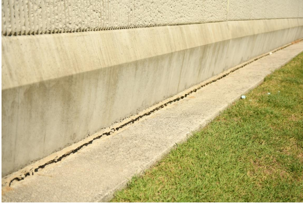
Figure 7.39 Separation between noise wall and concrete base, east side wall, close to receiver R#1
