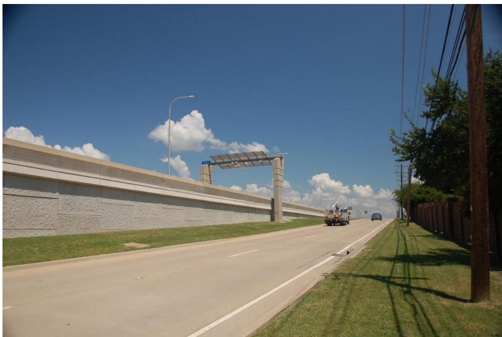
Figure 1.10 View of the northbound frontage road
