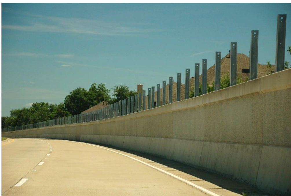
Figure 7.14 Noise wall installation progress on the west side (June 13, 2019)
