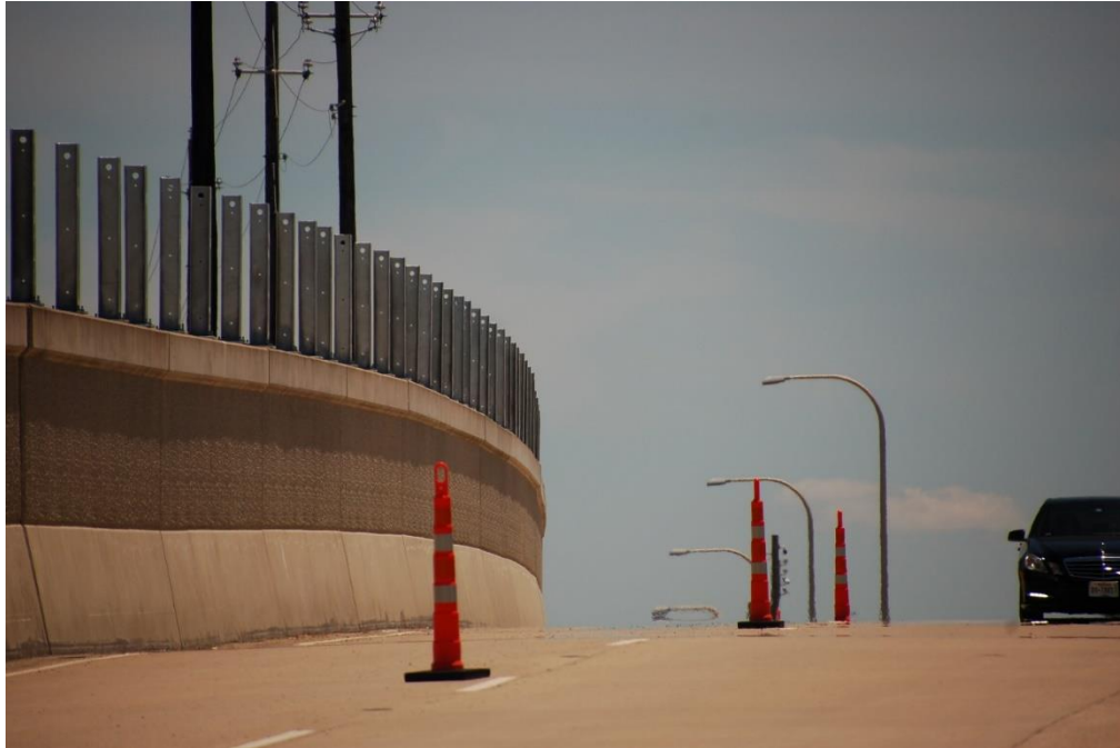
Figure 7.5 Noise wall installation on the east side (June 13, 2019)
