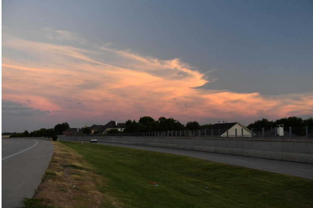
Figure 7.48 West side wall seen from main lanes
