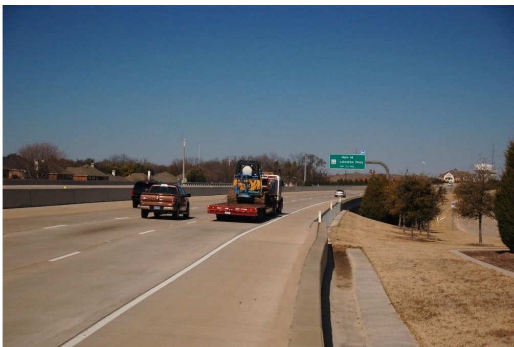
Figure 1.5 View of the northbound main lanes
