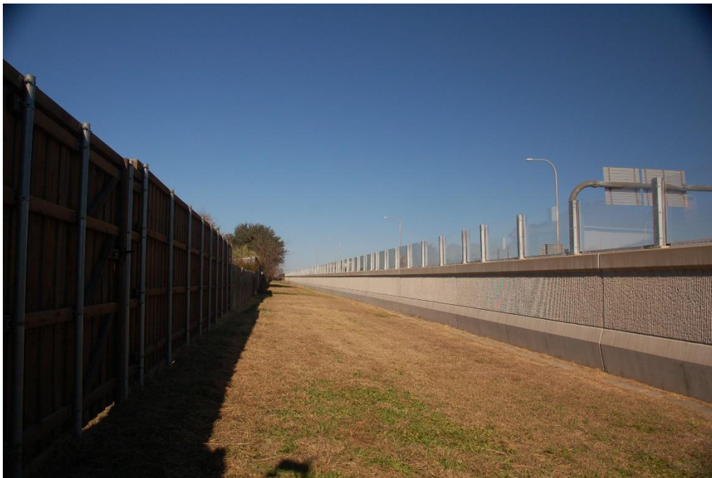
Figure 7.45 West side wall seen from neighborhood side
