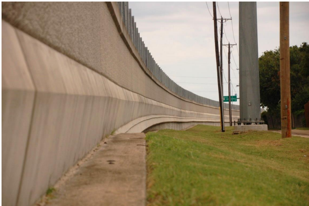
Figure 7.28 East side noise wall finalized, as seen from the neighborhood side (August 14, 2019)
