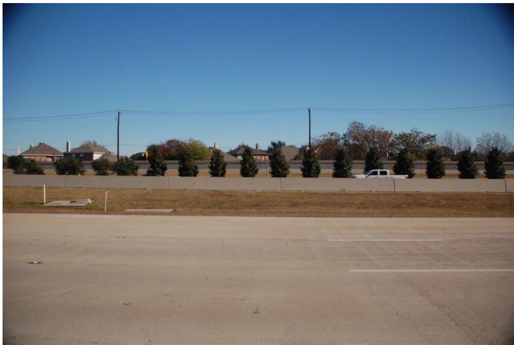
Figure 3.5 Southbound main lanes
