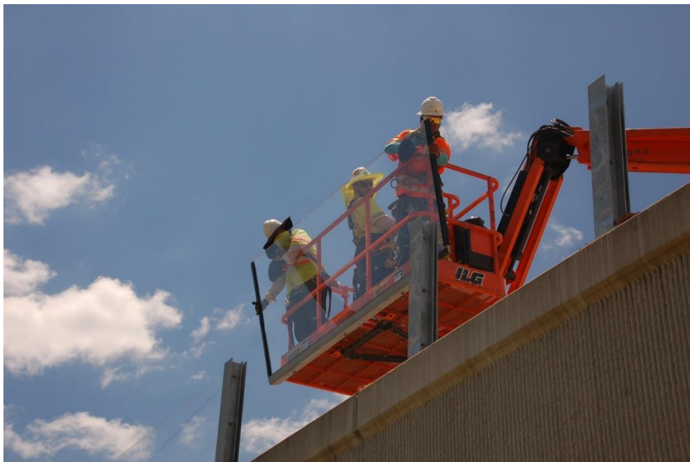
Figure 7.20 East side noise wall installation. Acrylic panel placement (July 24, 2019)
