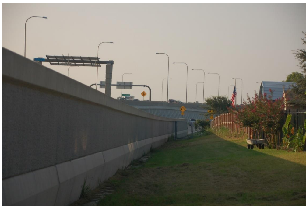
Figure 1.14 View of the west noise wall from the neighborhood side
