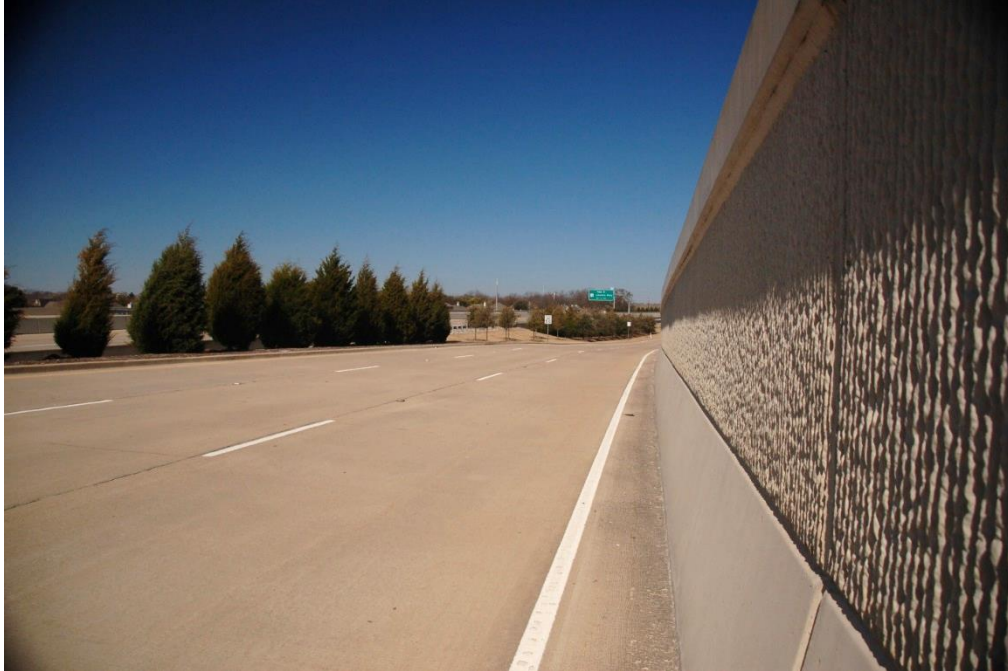
Figure 1.8 View of the northbound frontage road
