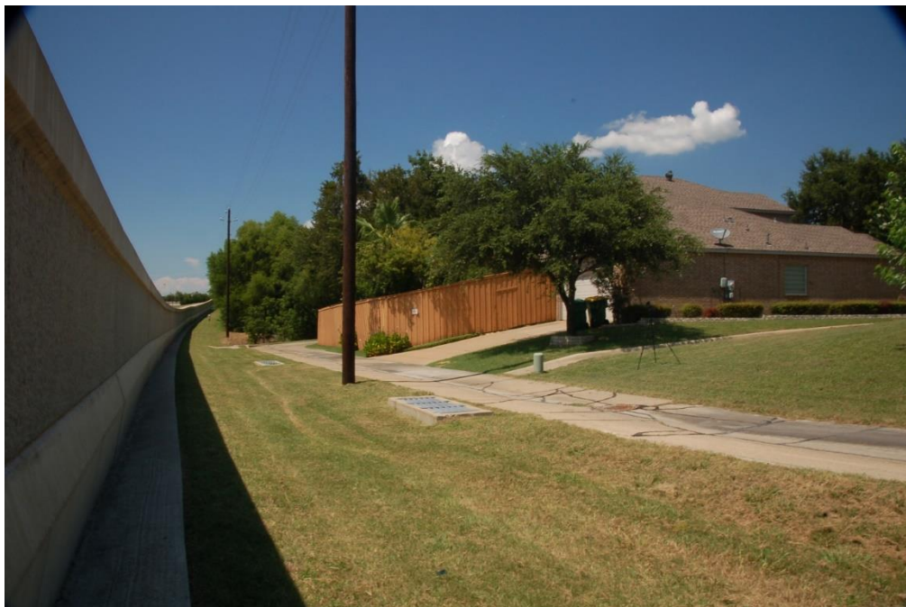
Figure 2.8 Noise measurement at Site #2: 2205 Mermaid Circle showing the back of the residence and existing noise wall
