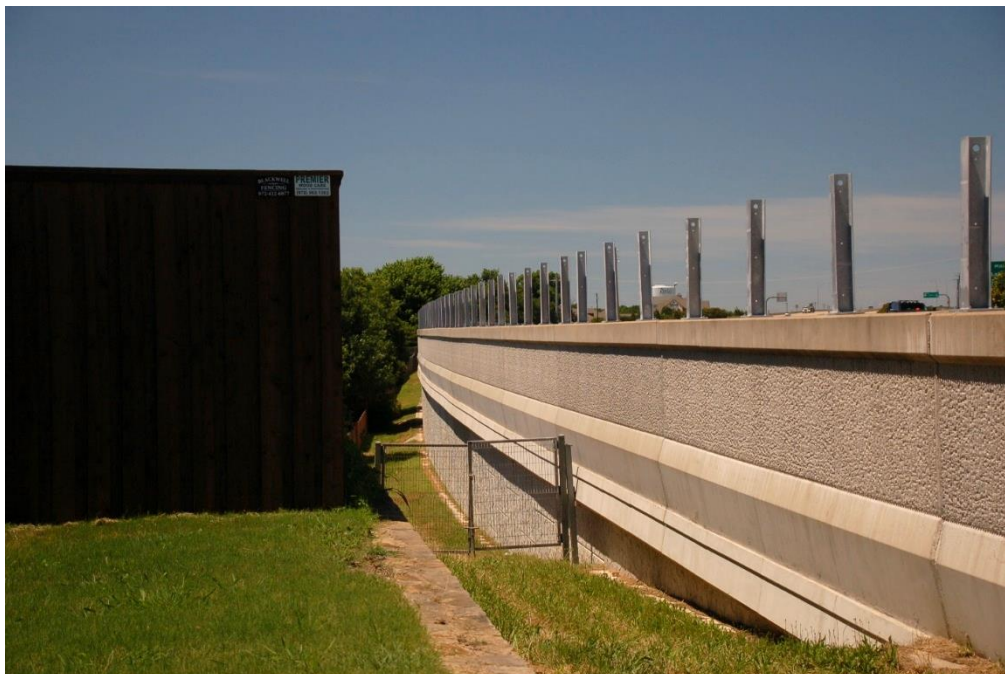
Figure 7.13 Noise wall installation progress on the west side (June 13, 2019)
