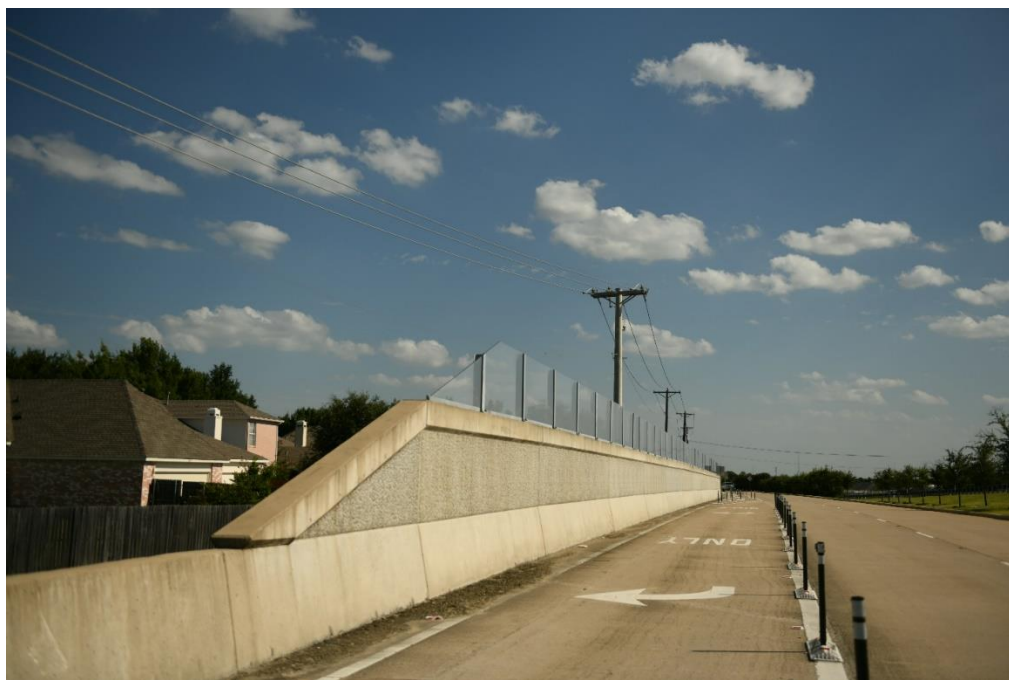
Figure 7.51 East side wall northernmost end
