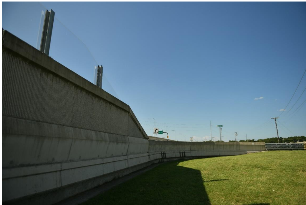
Figure 7.53 East side wall northernmost end
