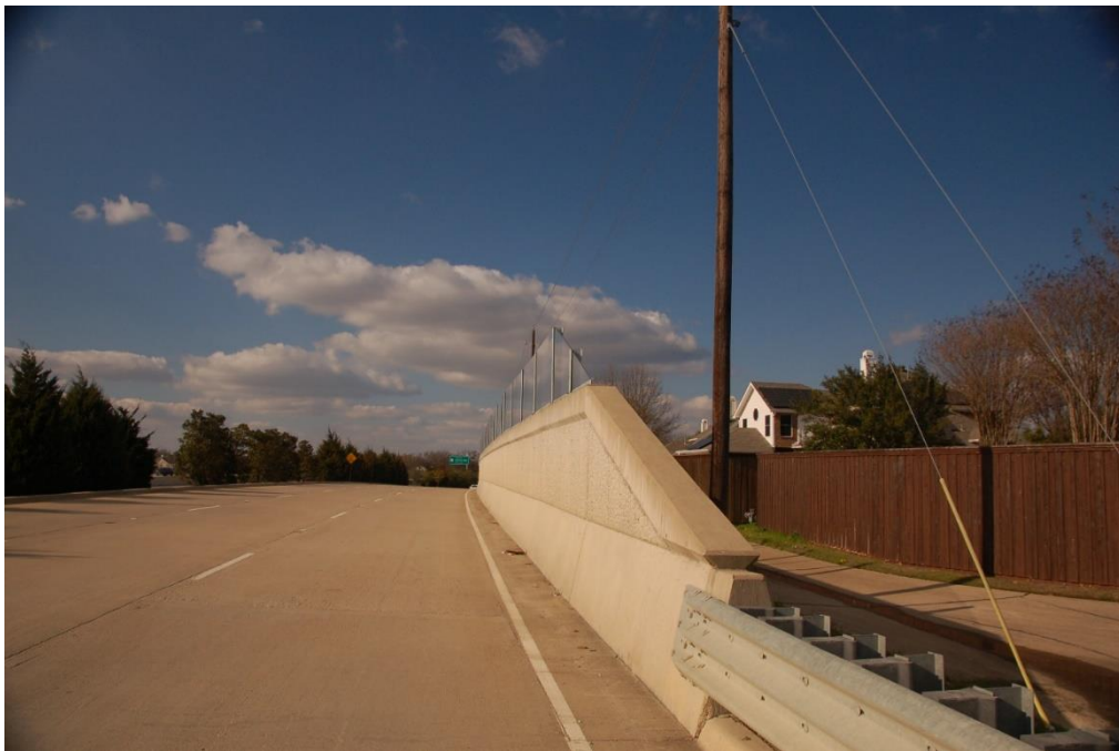
Figure 7.55 East side wall southernmost end
