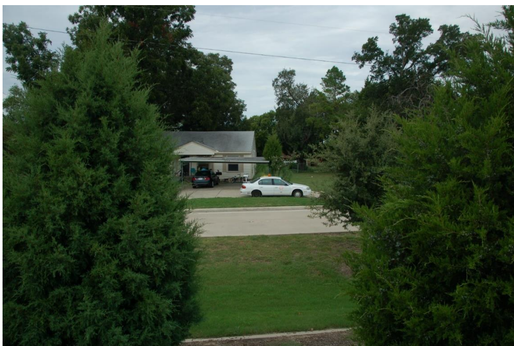
Figure 2.27 Front view of Site #7: 2629 Kirby Road, as seen from the main lanes of SH 190
