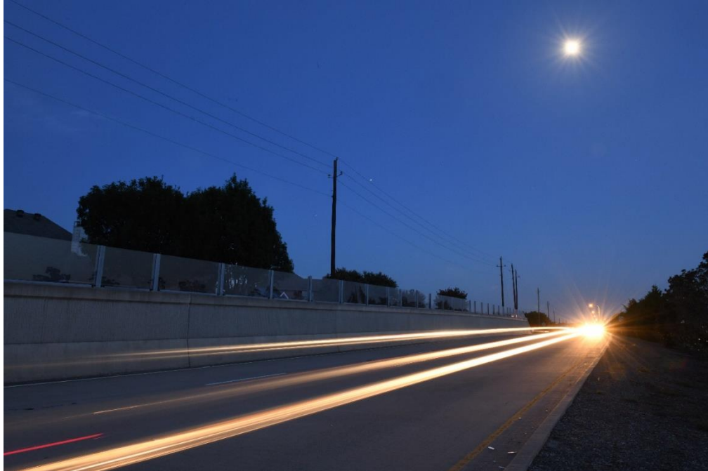
Figure 7.42 East side wall seen from northbound frontage road
