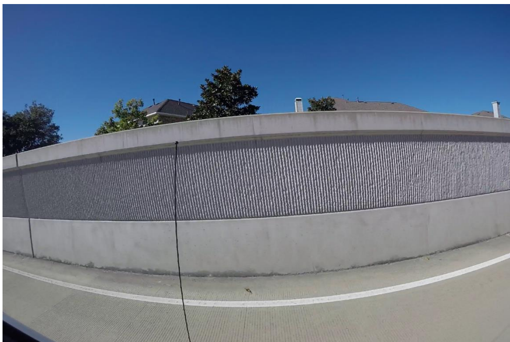
Figure 3.16 Southbound frontage road. Pavement in excellent condition as recorded by video
