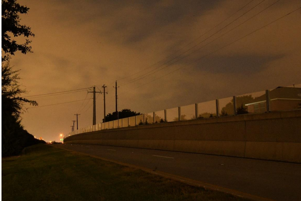
Figure 7.46 East side wall seen from northbound frontage road
