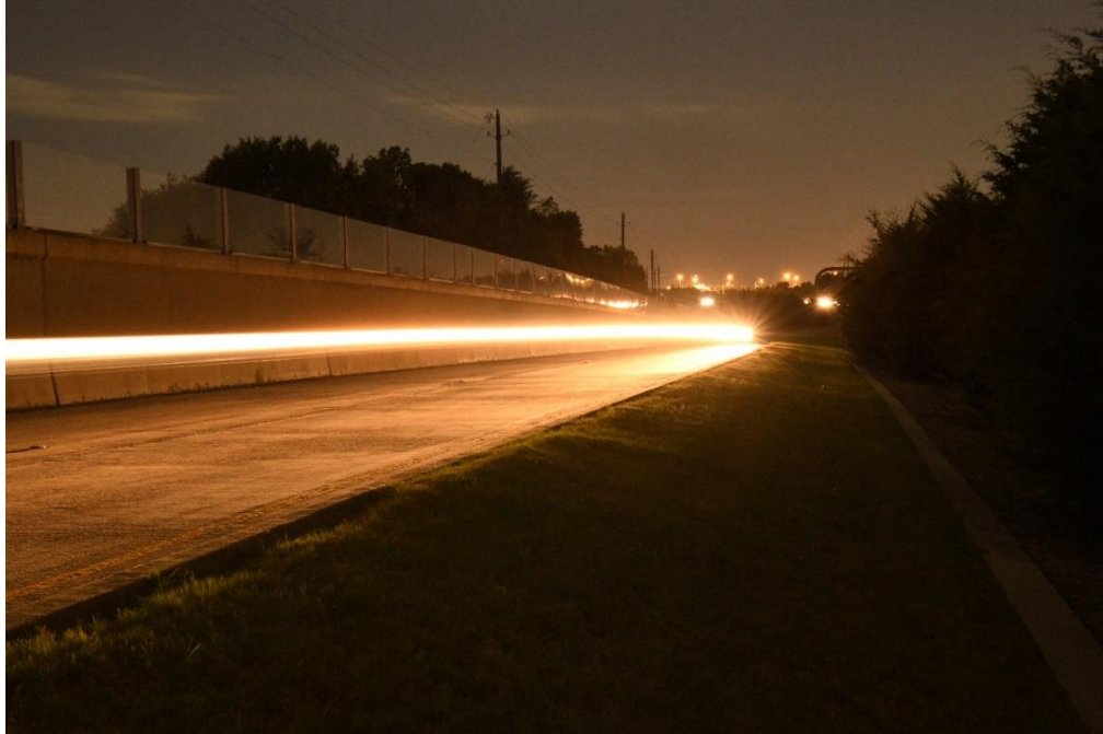
Figure 7.56 West side wall seen from southbound frontage road
