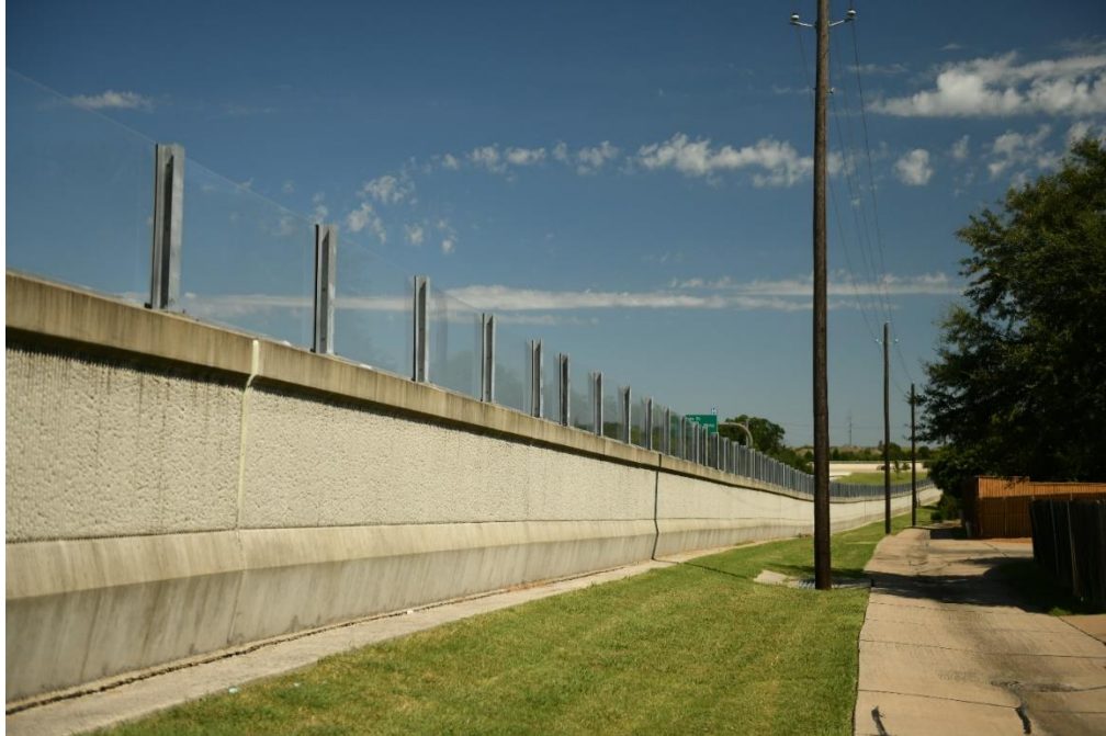
Figure 7.54 East side wall seen from neighborhood side
