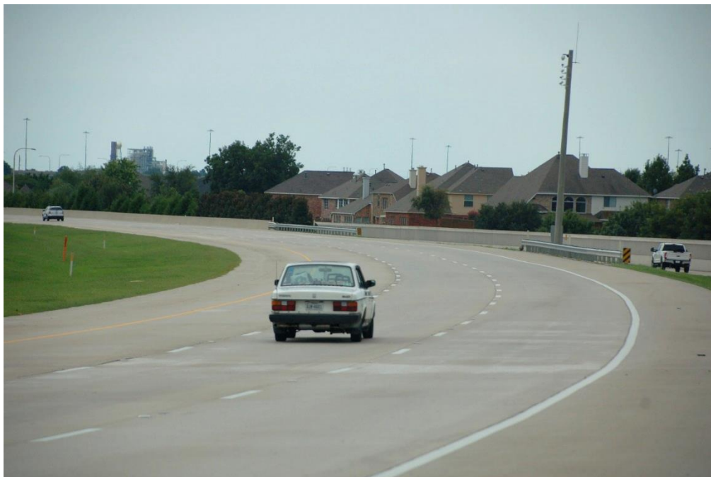
Figure 3.7 Southbound main lanes
