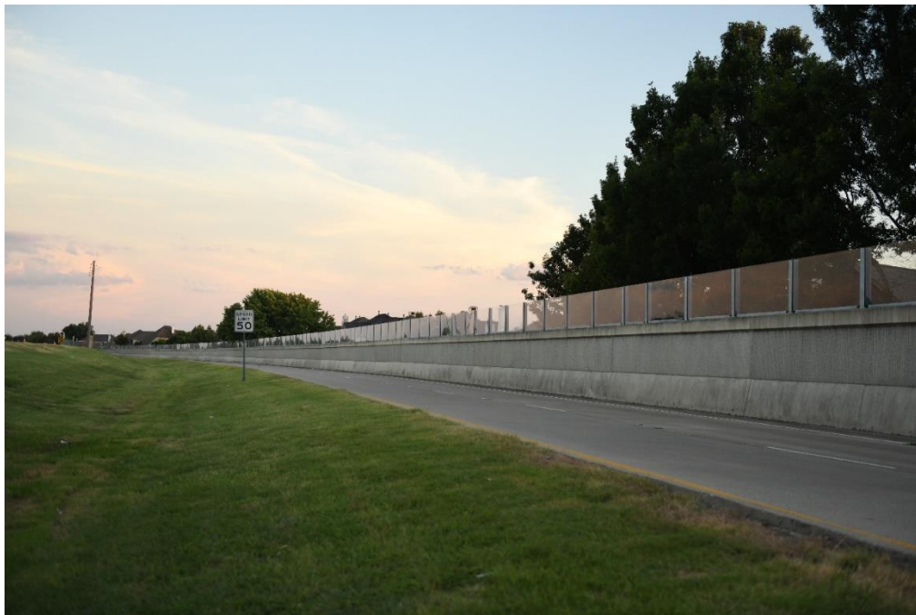
Figure 7.47 West side wall seen from southbound frontage road
