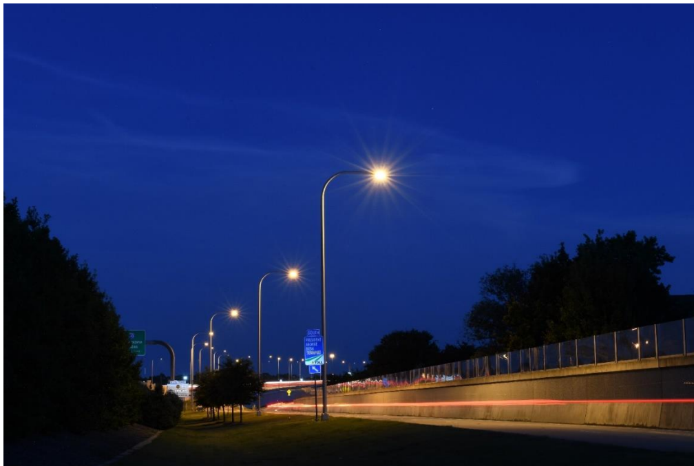
Figure 7.57 West side wall seen from main lanes
