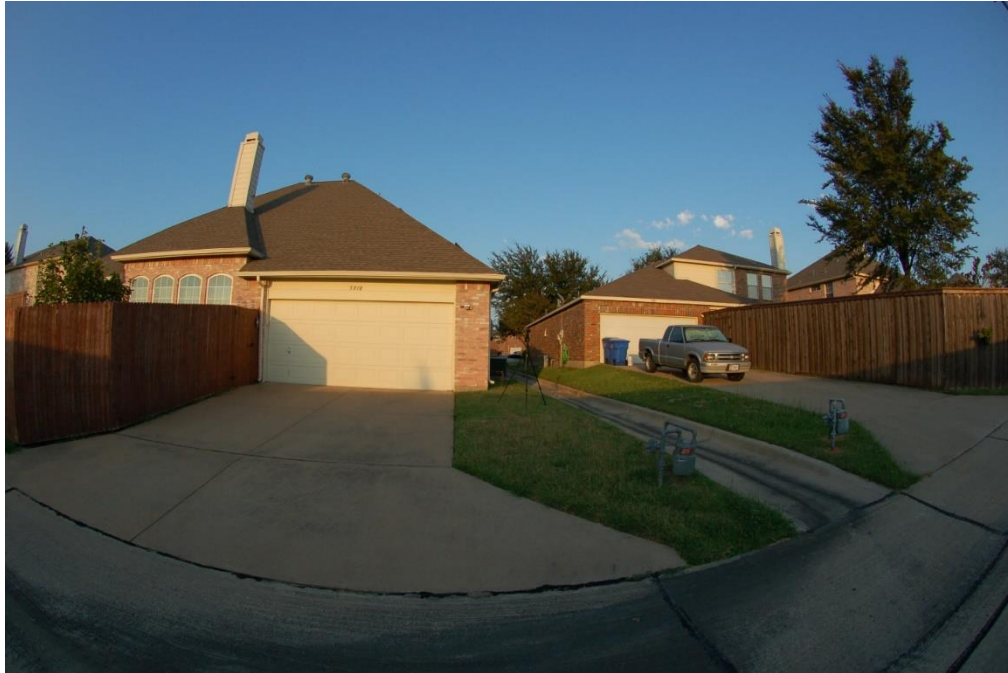
Figure 2.4 View of Site #1: 5010 Southport Drive from the back.
