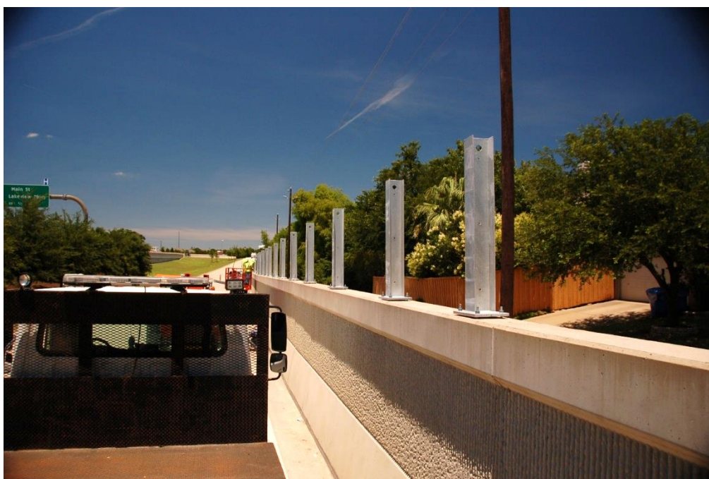
Figure 7.8 Noise wall installation on the east side (June 13, 2019)
