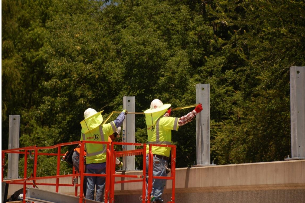
Figure 7.9 Noise wall installation on the east side (June 13, 2019)
