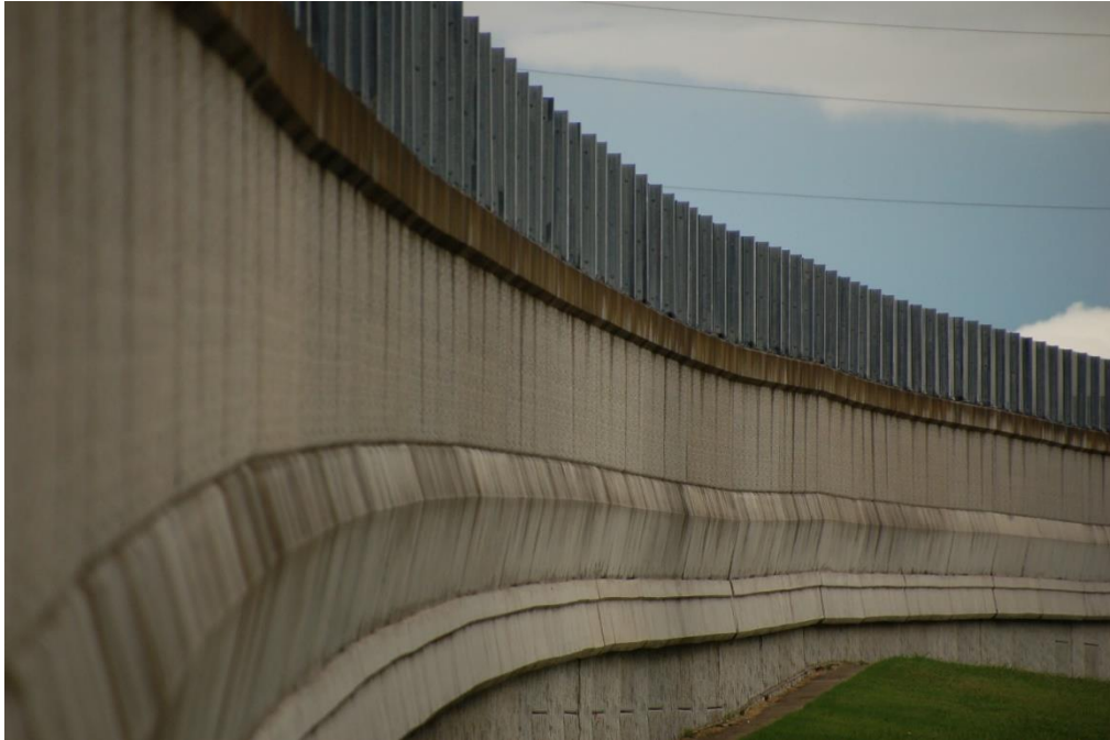
Figure 7.52 East side wall seen from neighborhood side
