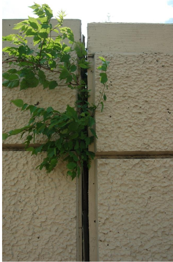
Figure 8.40 Vegetation from the creek side growing through the openings in the concrete structure
