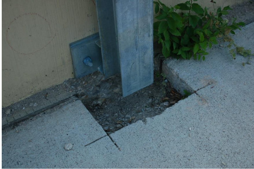
Figure 9.30 Small foundations to anchor vertical posts sawing existing concrete for Segment 3 (May 2018)
