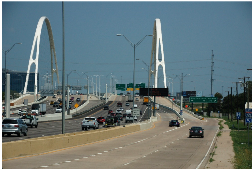
Figure 9.45 Asphalt overlay on main lanes (L), CRCP on frontage road (R) (April 2018)
