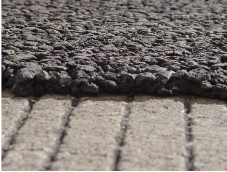
Figure 3.21 1-in.-thick 2010 PFC overlay on I-30 on top of CRCP (2010)
