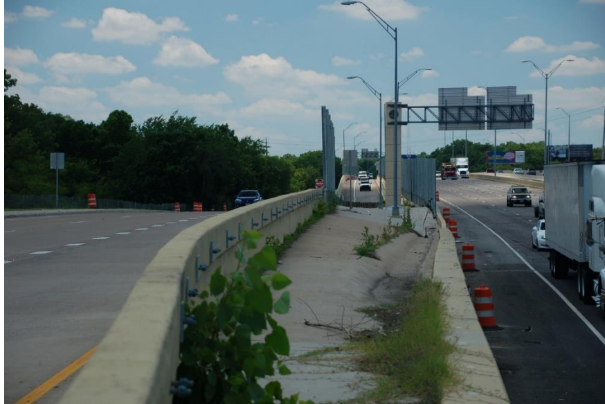
Figure 9.10 Frontage road and main lanes CTBs converge in a wedge-like shape (May 2018)
