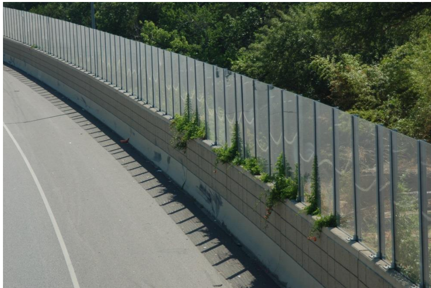
Figure 8.35 Vegetation from the creek side growing through the openings in the gaskets under noise barrier
