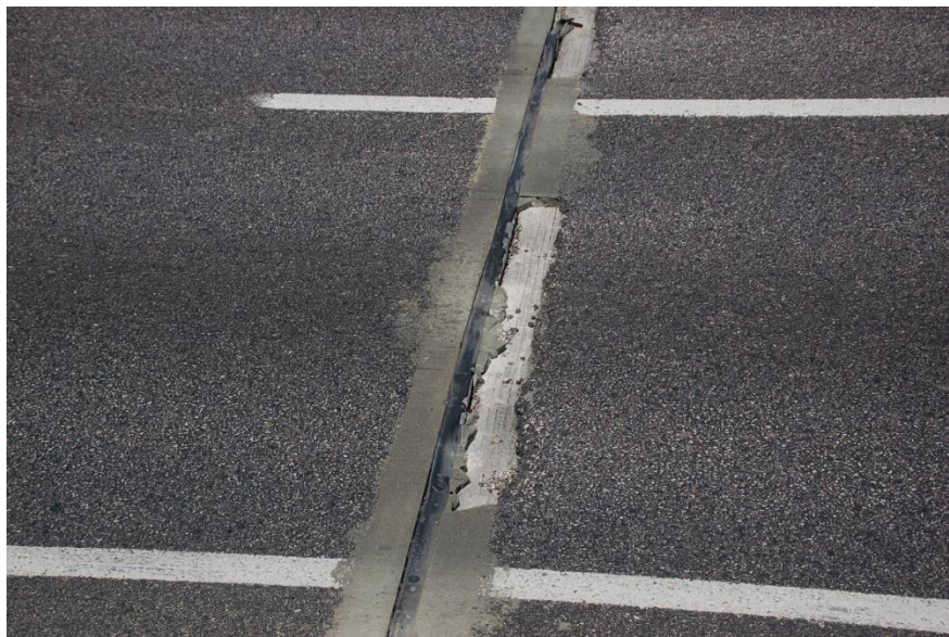
Figure 9.41 Open, damaged expansion joint in the pavement, eastbound outside lane (April 2018)
