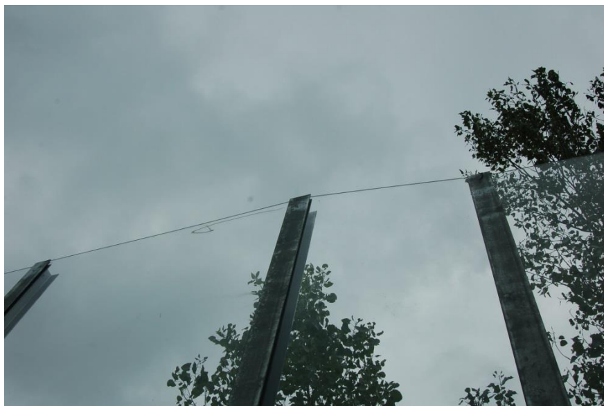
Figure 8.10 Vertical support off-plumb
