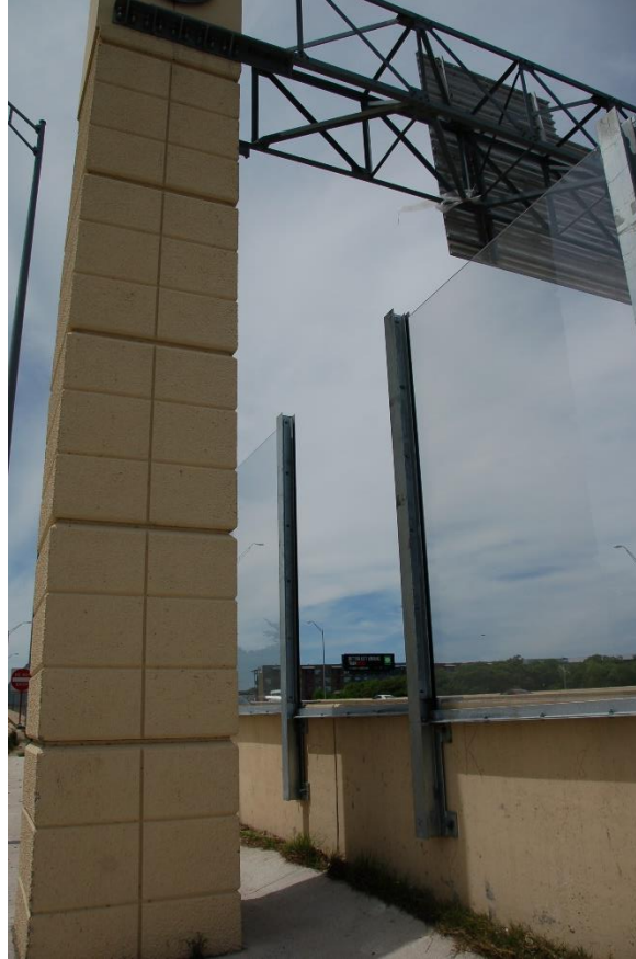
Figure 9.26 Missing panel under cantilever highway sign seen from behind the wall
