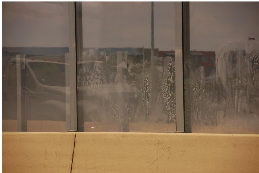
Figure 9.57 Panel showing permanent damage after cleaning (August 15, 2019)
