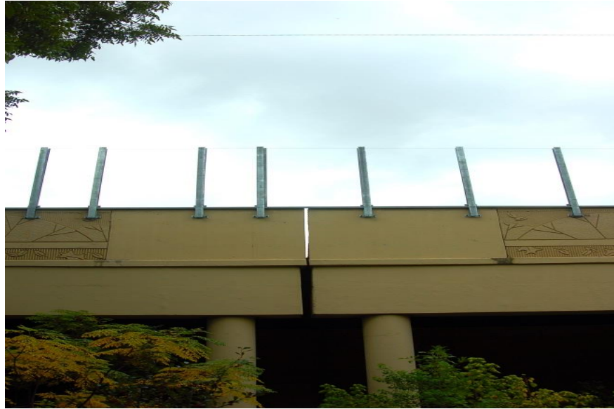
Figure 8.15 Gap in existing concrete wall at bridge expansion joint as seen from Coombs Creek
