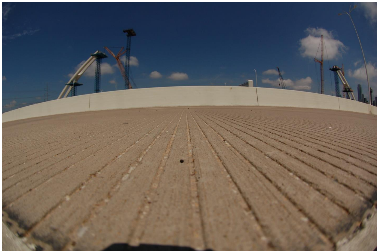
Figure 9.2 CRCP on the deck of the new McDermott Bridge
