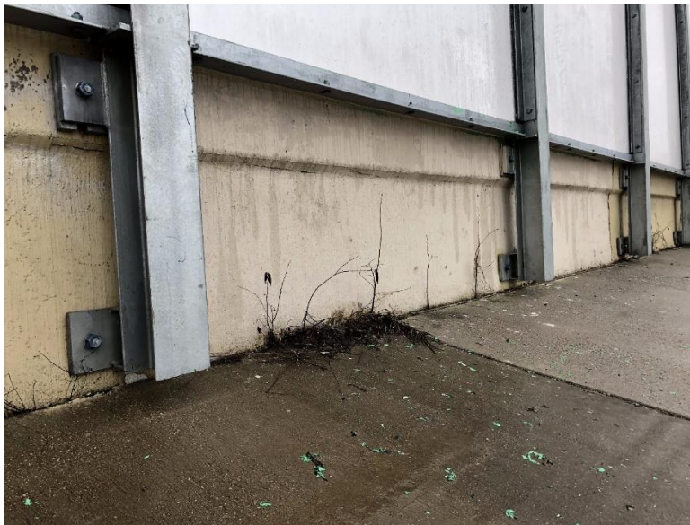
Figure 9.53 Painted CTB to cover graffiti and remnants of graffiti on the ground (February 19, 2019)
