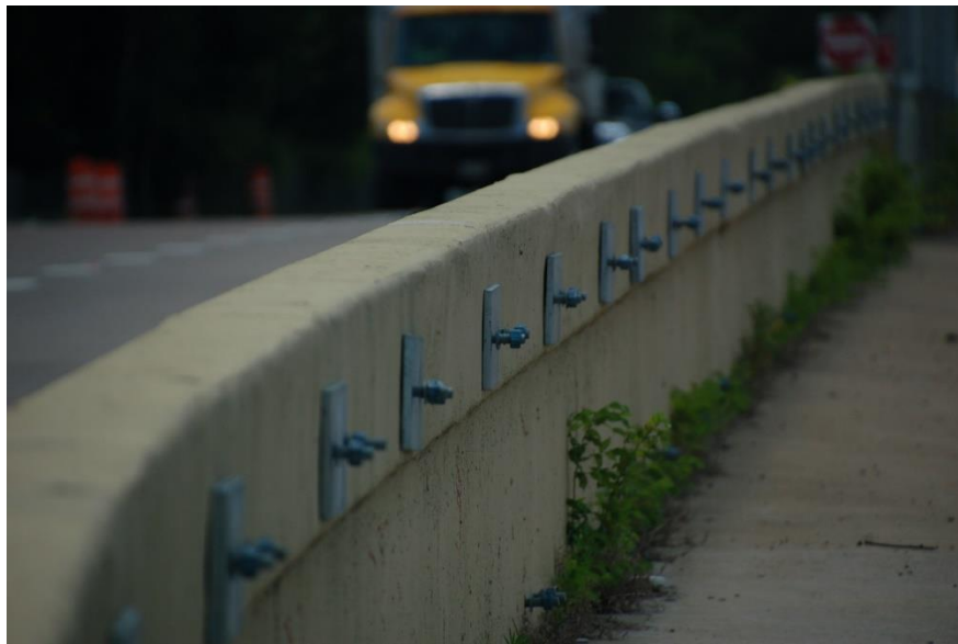
Figure 9.20 Only plates and bolts remained after some posts were removed in April to fix design problem (May 2018)
