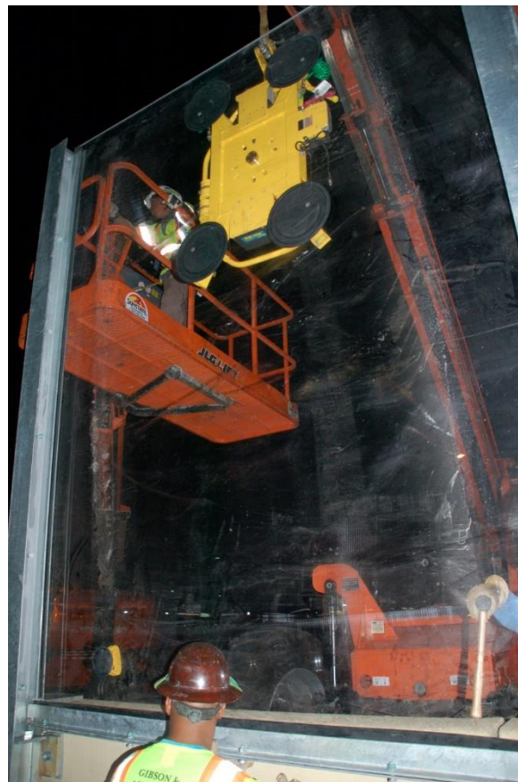
Figure 9.39 Acrylic panel installation
