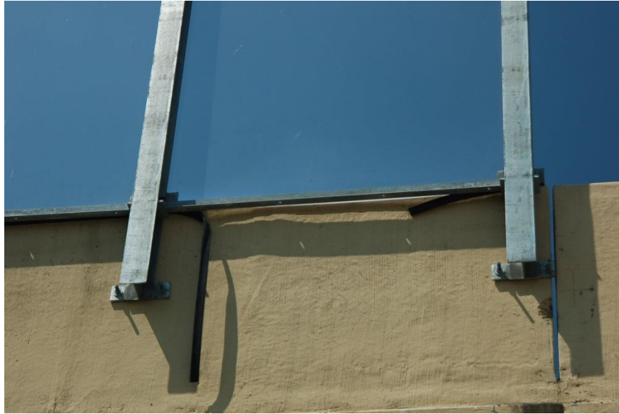
Figure 8.32 Broken horizontal rubber gasket
