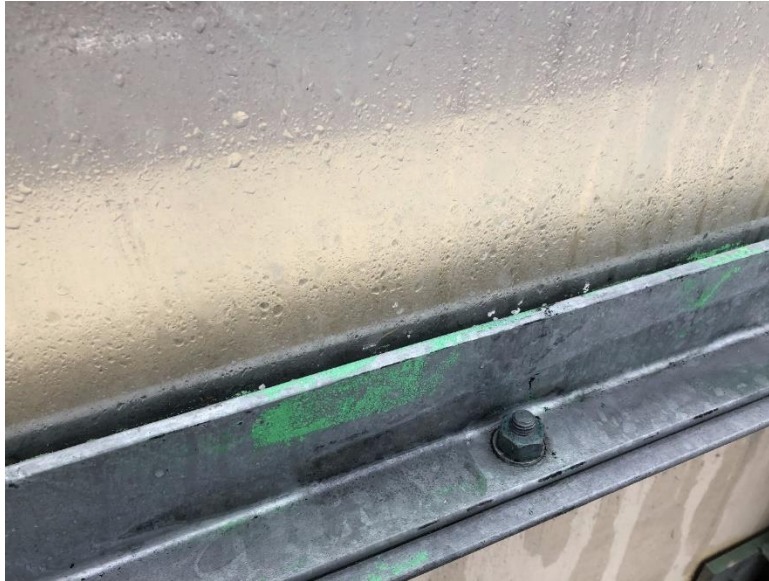
Figure 9.54 Paint remaining on metal support after graffiti removal (February 19, 2019)
