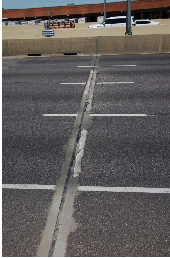
Figure 9.42 Open, damaged expansion joint in the pavement, main lanes (April 2018)
