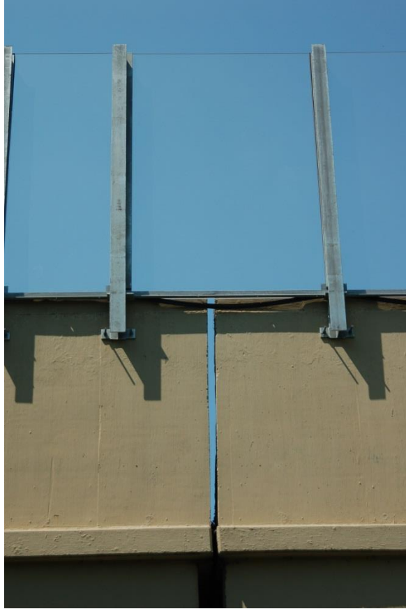
Figure 8.37 Expansion joint opening due to lack of sealant
