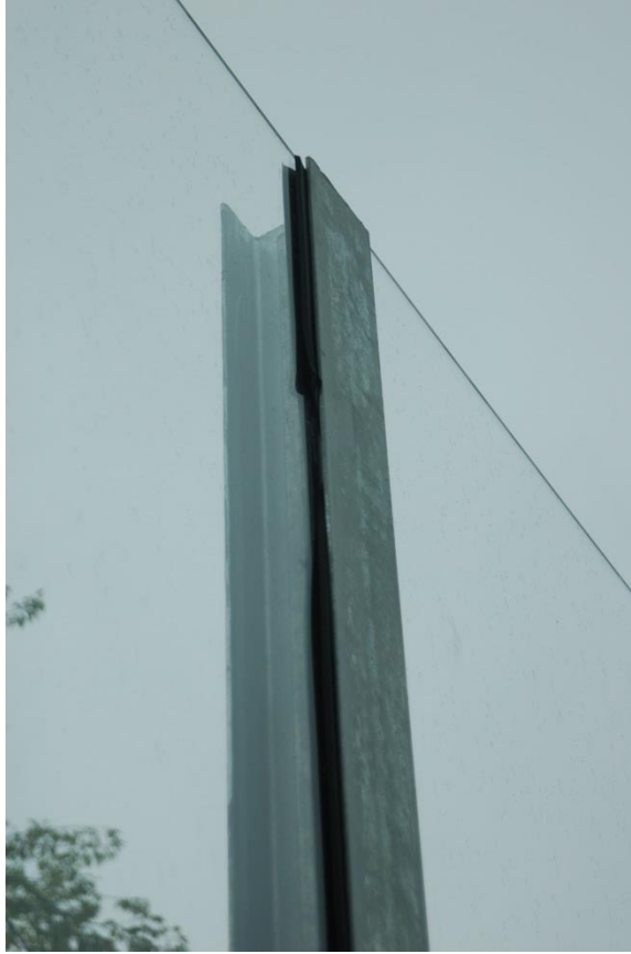
Figure 8.11 Gasket protruding from metal support
