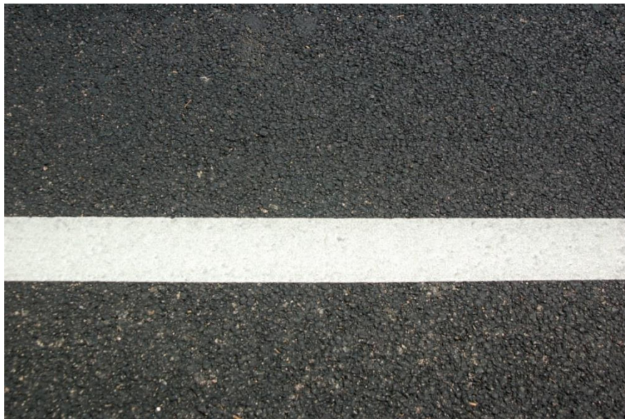
Figure 3.30 2010 PFC shortly after it was placed
