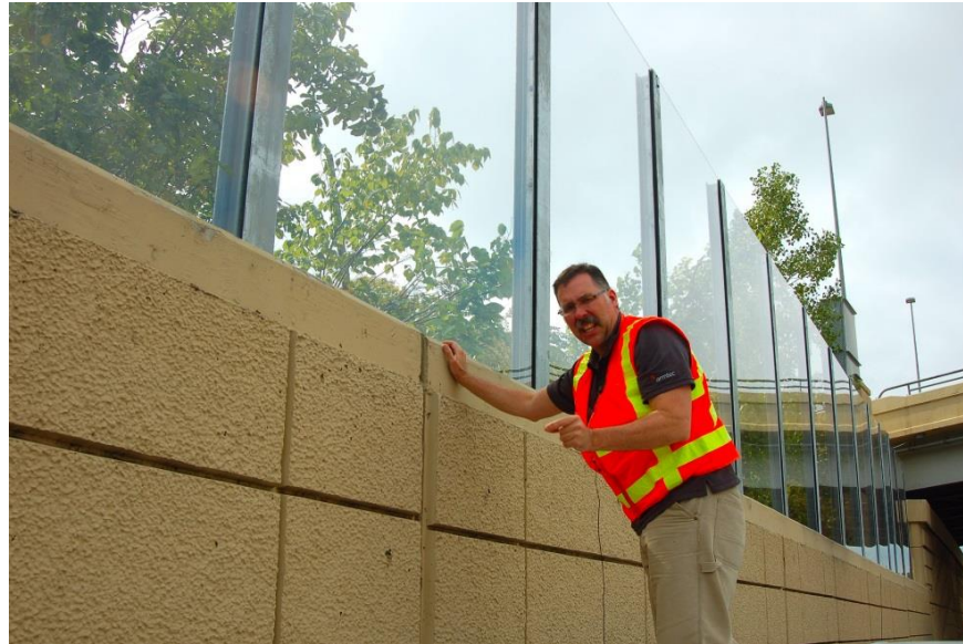
Figure 8.14 Armtec's Mark McIlheran inspecting the wall, showing the gap size between a panel and the gasket
