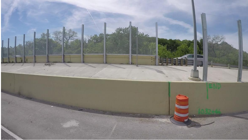
Figure 9.23 No overlap between Segment 2 and Segment 3, seen from the main lanes (April 2018)
