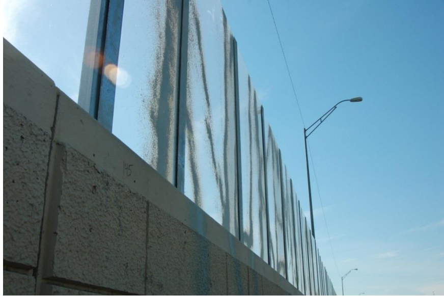
Figure 8.19 Graffiti as seen from the highway shoulder on November 11, 2013. The damage extends to the concrete wall under span #144.
