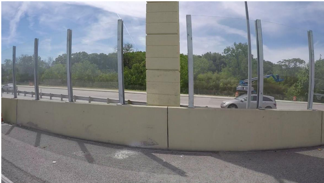
Figure 9.27 Missing panel under cantilever highway sign seen from the main lanes
