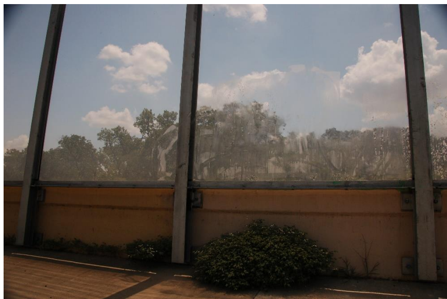
Figure 9.58 Three panels showing permanent damage after cleaning (August 15, 2019)
