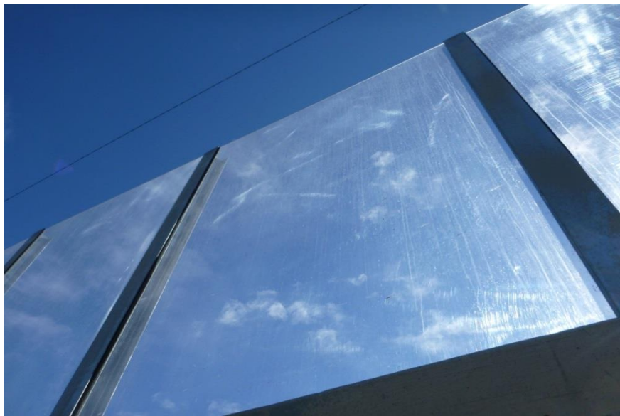
Figure 8.25 Cleaned panel showing traces of the cleaning operation
