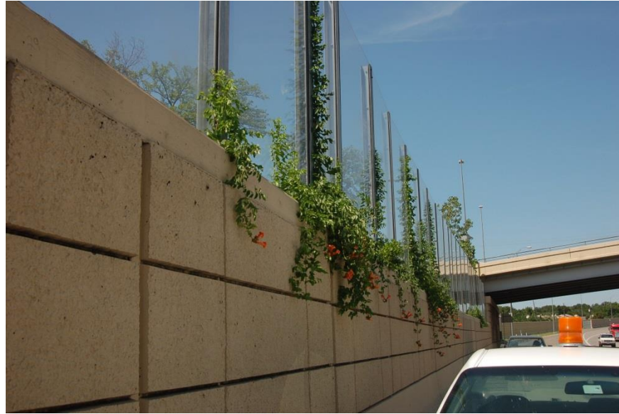
Figure 8.36 Vegetation from the creek side growing through the openings in the gaskets under noise barrier
