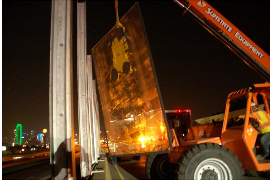
Figure 9.38 Hoisting acrylic panel
