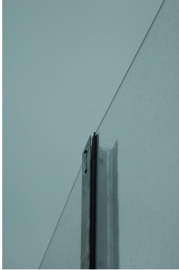
Figure 8.12 Gap between vertical gasket and metal support
