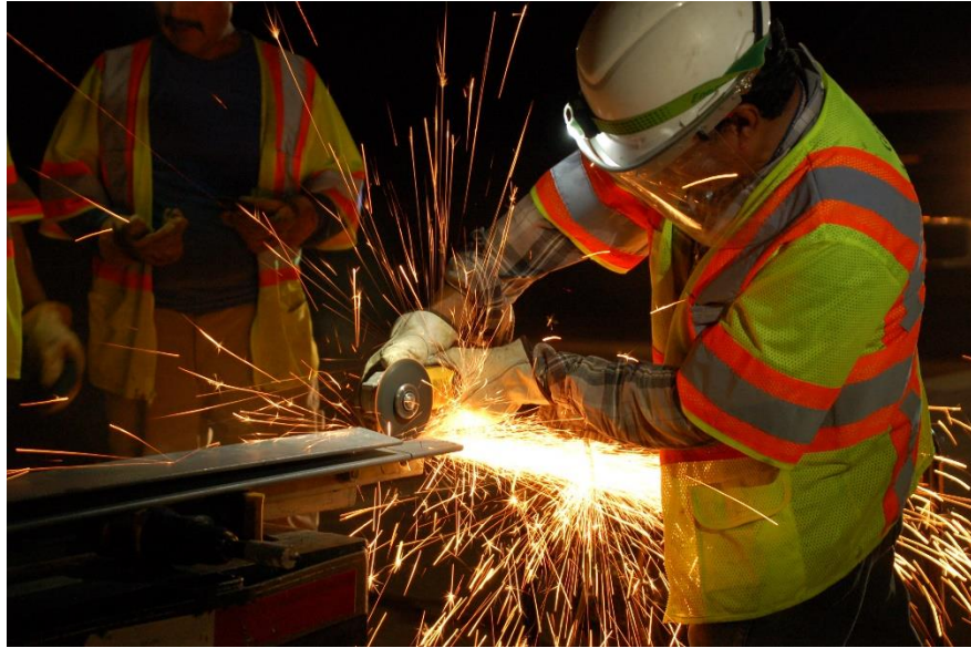
Figure 9.32 On-site cutting of metal post
