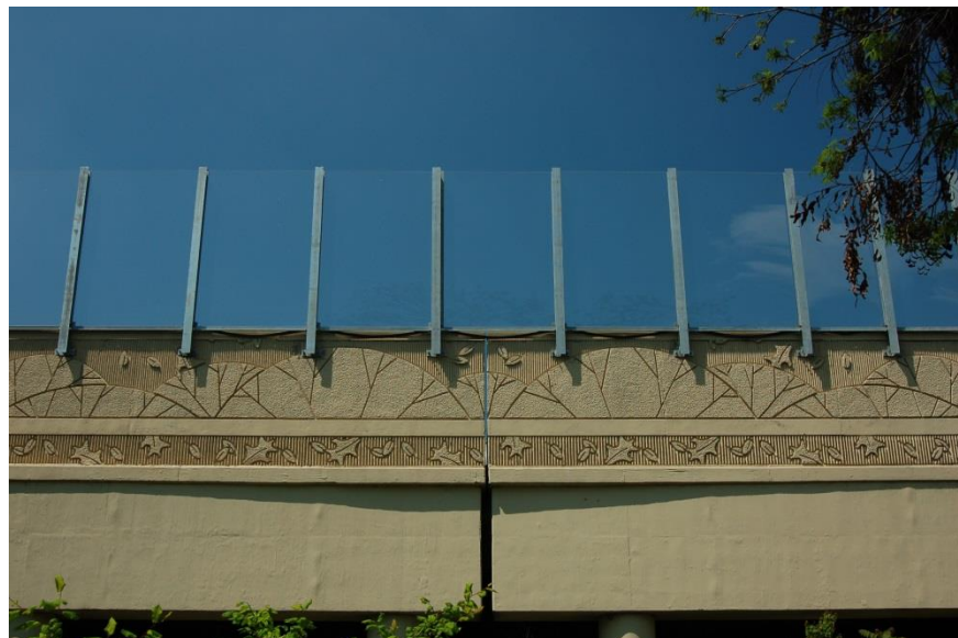
Figure 8.29 Sagging of horizontal rubber gaskets
