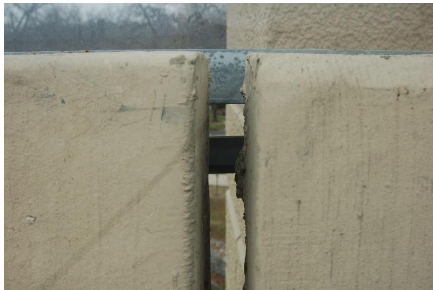
Figure 8.16 Gap in existing concrete wall at bridge expansion joint as seen from the highway side
