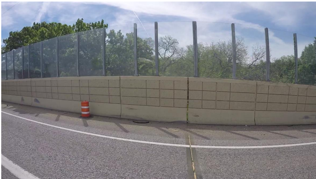
Figure 8.39 Open joint seen from the eastbound main lanes
