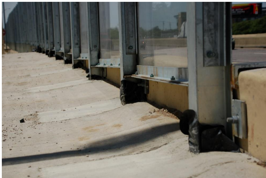
Figure 9.29 Small foundations to anchor vertical posts in Segment 2 (April 2018)
