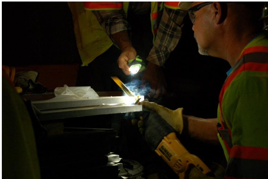
Figure 9.33 On-site cutting of acrylic panel
