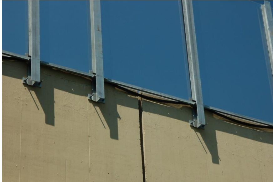
Figure 8.30 Sagging of horizontal rubber gaskets
