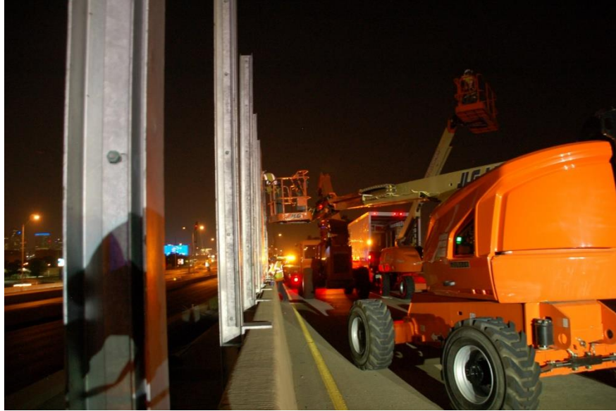
Figure 9.40 Finalizing panel installation from the bucket truck
