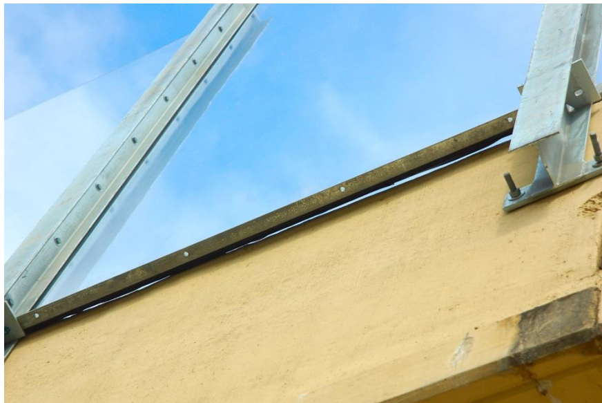
Figure 8.13 Gap between horizontal gasket and metal support
