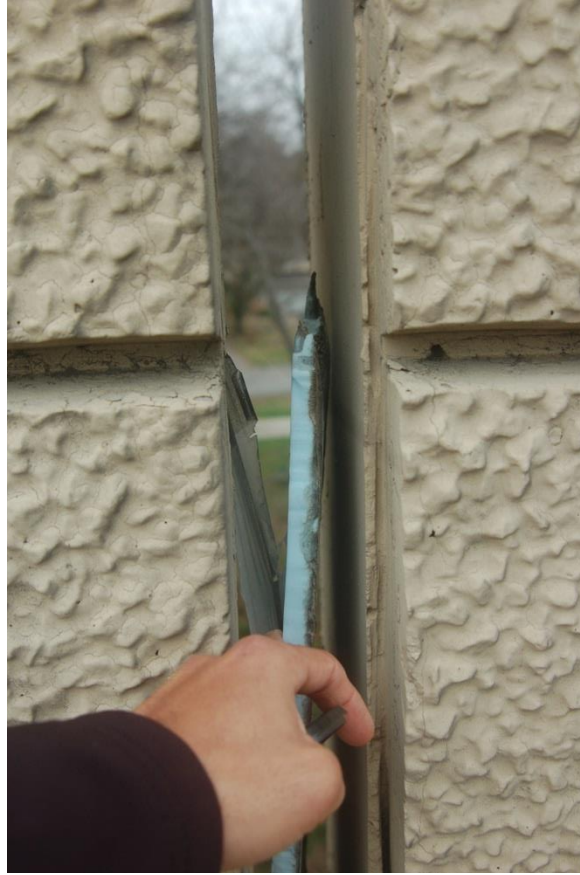
Figure 8.38 Damaged, old sealant material in the expansion joints of bridge structure
