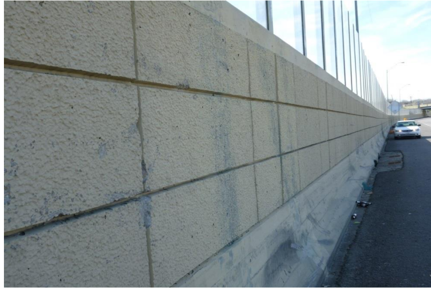
Figure 8.26 Remnants of the graffiti on the concrete wall below the panels
