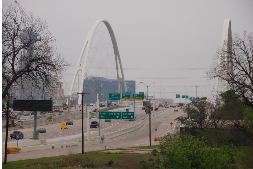
Figure 9.44 CRCP on both the main lanes and frontage road (March 2017)
