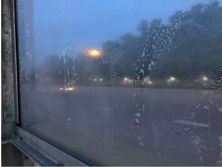
Figure 9.56 Panel showing permanent damage after cleaning (June 13, 2019)
