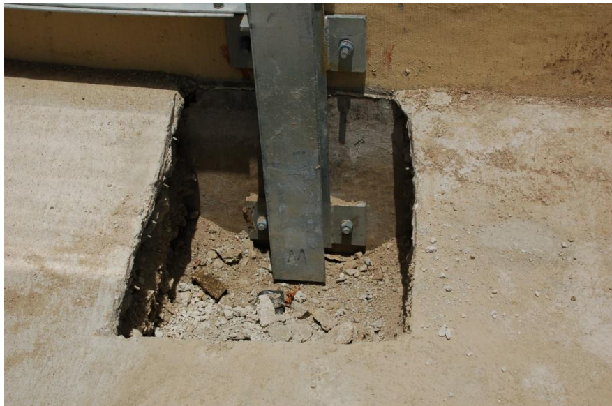
Figure 9.31 Small foundation under construction for Segment 2, sawing existing slab (July 2018)
