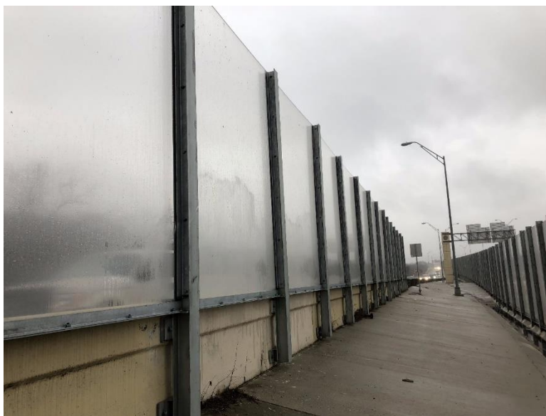
Figure 9.51 Graffiti cleaned from acrylic panels and CTB painted to cover graffiti (February 19, 2019)
