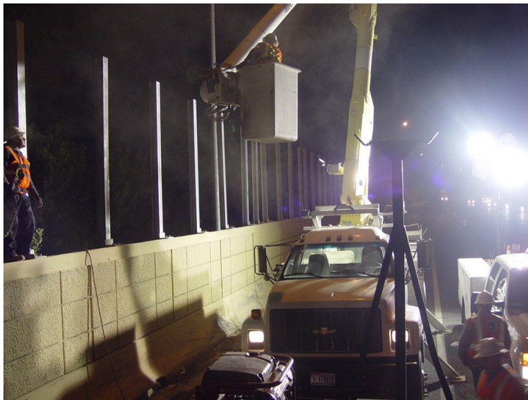
Figure 8.2 Vertical support placement
