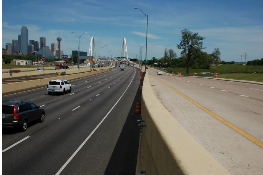
Figure 9.46 Asphalt overlay on main lanes (L), CRCP on frontage road (R) (April 2018)
