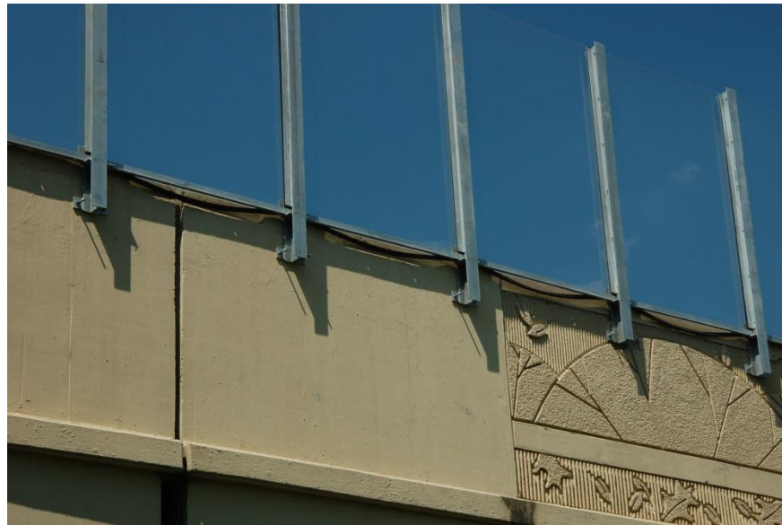
Figure 8.28 Sagging of horizontal rubber gaskets
