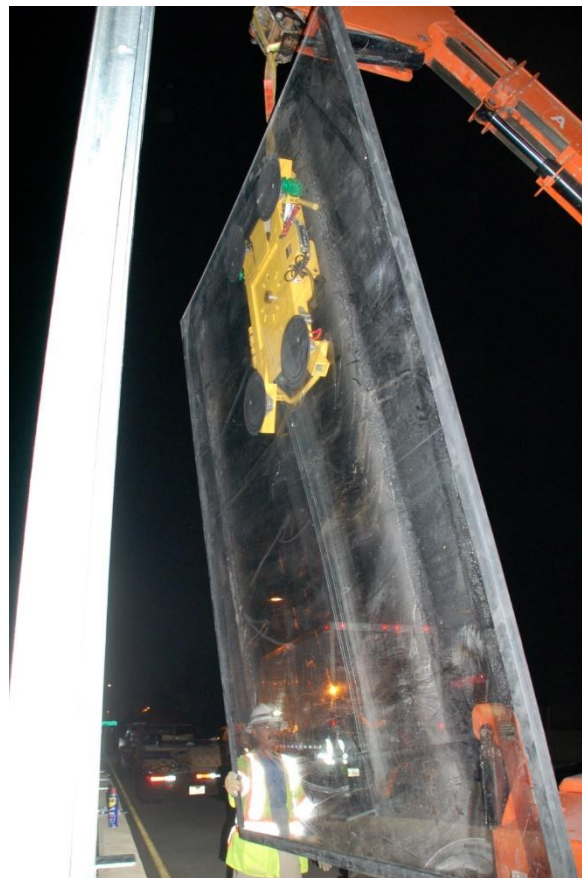
Figure 9.37 Hoisting acrylic panel
