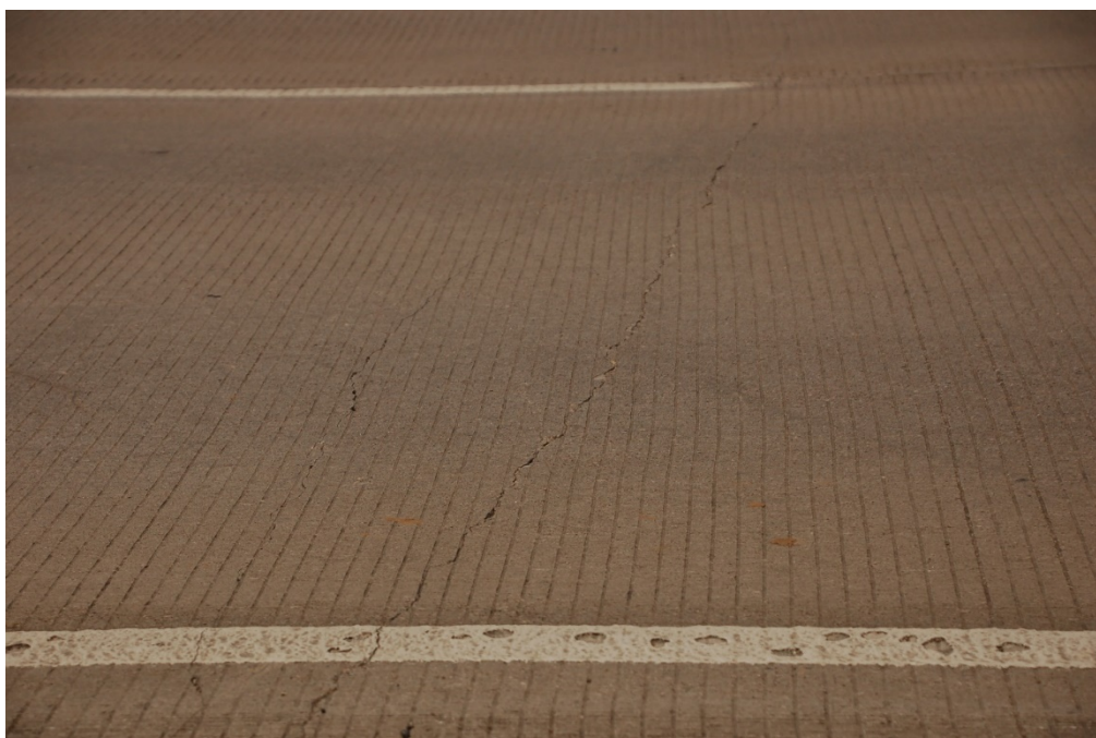
Figure 3.11: Northbound frontage road. Transverse cracks
