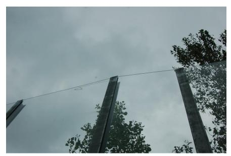
Figure 8.10: Vertical support off-plumb
