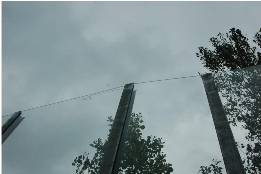
*Figure 8.10: Vertical support off-plumb*
