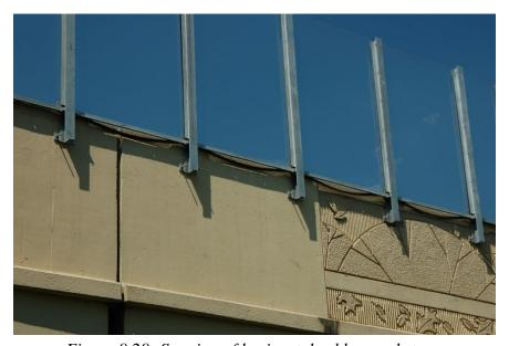
Figure 8.28: Sagging of horizontal rubber gaskets
