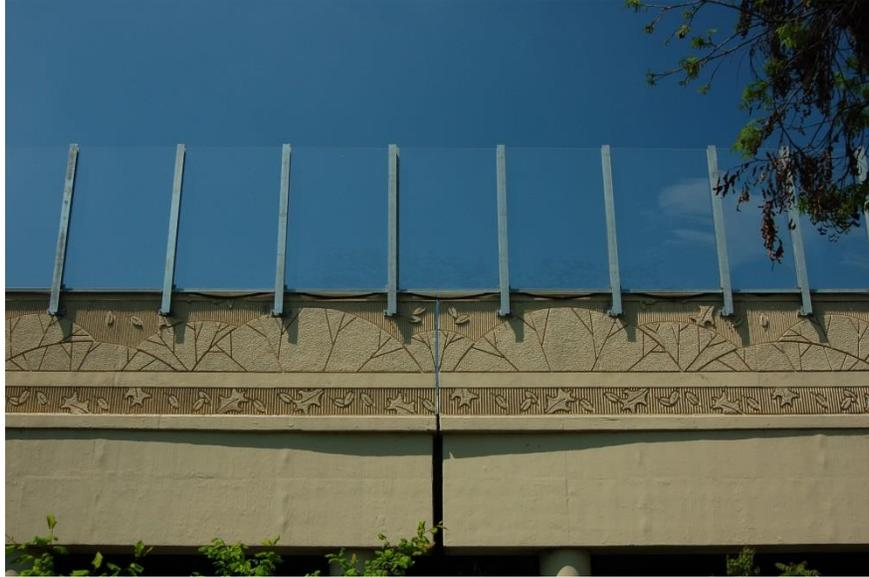
*Figure 8.29: Sagging of horizontal rubber gaskets*
