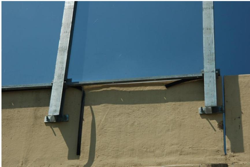
*Figure 8.32: Broken horizontal rubber gasket*
