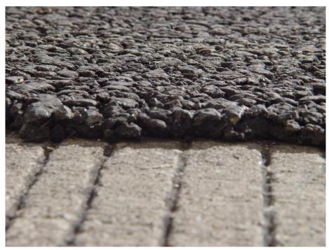
Figure 3.20: 1-in. thick 2010 PFC overlay on IH-30 on top of CRCP (2010)
