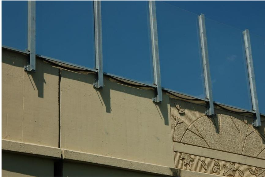
*Figure 8.28: Sagging of horizontal rubber gaskets*
