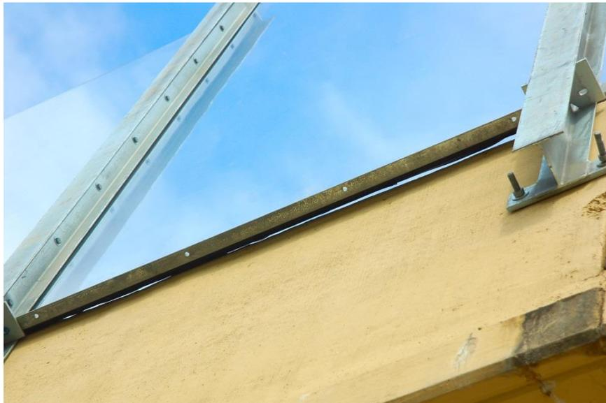
*Figure 8.13: Gap between horizontal gasket and metal support*
