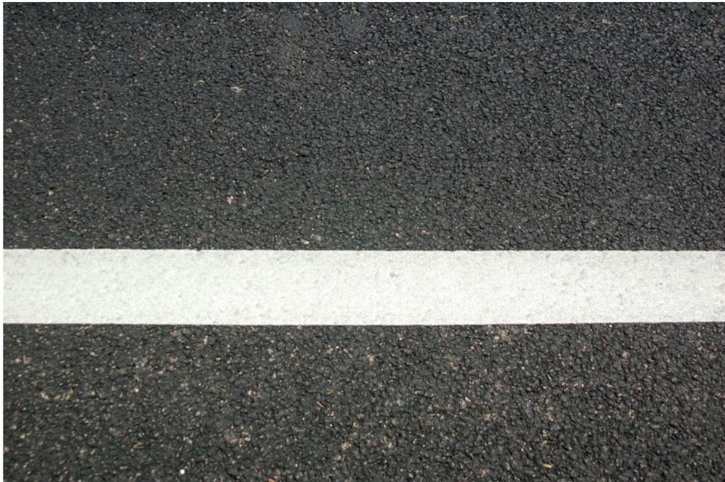
*Figure 3.25: 2010 PFC shortly after it was placed*
