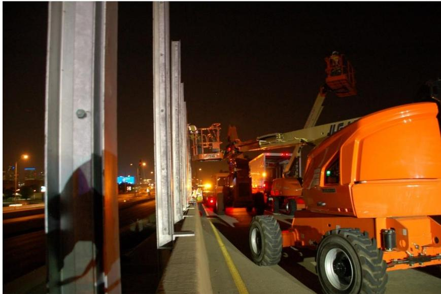
*Figure 9.40: Finalizing panel installation from the bucket truck*
