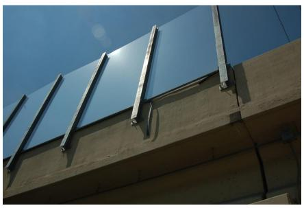
Figure 8.33: Broken horizontal rubber gasket
