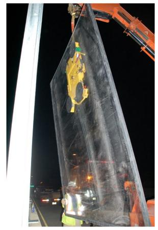
Figure 9.37: Hoisting acrylic panel
