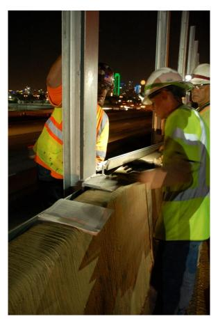
Figure 9.34: Installation of horizontal metal support
