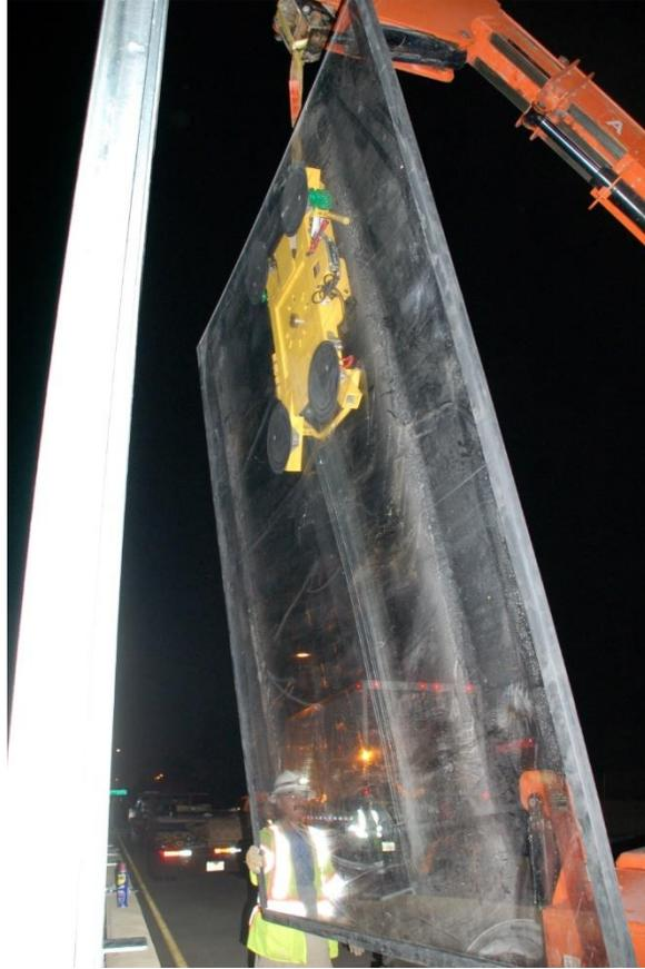
*Figure 9.37: Hoisting acrylic panel*
