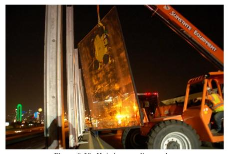
Figure 9.38: Hoisting acrylic panel
