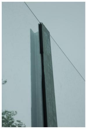
Figure 8.11: Gasket protruding from metal support
