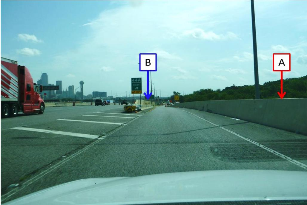
*Figure 5.14: Jersey barriers for proposed Segment A and Segment B of the Site 2 noise barrier*
