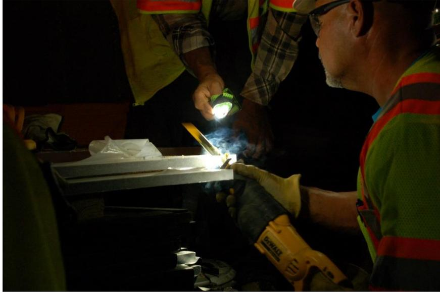
*Figure 9.33: On-site cutting of acrylic panel*
