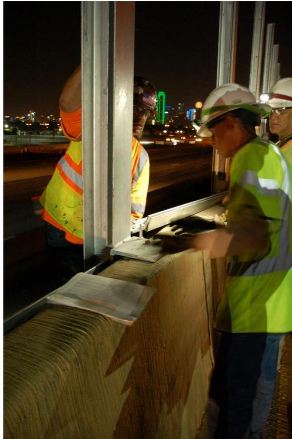
*Figure 9.34: Installation of horizontal metal support*
