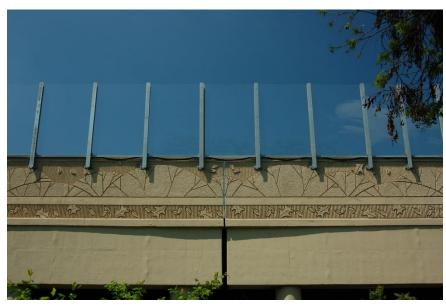
Figure 8.29: Sagging of horizontal rubber gaskets
