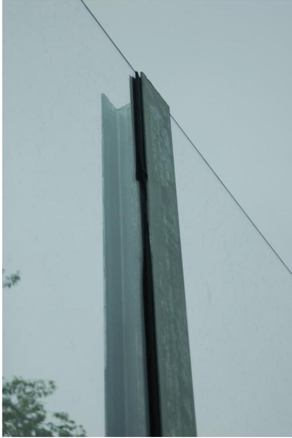
*Figure 8.11: Gasket protruding from metal support*
