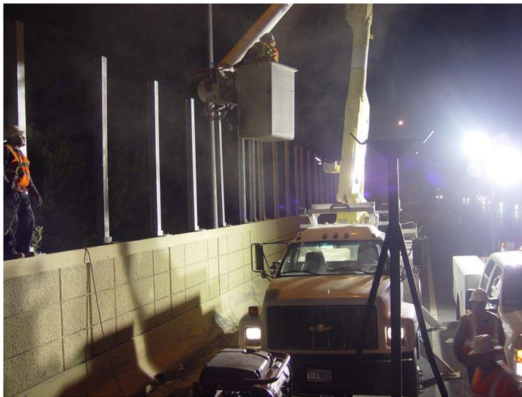
*Figure 8.2: Vertical support placement*
