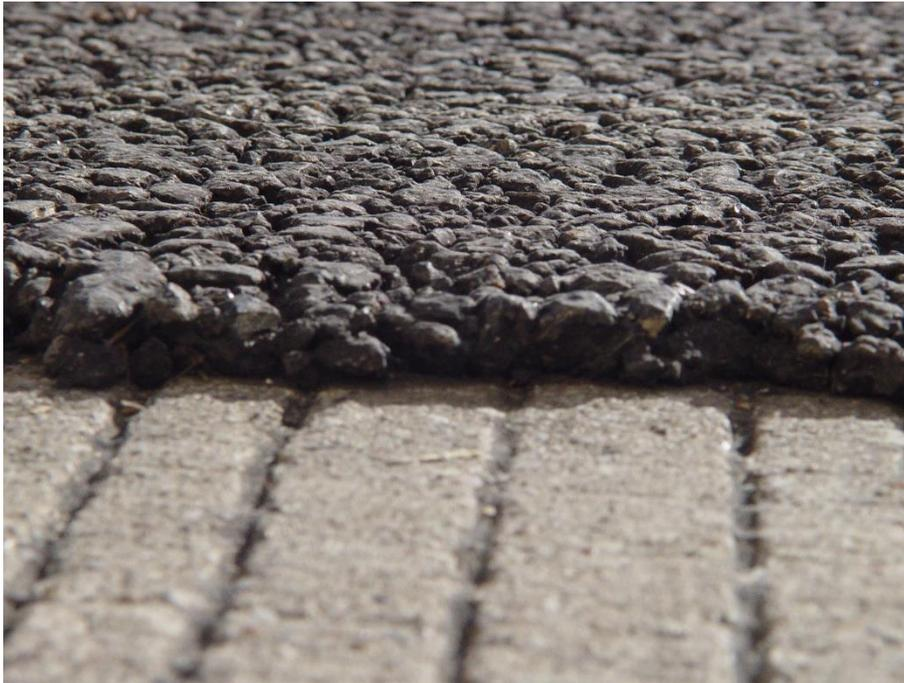
*Figure 3.20: 1-in. thick 2010 PFC overlay on IH-30 on top of CRCP (2010)*
