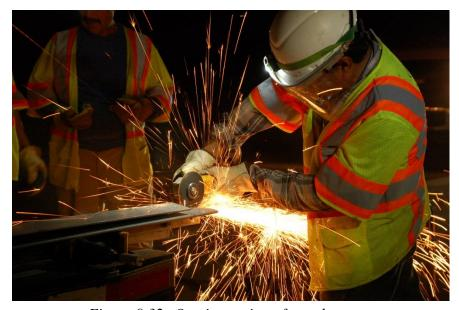
Figure 9.32: On-site cutting of metal post
