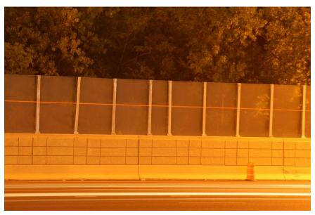
Figure 8.9: Some vertical supports off-plumb
