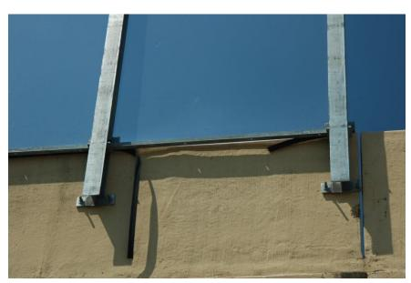
Figure 8.32: Broken horizontal rubber gasket
