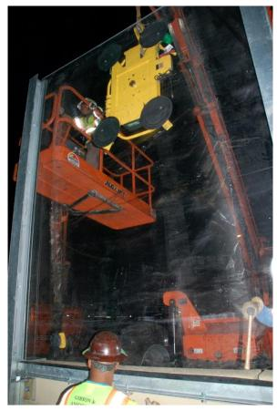
Figure 9.39: Acrylic panel installation
