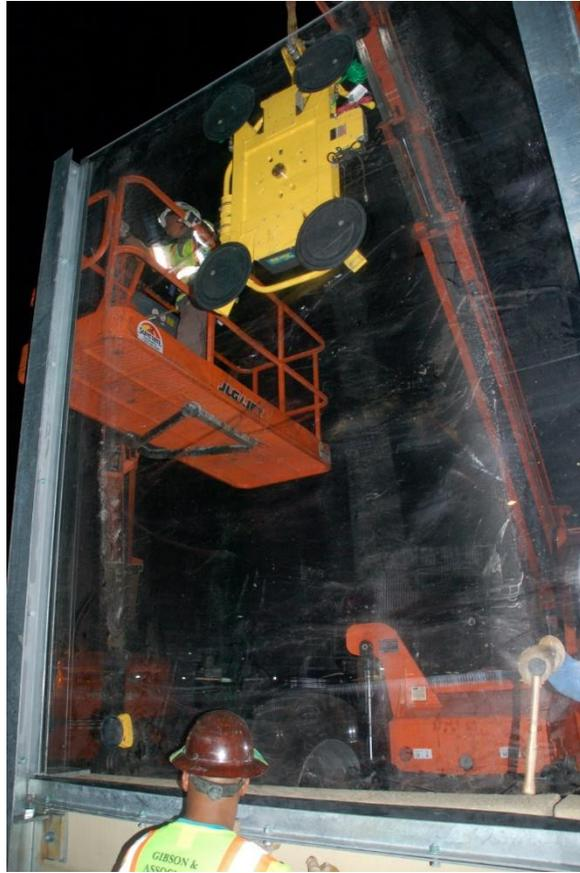
*Figure 9.39: Acrylic panel installation*
