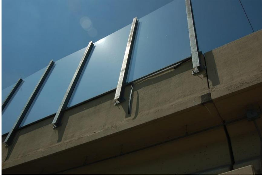
*Figure 8.33: Broken horizontal rubber gasket*
