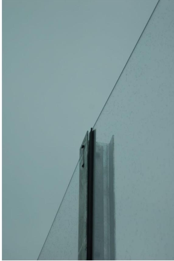
*Figure 8.12: Gap between vertical gasket and metal support*
