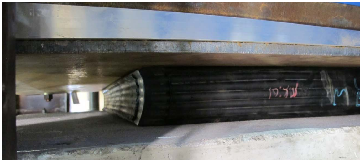
Figure 4.28: Increased local shear deformations noticeable at the compression side of the bearing
