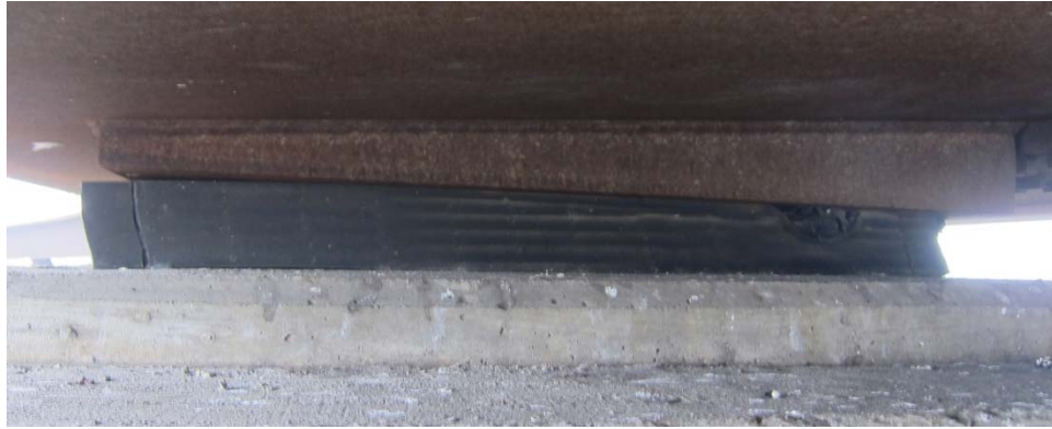
Figure 8.2: Distressed bearing for girder 1, bent 4
