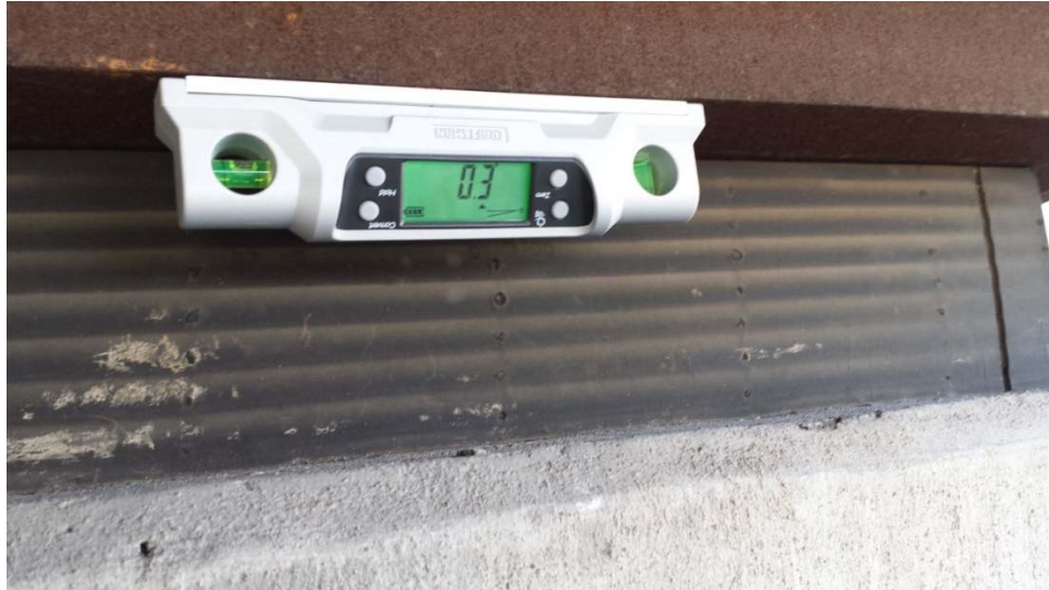
Figure 8.6: Digital level on the steel sole plate
