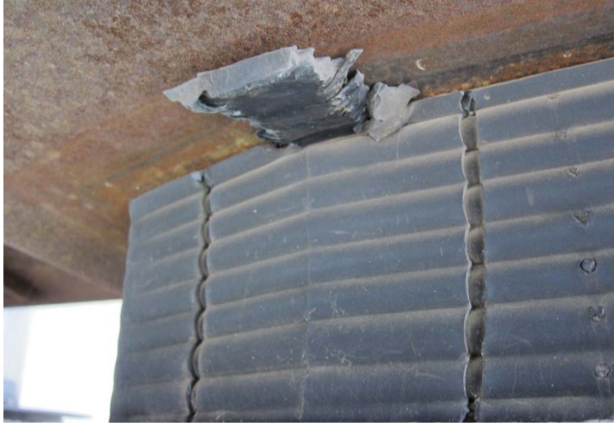
Figure 8.4: Bearing with damage for girder 1, bent 5
