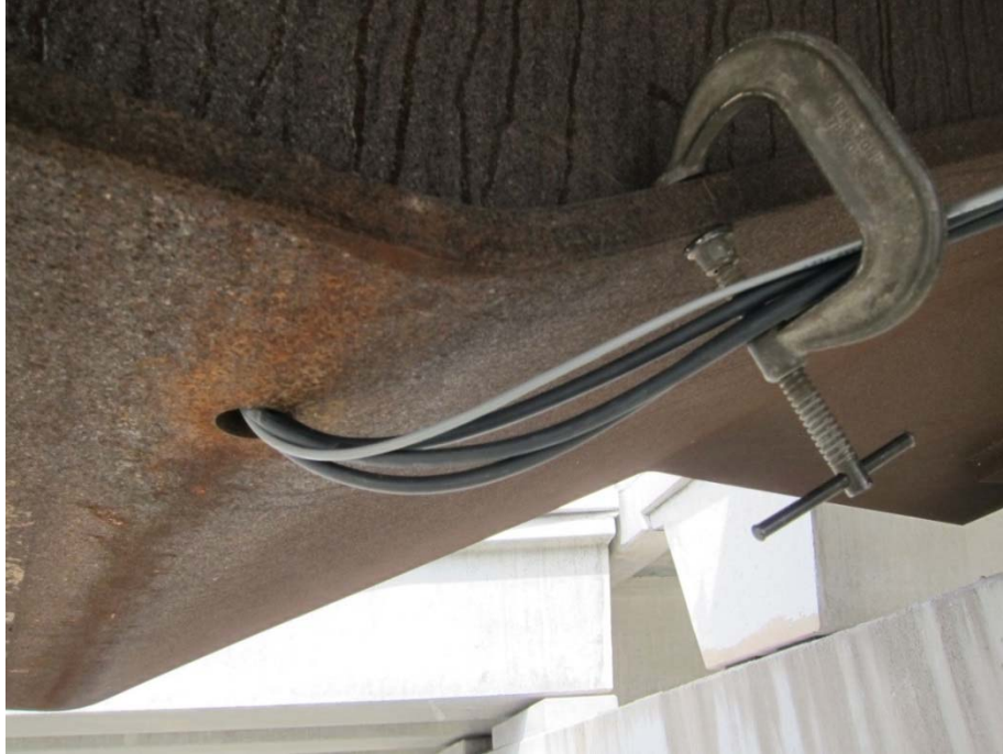
Figure 3.11: Cables from east girder entering the west girder through a hole provided for drainage
