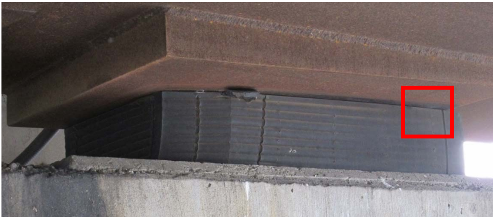
Figure 3.28: Observed slipping between the bearing and girder sole plate (Ambient Temperature at time of picture - 61 °F)
