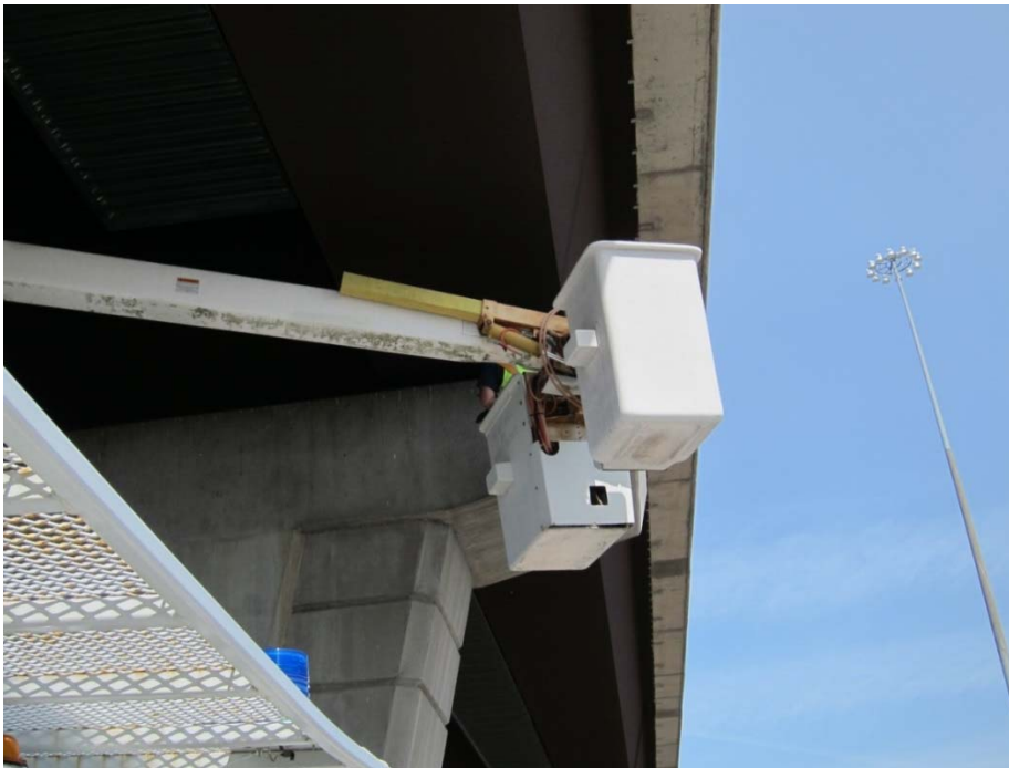
Figure 3.12: Instrumentation in the exterior of the bridge using a bucket truck
