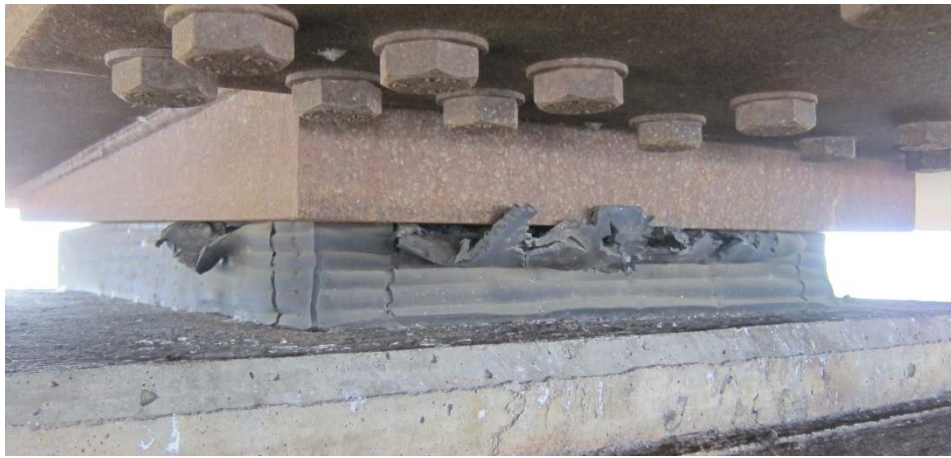
Figure 8.3: Distressed bearing for girder 1, bent 4
