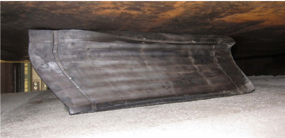
Figure 5.25: Buckled bearing M
