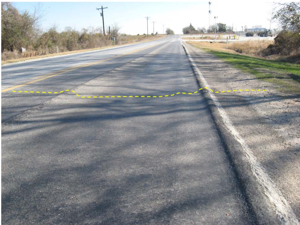
Figure 4.20: Asphalt Concrete Pavement with Wide Surface Rut Due to Repeated Heavy Loads
