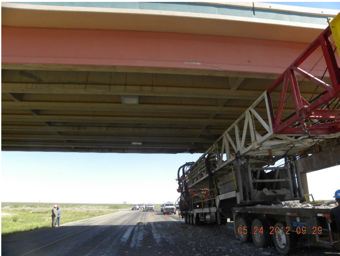
Figure 1.4: Bridge Damage from OS/OW Load at Overpass on US 385 at SH 158—Odessa District
