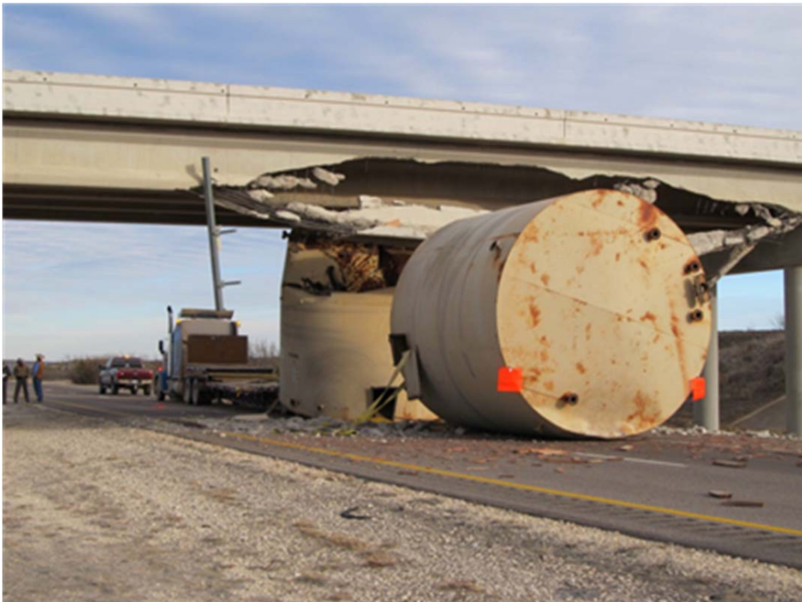
Figure 4.34: Oil Tanks Lying in the Travel Lane Immediately after Collision with a Bridge
