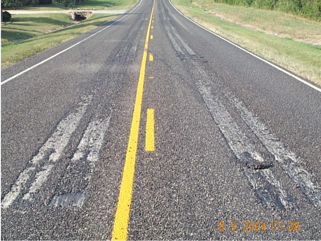
Figure 1.7: Seal Coat Damage Due to Heavy Load
