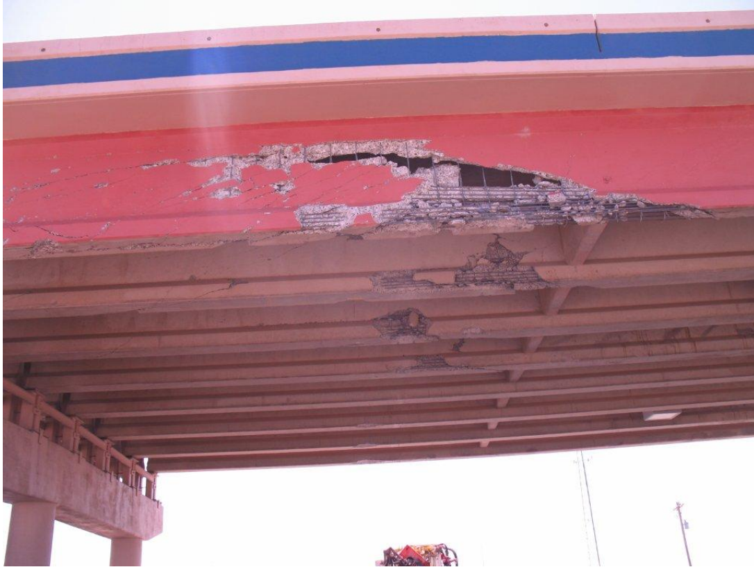
Figure 1.5: Bridge Damage from OS/OW Load at Overpass on US 385 at SH 158—Odessa District
