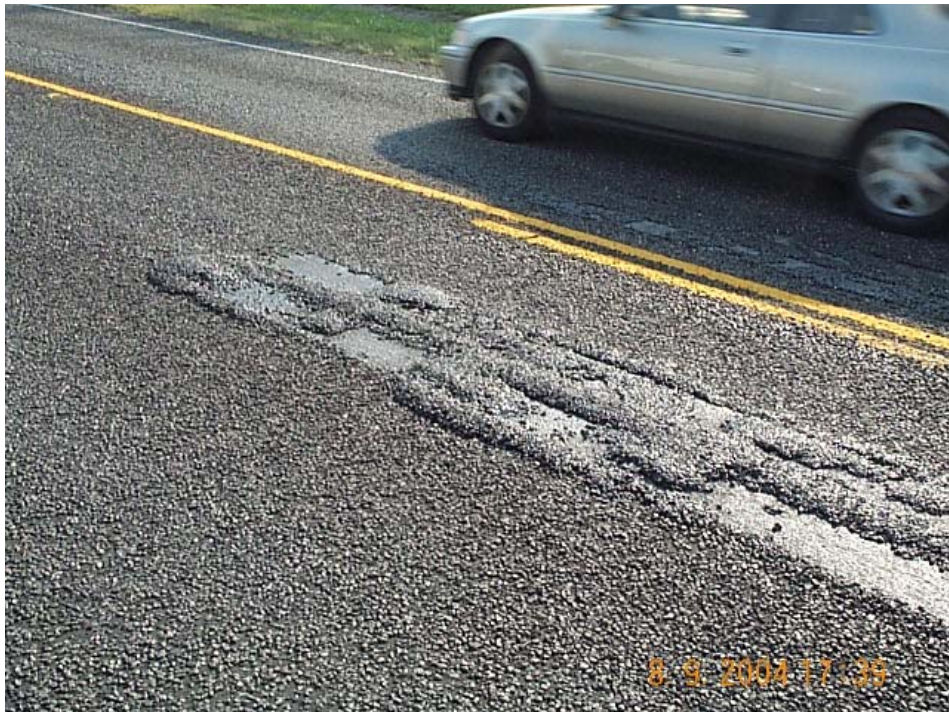
Figure 4.17: Damaged Seal Coat from Super-heavy Load Prime Mover Tandem Drive Axles
