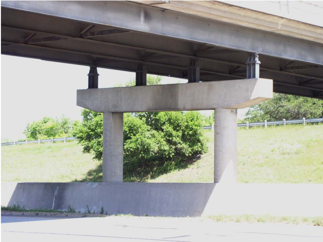
Figure 4.30: Retrofit Bridge Modifications (Pedestals) to Increase Vertical Clearance
