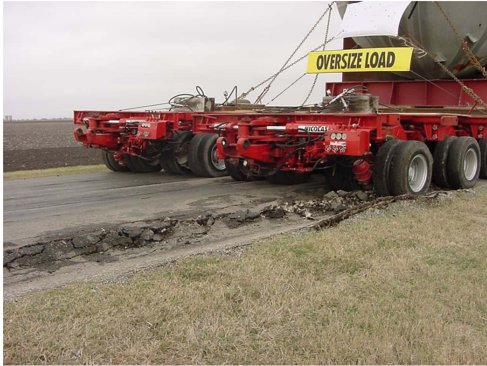
Figure 4.9: Severe Rut Damage Occurring under Heavy Wheel Loads due to Lateral Shear Failure
