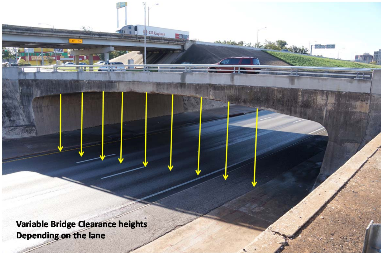
Figure 4.29: IH 35 Overpass Clearance, by Lane, to Determine Potential OS/OW Route Options
