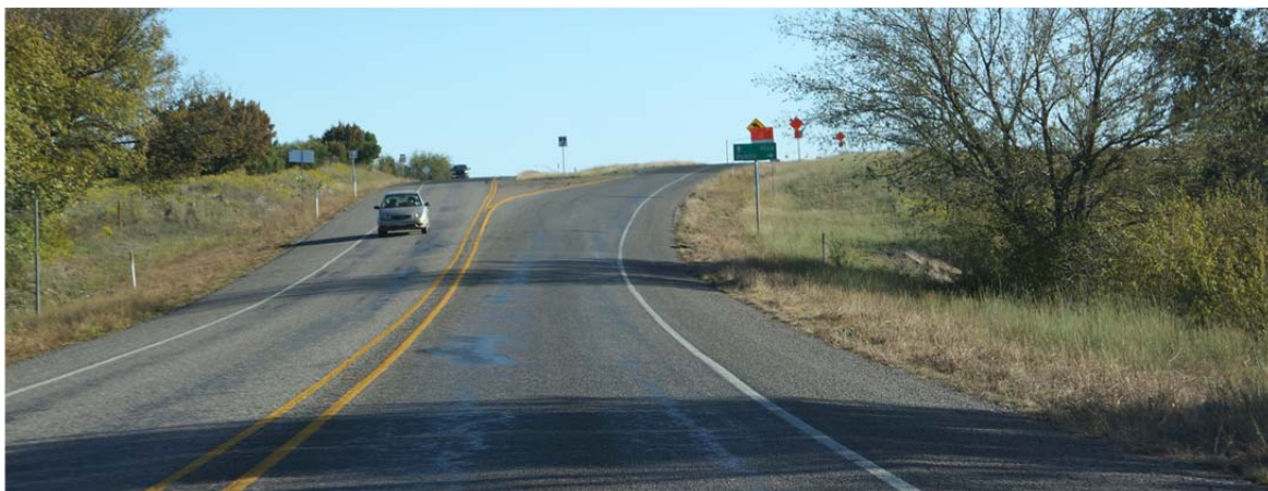
Figure 4.27: Extra-Wide Lanes within the Vicinity of a Major At-Grade Intersection along US 281
