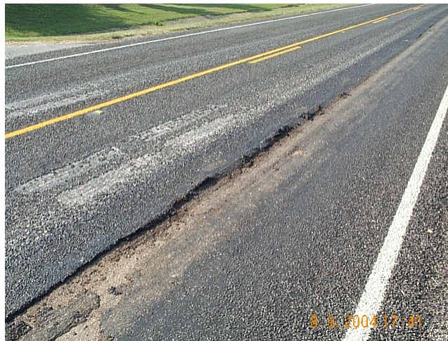
Figure 1.8: Seal Coat Damage Due to Heavy Load
