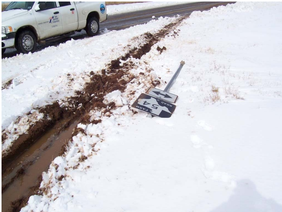
Figure 4.46: Traffic Sign Downed by Wind Turbine Loads Turning at a Rural Intersection—Lubbock
