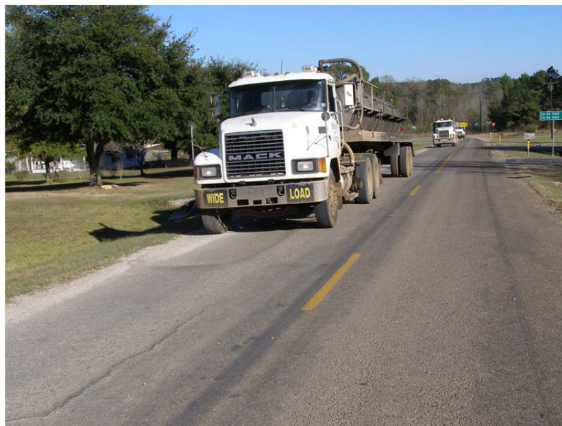
Figure 4.7: Five-Axle Tractor Trailer Unit on a Narrow FM Road with No Edge Striping or Paved Shoulder
