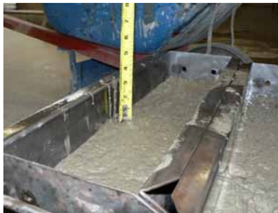
Figure 12.17: Casting the bottom layer of fatigue-corrosion beams
