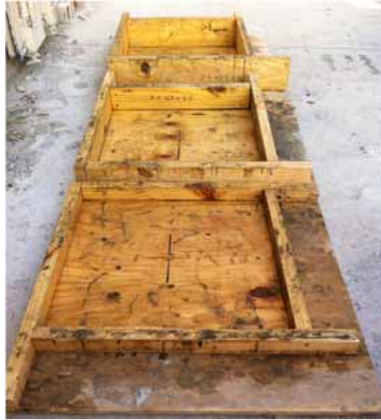
Figure 7.25: The three temperature gradient slabs formwork
