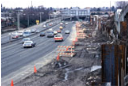
Figure 12. Tri-Met MAX Light Rail in Portland under Construction in 1980 (Source: www.trimet.org )
