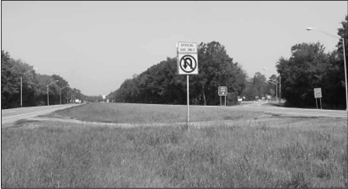
Figure 58. Emergency Crossover (Source: Barton, 2011)
