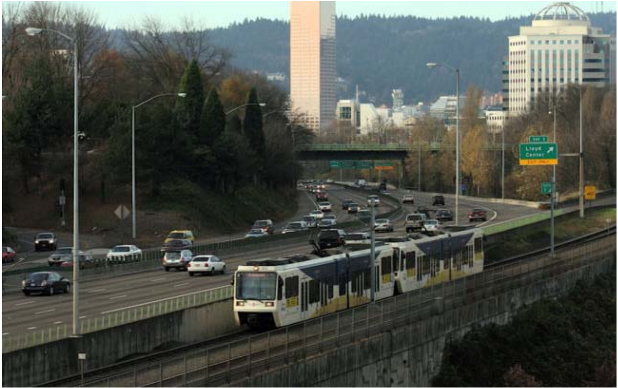
Figure 13. Portland MAX Light Rail next to Banfield Highway (Interstate 84)
