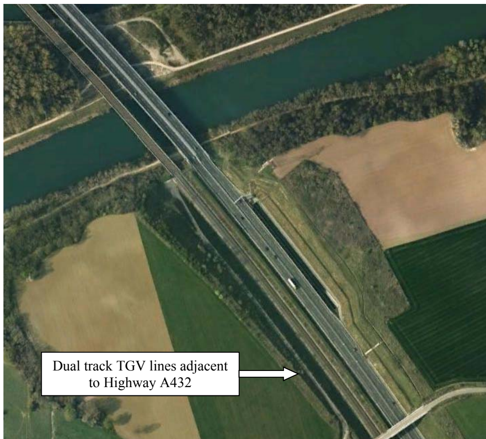
Figure 3. French TGV Route Parallel to Highway A432 near Lyon, France (Source: Google Earth)
