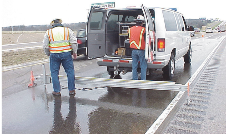
Figure 2.2: MLS transverse profile beam used on IH 35 during an accident investigation
