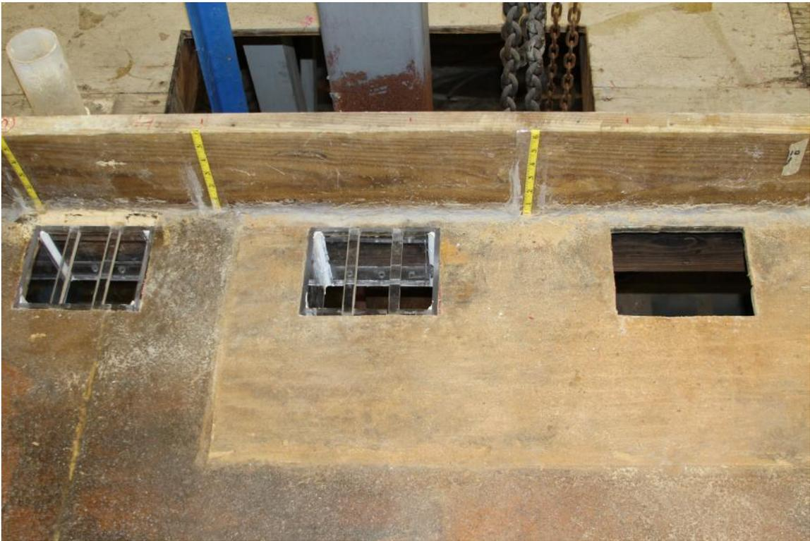
**Figure B-14 6in. × 8in. Drain Installation**
