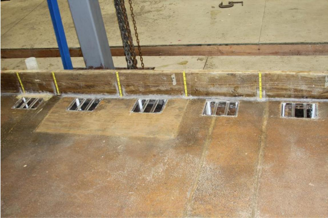
**Figure B-15 Finished 6in. × 8in. Drain Installation**
