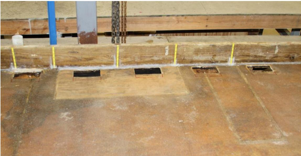
**Figure B-12 6in. × 8in. Drain Placement**
