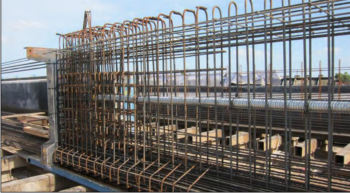
*Figure 3.16: End-block reinforcing cage of Tx62-7*
