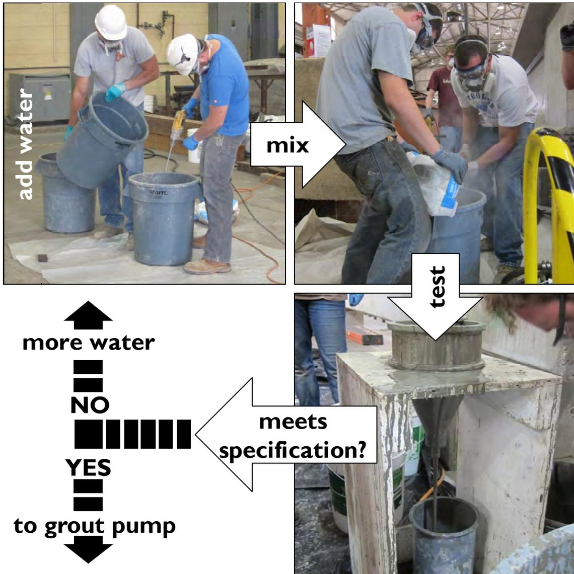
Figure 3.23: Grout mixing procedure
