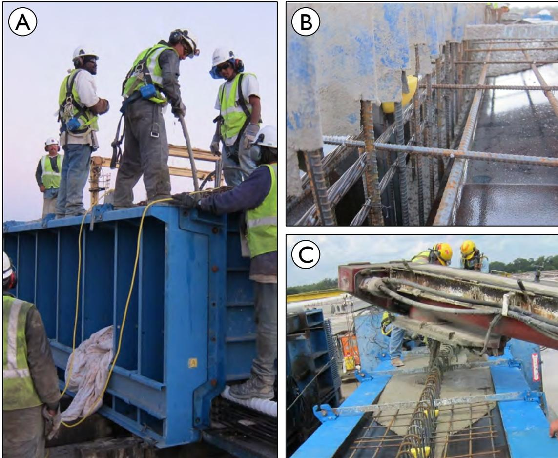
Figure 3.17: Concrete Consolidation (A) “Stinger” Type Vibrators Used within End-Block & (B), (C) Self-Consolidating Concrete Flow
