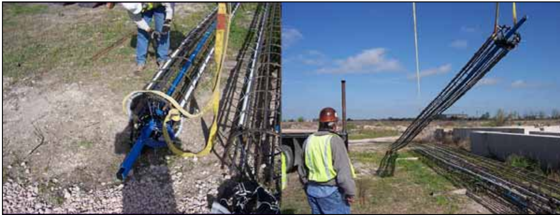
Figure 4.15: Lifting an instrumented cage with two cranes.
