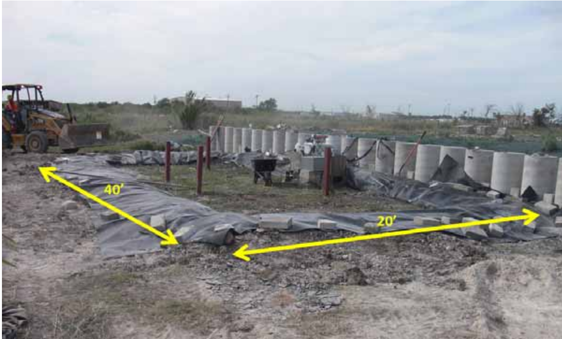
Figure 4.34: Completed inundation berm.
