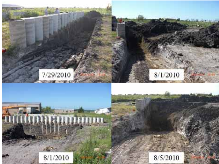
Figure 5.5: Photos of initial excavation progress (7/29/2010–8/5/2010).
