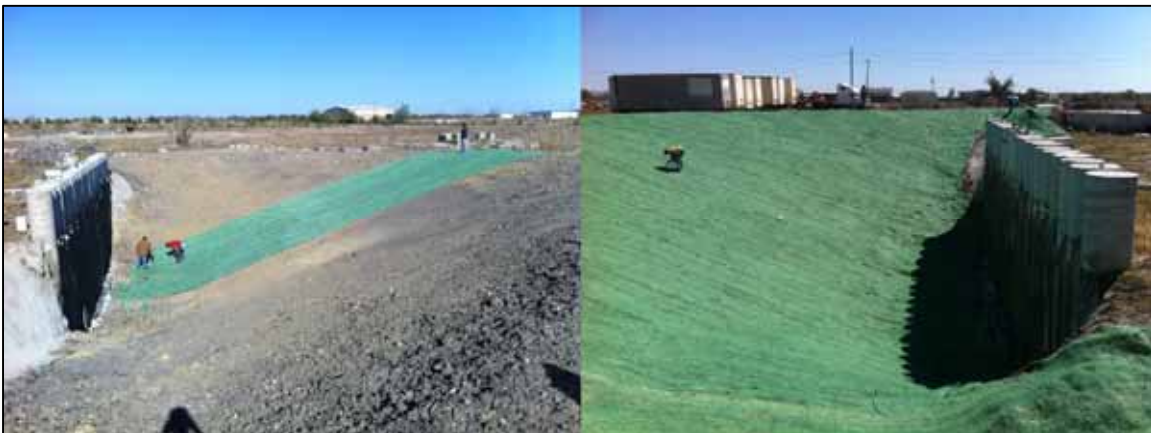
Figure 4.21: Erosion control material is installed on October 18, 2011.
