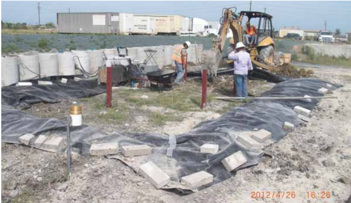
Figure 4.32: Compacting soil with backhoe bucket.
