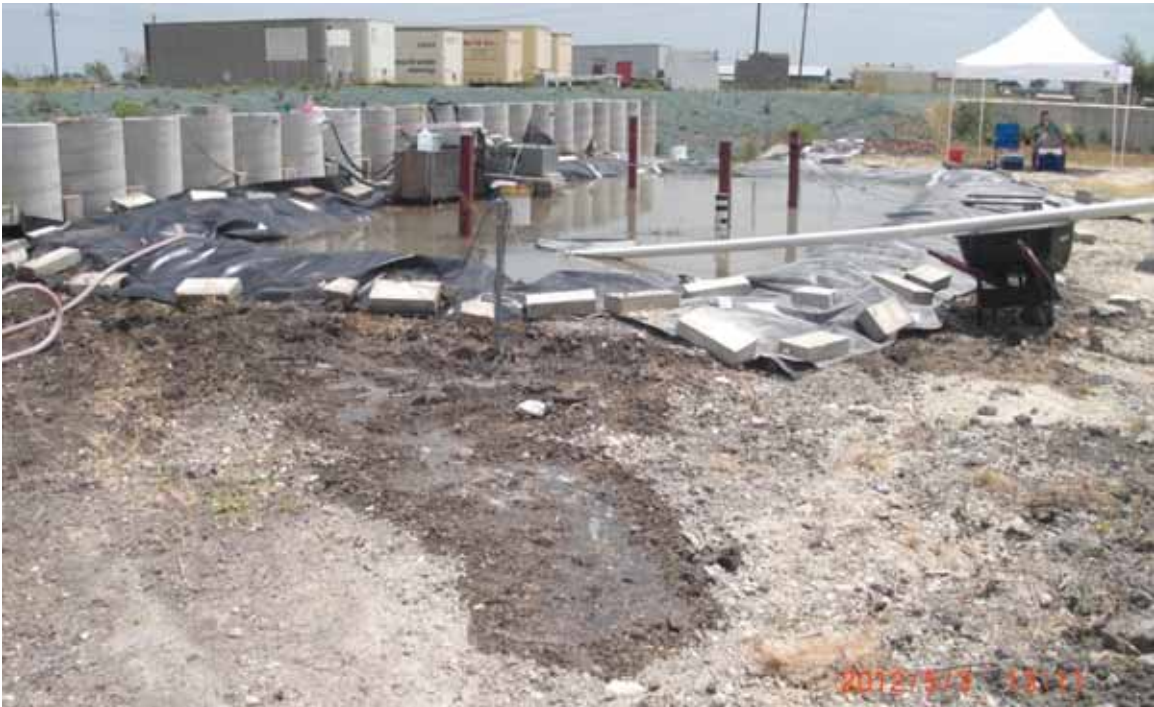
Figure 4.37: Leakage from west side of inundation zone.
