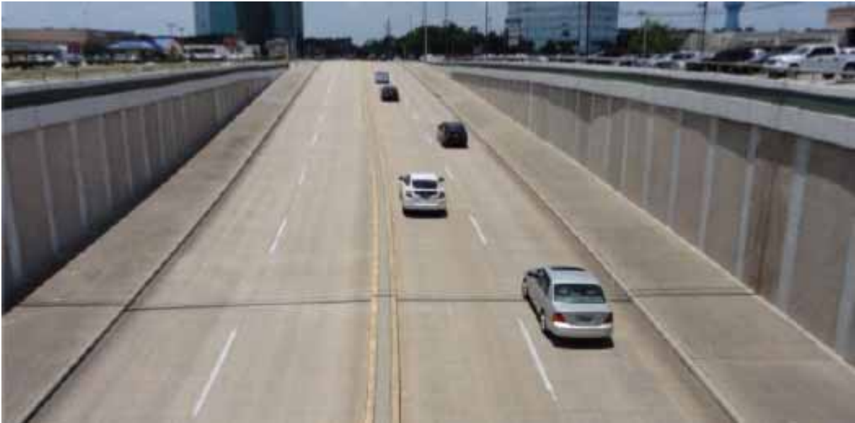
Figure 3.35: View of current wall conditions, facing west.
