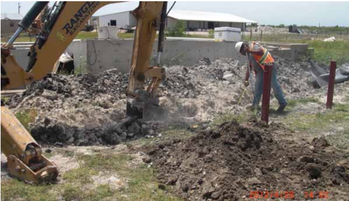
Figure 4.31: Compacting soil with backhoe bucket.
