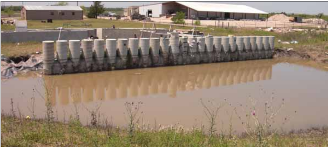
Figure 5.26: Flooding in response to a large storm before the May 6, 2013, data surveys. Water level in the excavation reached ground surface.
