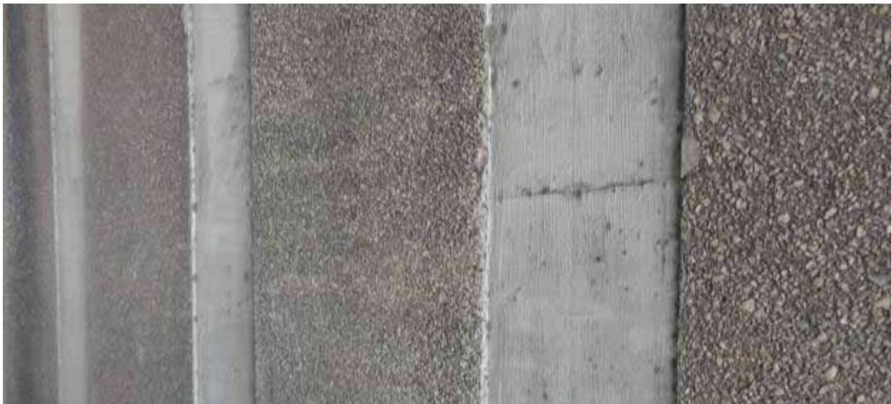
Figure 3.36: Example of imperfection in white concrete facing, possibly caused by a seam in the plywood formwork.
