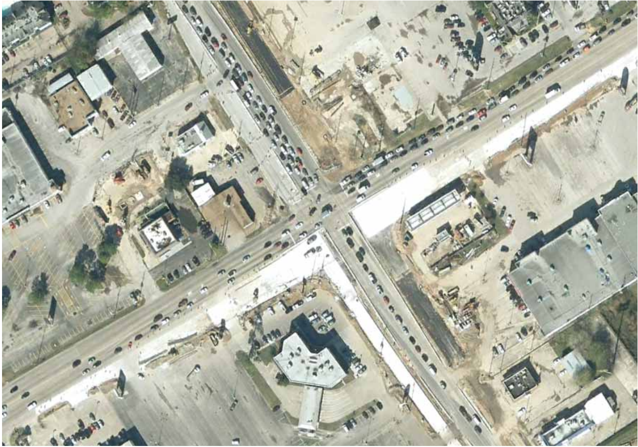
Figure 3.2: Aerial view of project area before excavation (image date: January 2008) (Google Inc., 2011).
