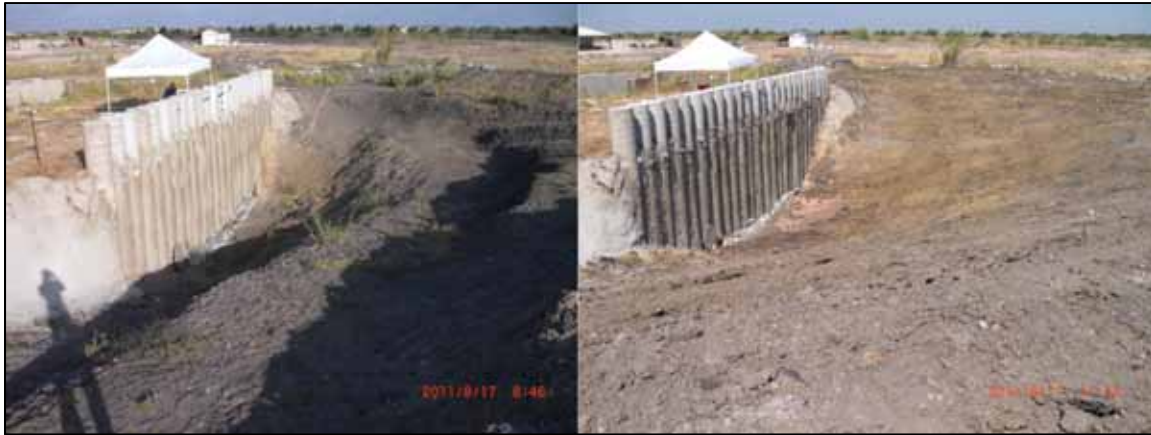
Figure 4.20: Excavation slopes are reshaped on August 17, 2011.
