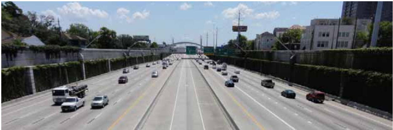
Figure 3.31: Large-scale view of project area (facing east). Sound wall is located above the main retaining structure.
