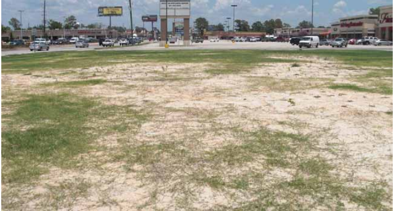
Figure 3.30: Unpaved area near southeast corner of intersection.
