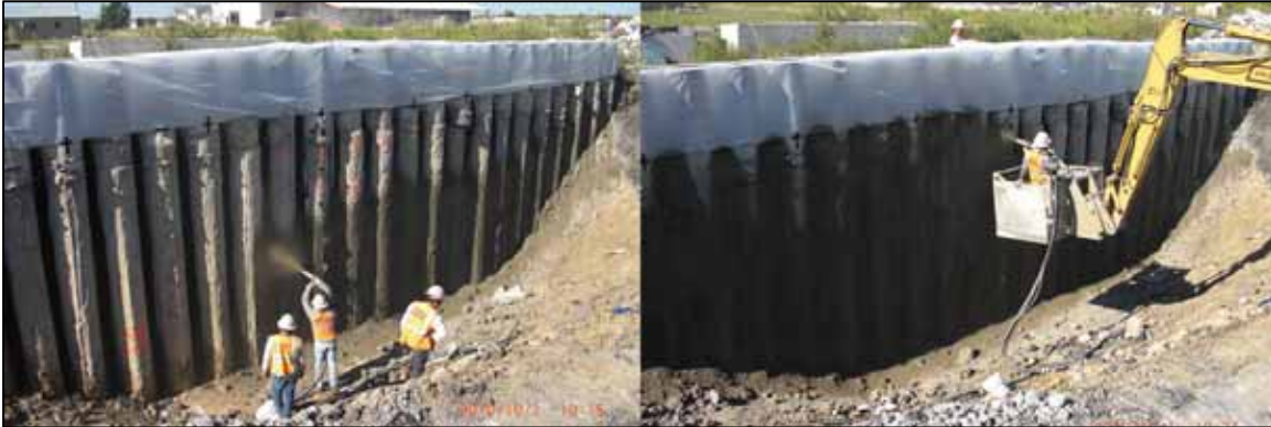
Figure 4.16: Installation of shotcrete facing on October 1, 2010.
