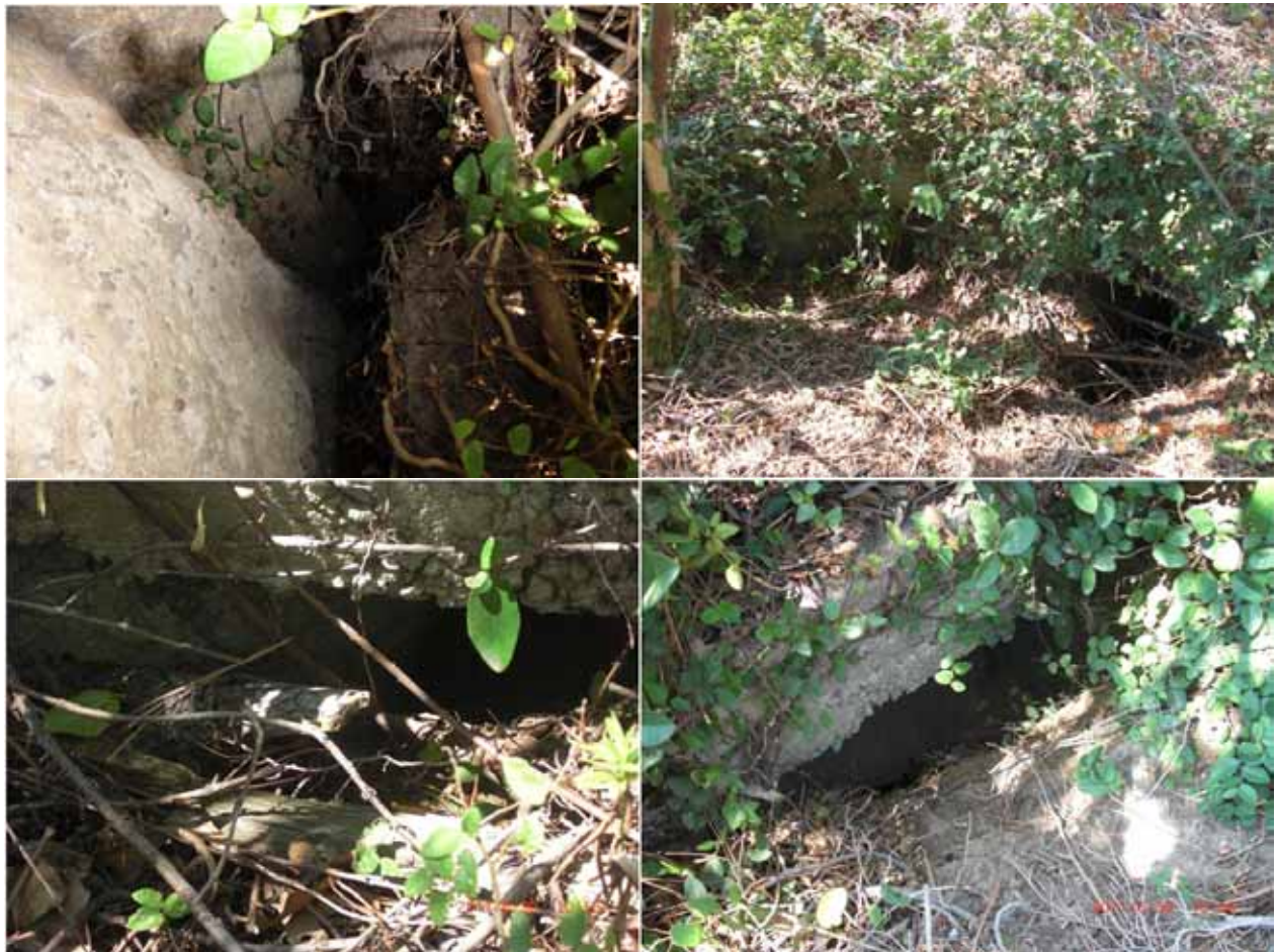
Figure 3.34: Several gaps were observed between the shafts and the soil behind the wall.
