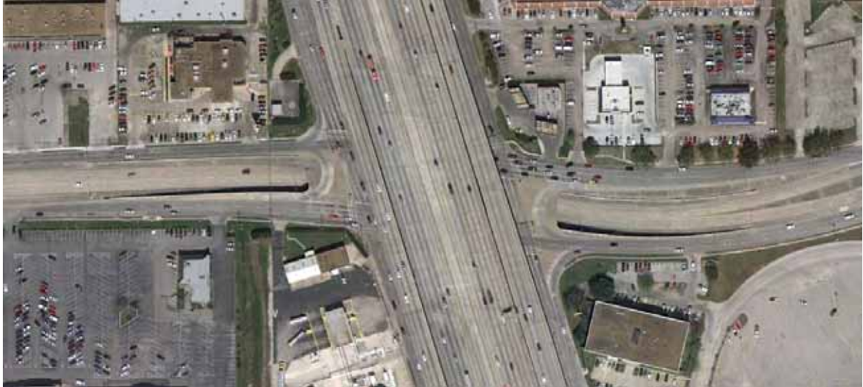
Figure 3.10: Aerial view of the project area after completion (image date: March 2011) (Google Inc., 2011).
