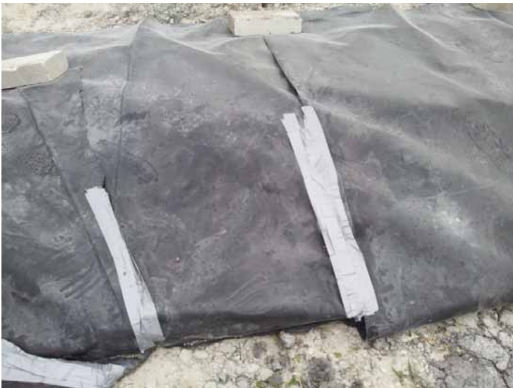
Figure 4.33: Detail of geomembrane seam.
