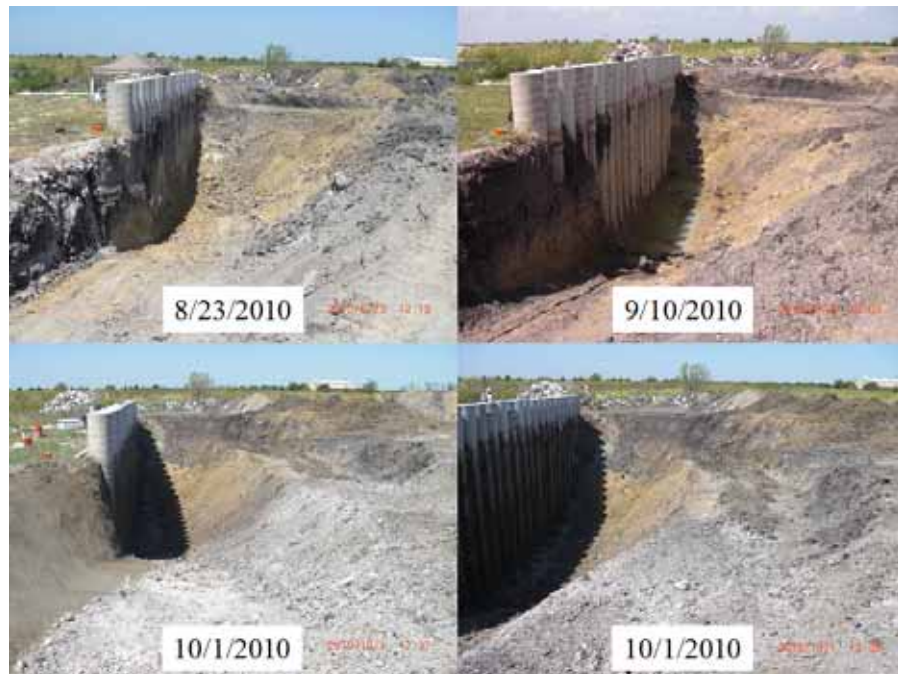
Figure 5.6: Photos of later excavation progress (8/23/2010 - 10/1/2010).
