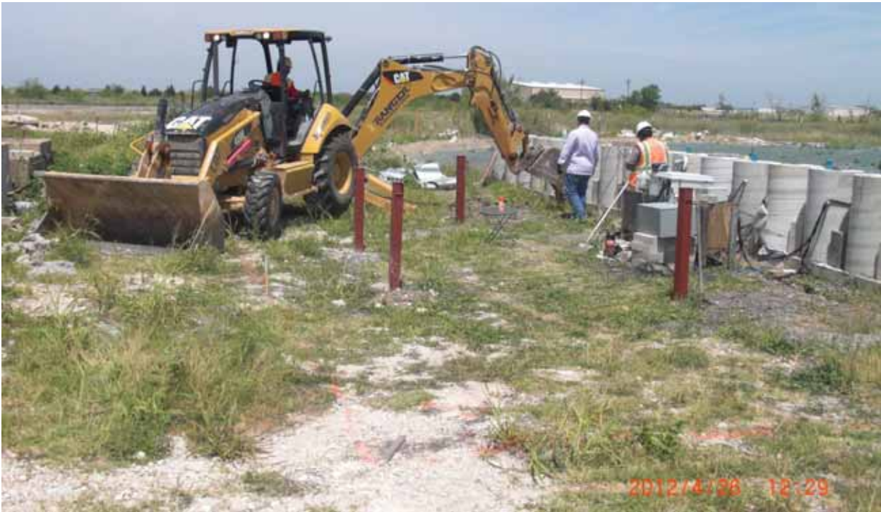
Figure 4.29: Excavation of trench for inundation berm.
