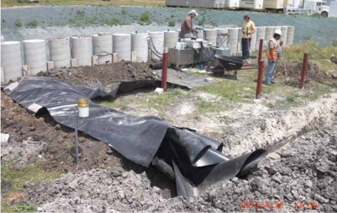
Figure 4.30: Installation of geomembrane in trench.
