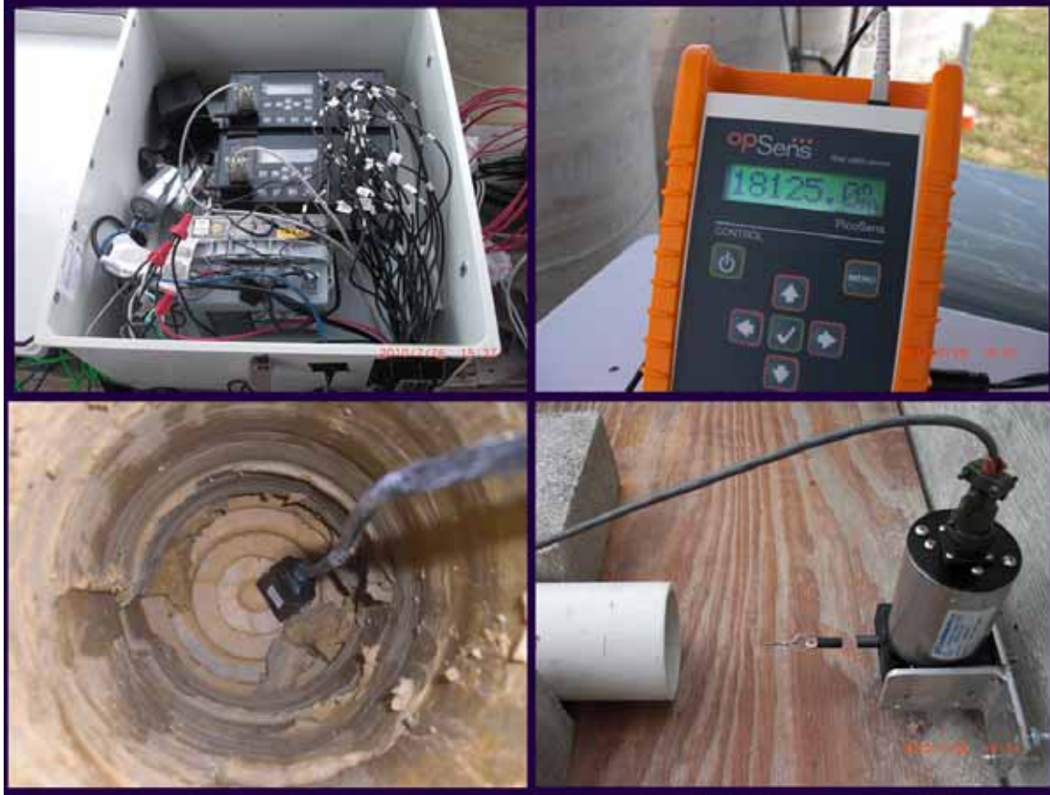
Figure 4.13: Instrumentation on the project site. Clockwise from top left: temperature resistant datalogger and enclosure for continuous strain readings; signal conditioner for individual strain readings; linear potentiometer; TDR probe installed through facing.
