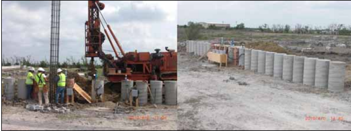
Figure 4.14: Construction of test wall, April 2010.
