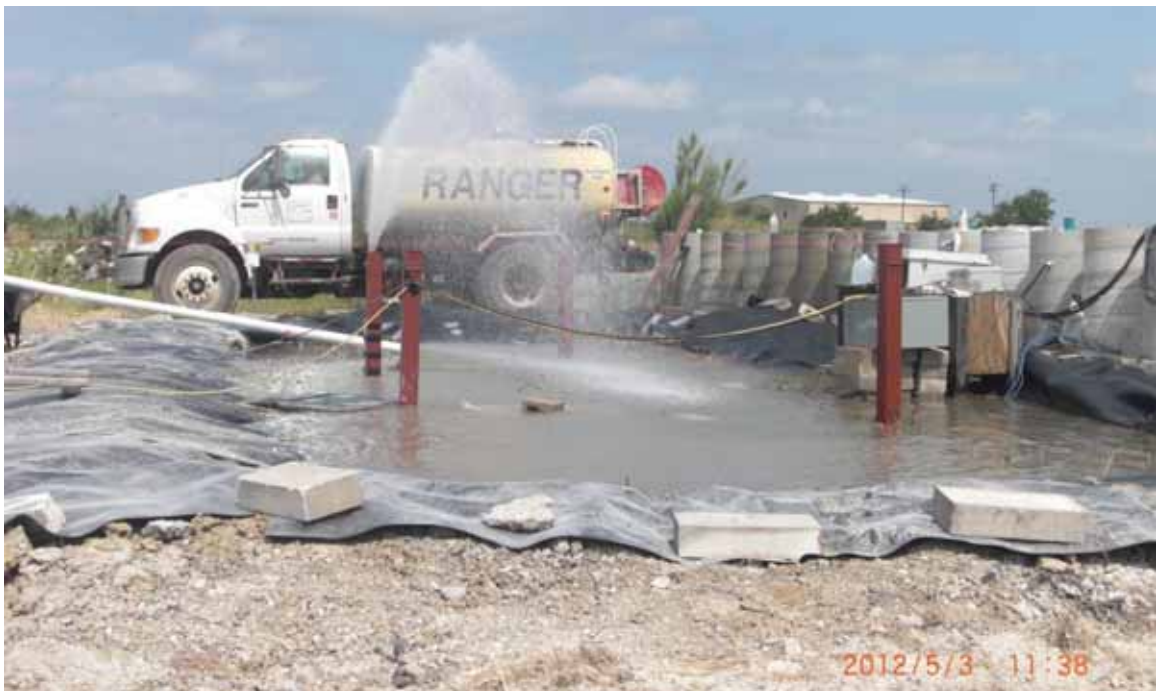
Figure 4.35: Filling the inundation zone.
