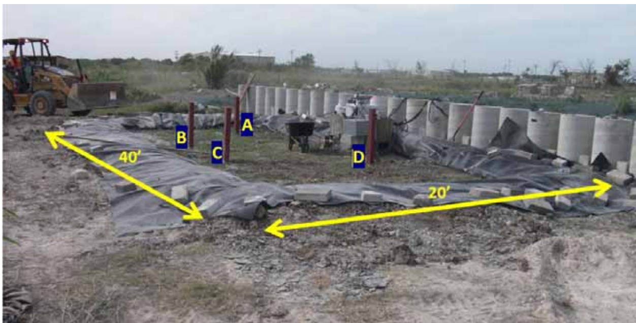
Figure 4.26: The four standpipe piezometers installed behind the wall in the inundation berm.
