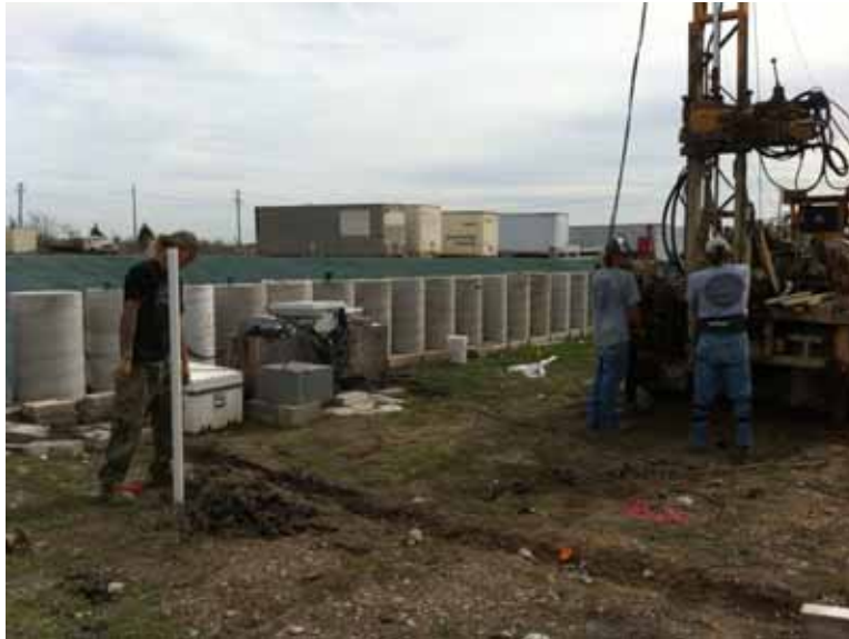
Figure 4.25: Piezometer being installed in borehole A.
