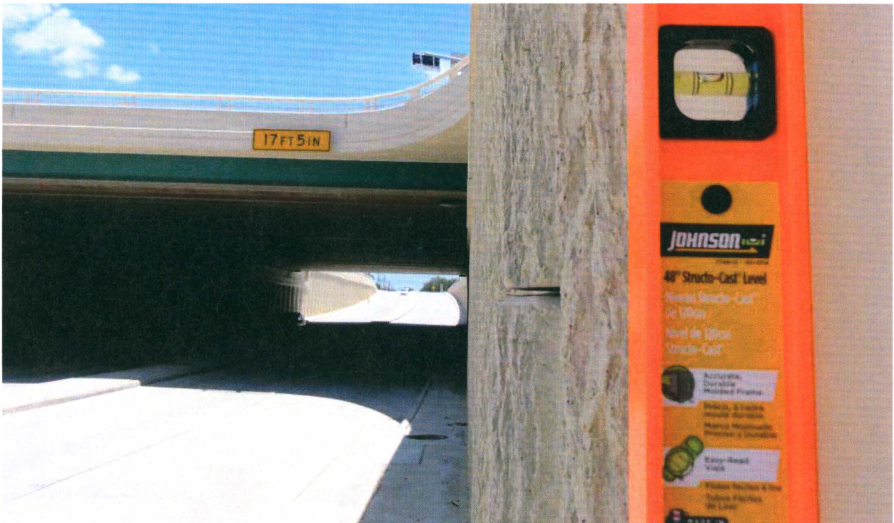
Figure 6.2: Wall facing was observed to be vertical and in good condition throughout the project area.
