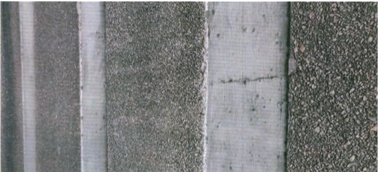
Figure 6.11: Example of imperfection in white concrete facing, possibly caused by a seam in the plywood formwork.
