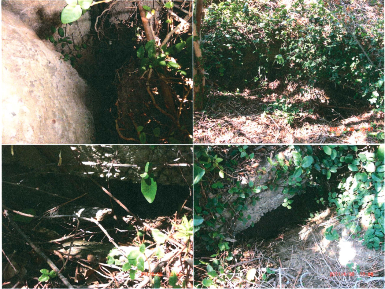
Figure 6.9: Several gaps were observed between the shafts and the soil behind the wall.
