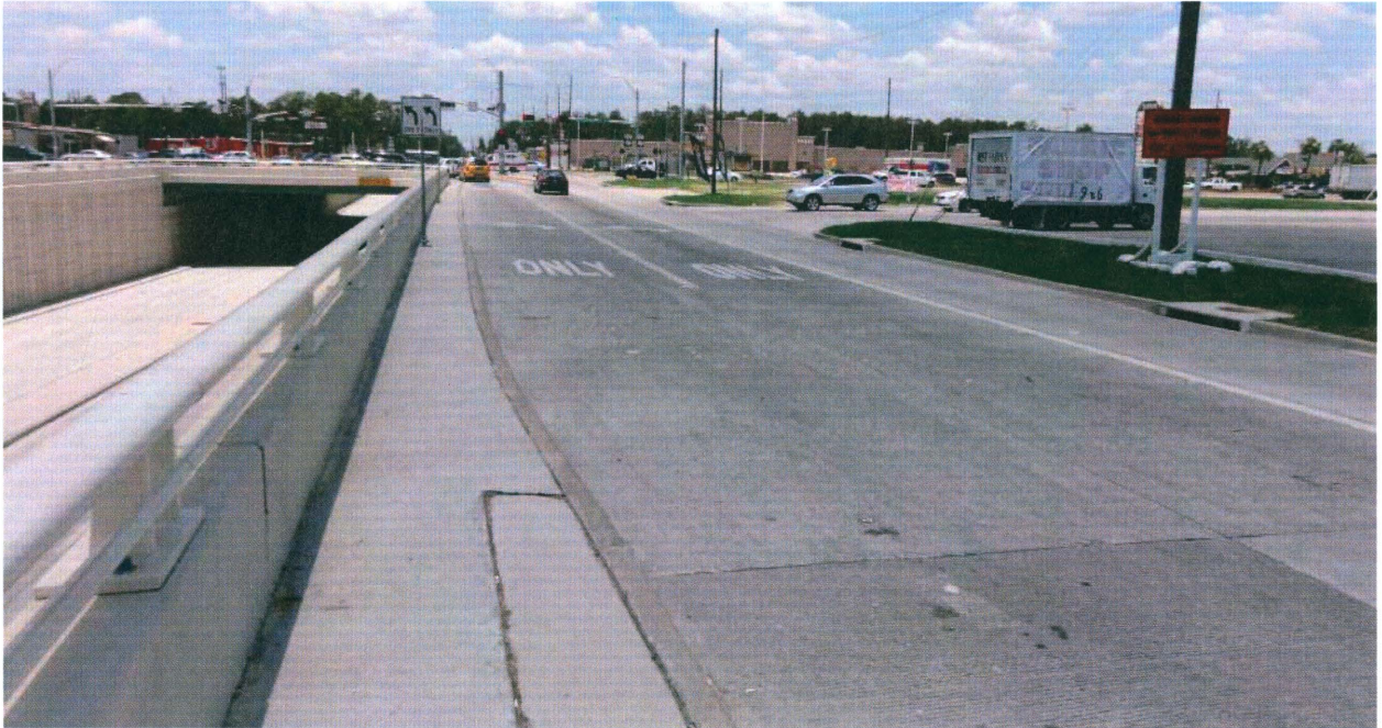
Figure 6.3: Paved area behind the wall. In all locations, pavement extends at least 30 feet behind the wall.
