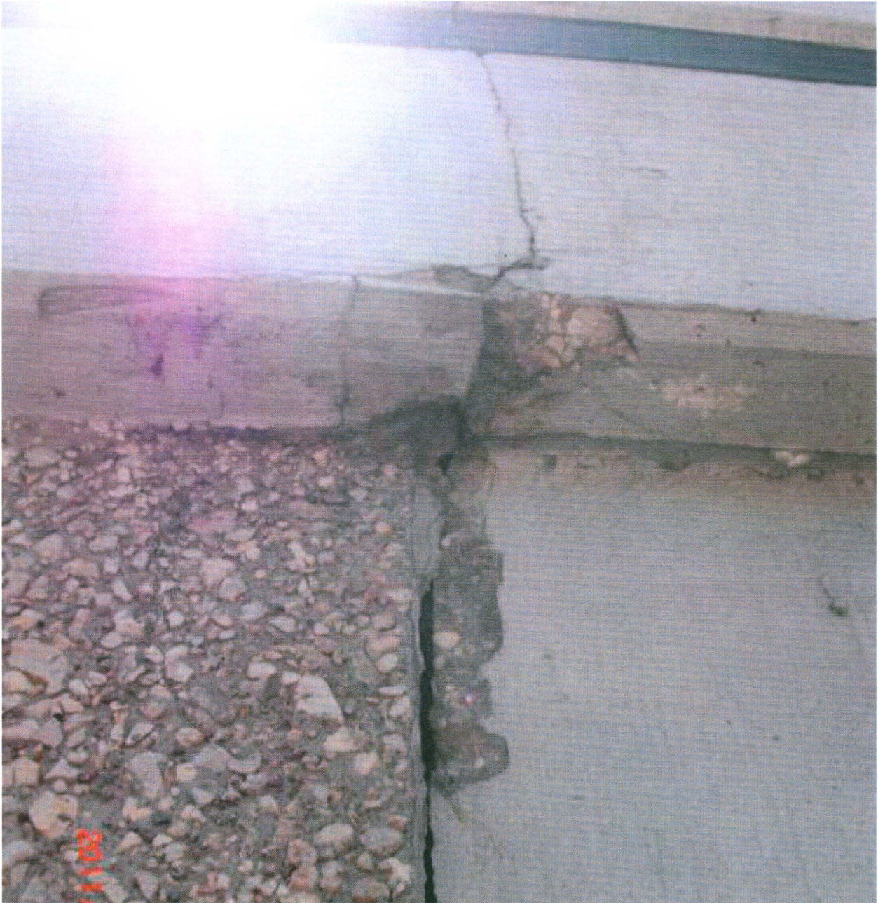
Figure 6.13: Some cracking was seen at the connection between two facing panels on the southwestern portion of the wall.
