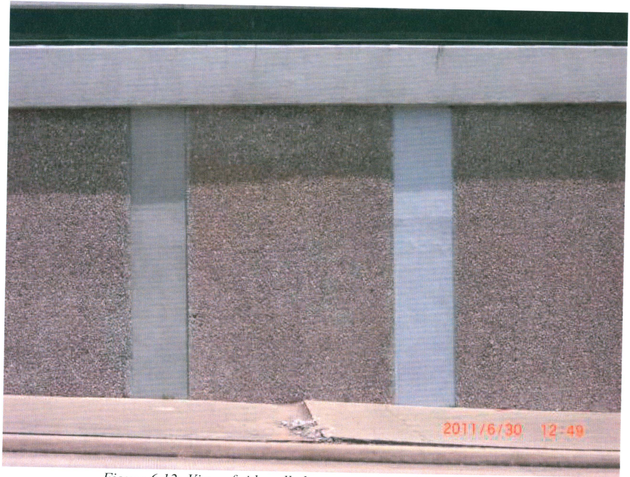
Figure 6.12: View of sidewalk damage along the base of the wall.
