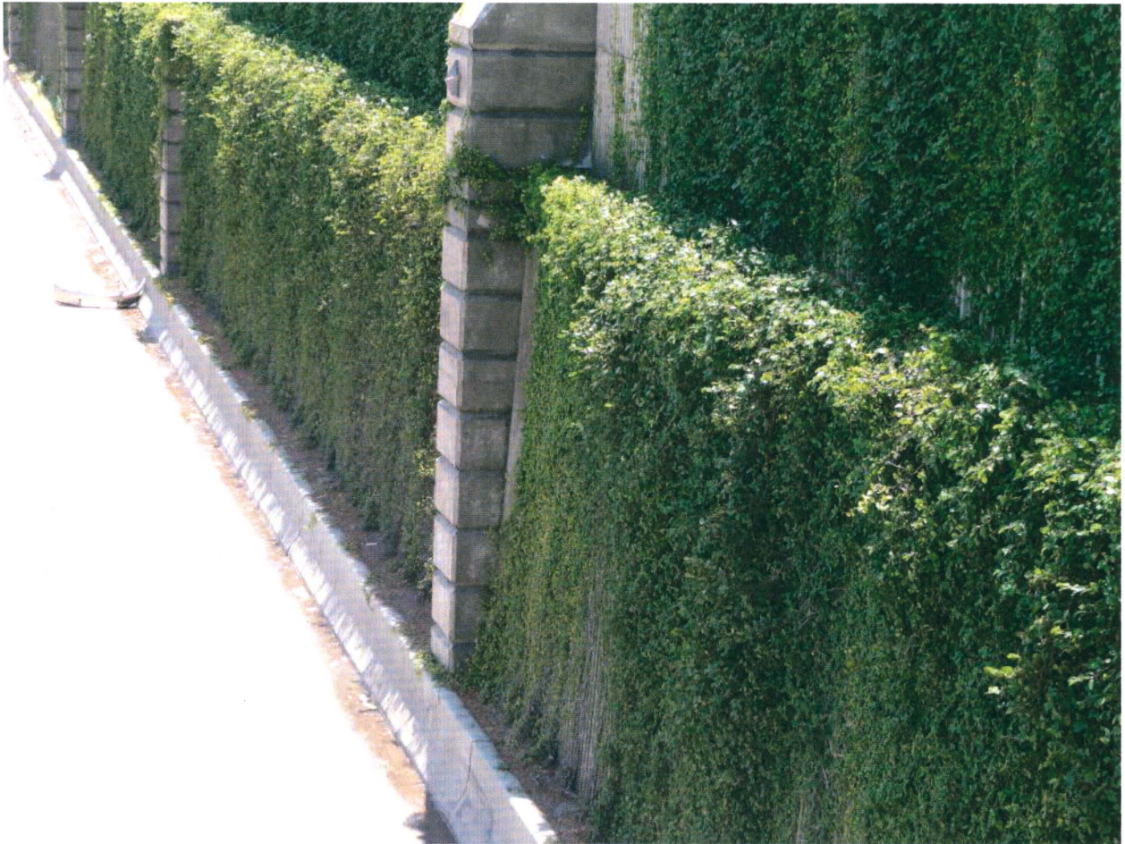
Figure 6.7: Dense vegetation and batter angle on concrete facing panels. Sound wall is located above main retaining structure.
