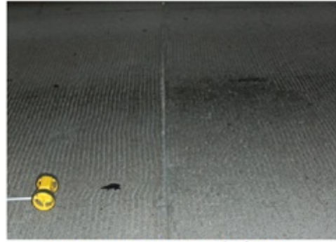
Transverse joint at end of BCO (Westbound direction)
