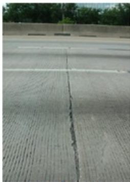
Joint damage
