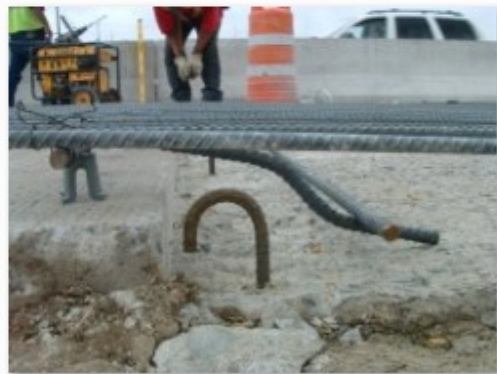
Close-Up of Reinforcement at Transition
