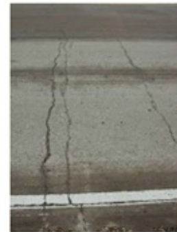
Picture 4 Area of potential punchout (RM 51 + 214 ft)
