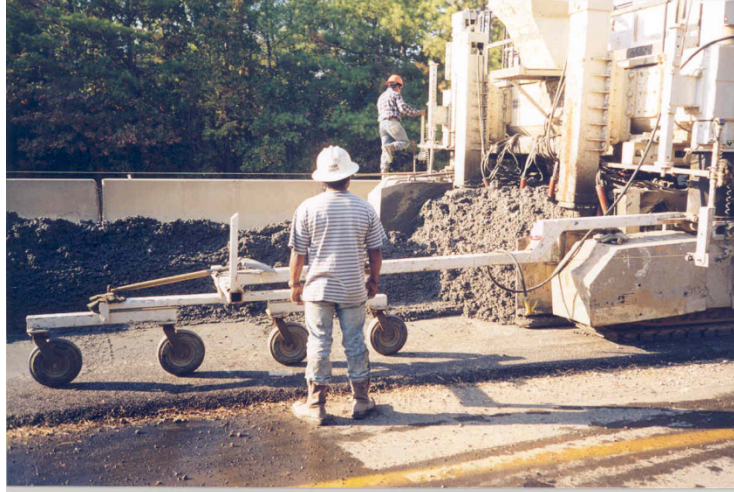
Figure 7.9: Existing pavement, 2-in. thick asphalt separation layer, and concrete overlay placement
