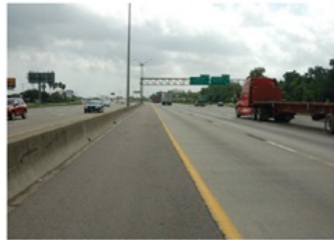
View east of MLK Blvd. 1989-1990 Experimental sections (EB)
