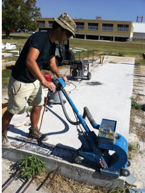
Figure 4.12: Shotblasting in progress
