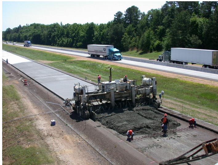
Figure 2.11: Prompt curing following the paver
