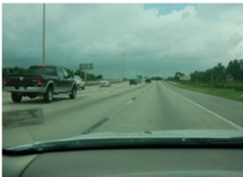
Survey from the vehicle Eastbound outside lane. 1990 BCO
