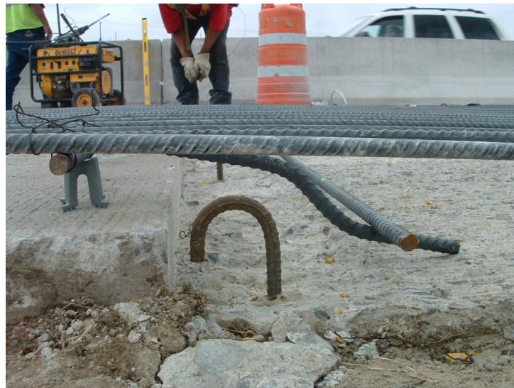
Figure 3.8: Transition reinforcement detail close-up
