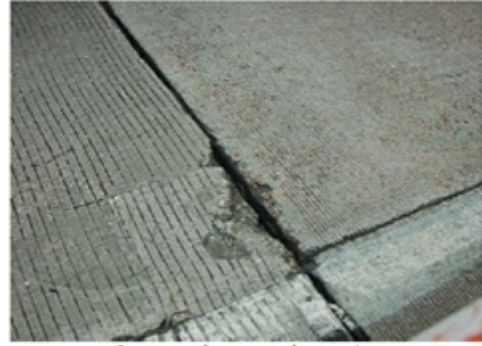
Corner damaged repair
