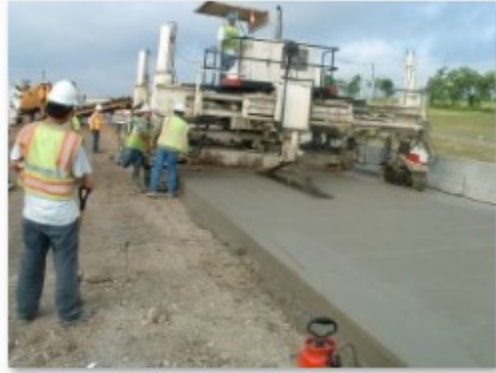
Following the Paver
