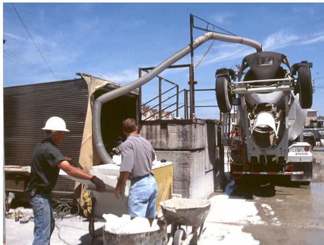
Figure 2.9: Blowing the fiber into the mixing truck
