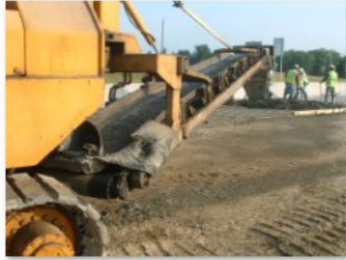
Start of Construction
