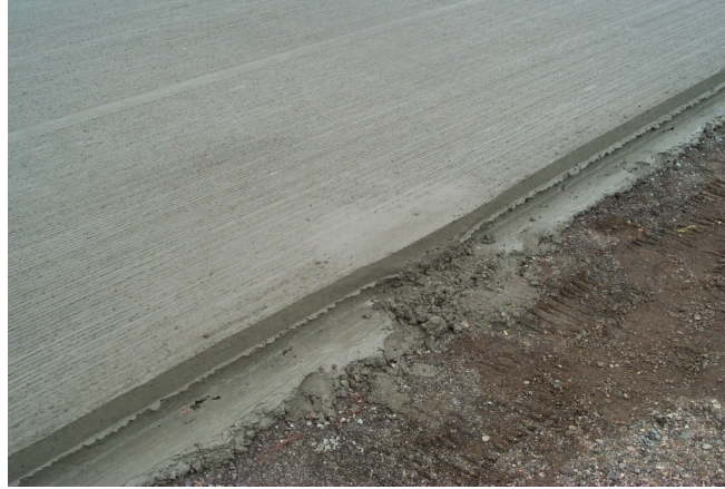
Figure 7.10: Carpet dragged surface texture
