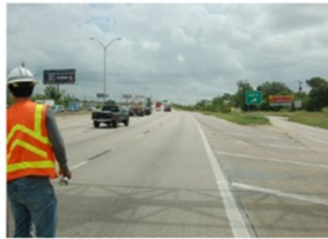
Beginning of survey- 1983 BCO EB outside lane, after Cullen Blvd. overpass, exit 36A
