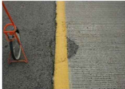
Small AC patch 1989-1990 Experimental sections (EB)
