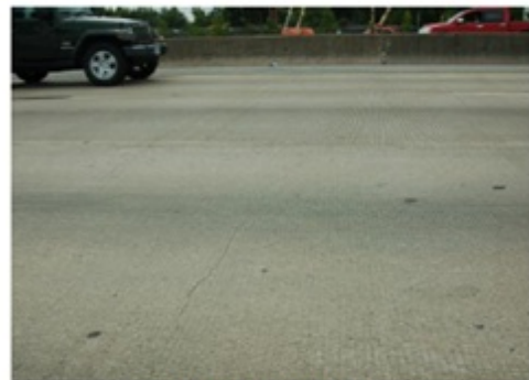
Transverse cracks
