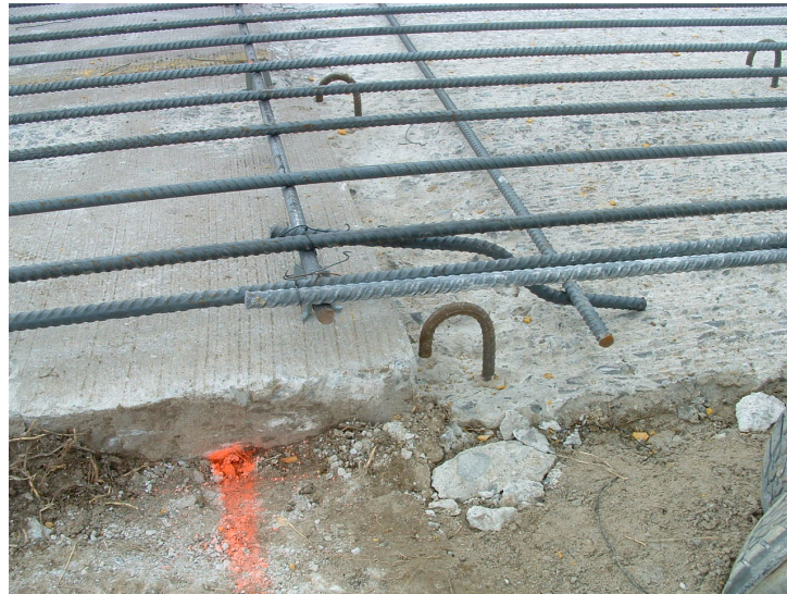
Figure 3.7: Transition reinforcement detail
