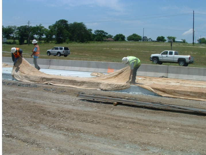
Figure 3.13: Laying down burlaps
