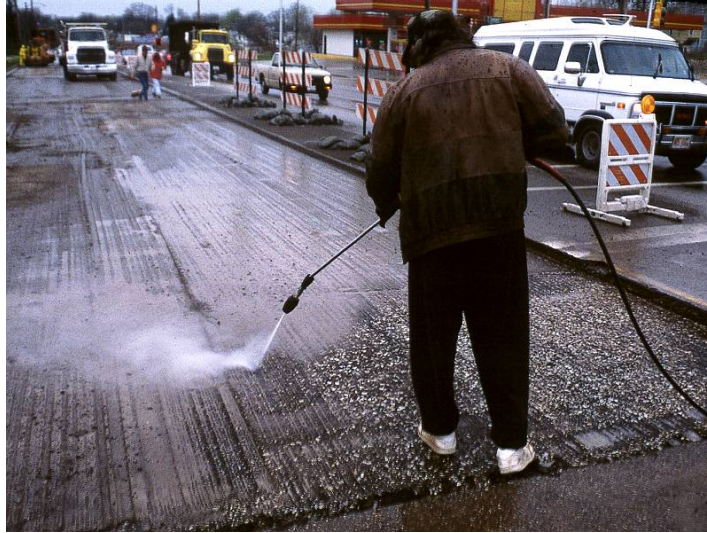
Figure 2.8: Cleaning the surface with hydro cleaning equipment
