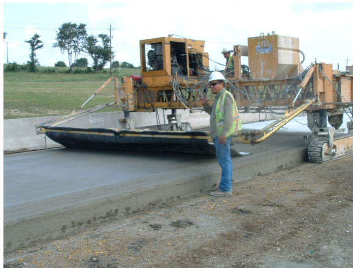
Figure 3.12: Carpet dragging, tining, and spraying curing compound
