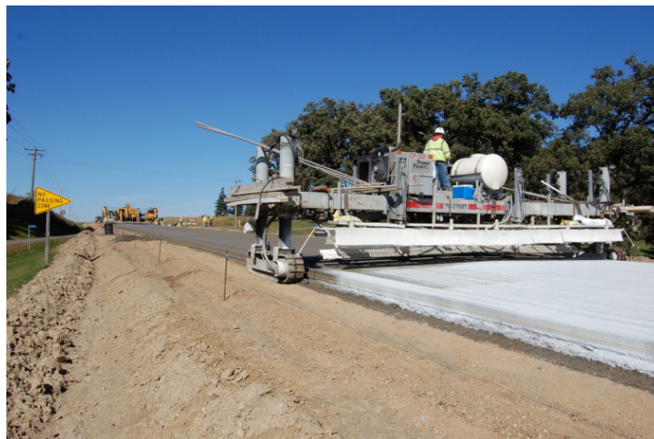
Figure 7.11: Curing compound being promptly applied following paving operation
