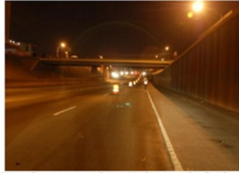
Sounding approaching N. Oregon St. Bridge (Westbound direction)
