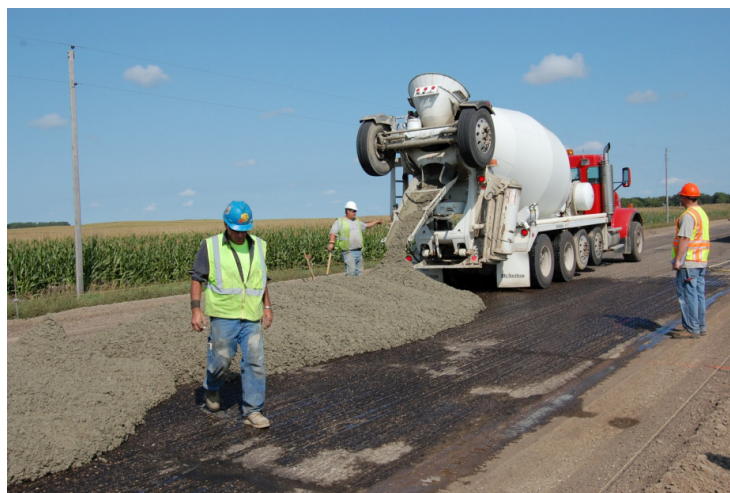
Figure 7.6: Wetted surface and dried surface
