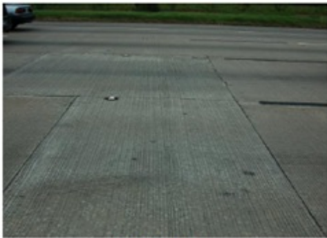
PCC Patches 1989-1990 Experimental sections (EB)
