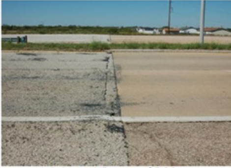
Joint at NB start of BCO
