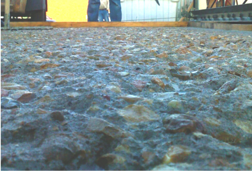
Figure 7.4: A shot blasted existing concrete pavement
