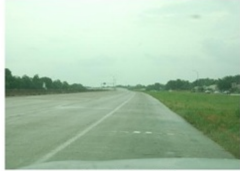
General view (NB)
