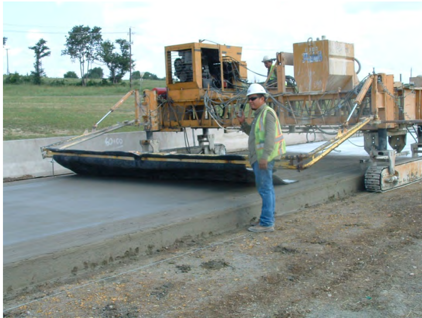
Figure 8.12: Carpet dragging, tining, and spraying curing compound
