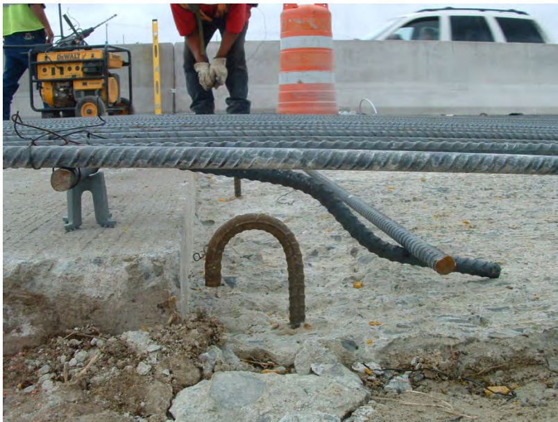
Figure 8.8: Transition reinforcement detail close-up
