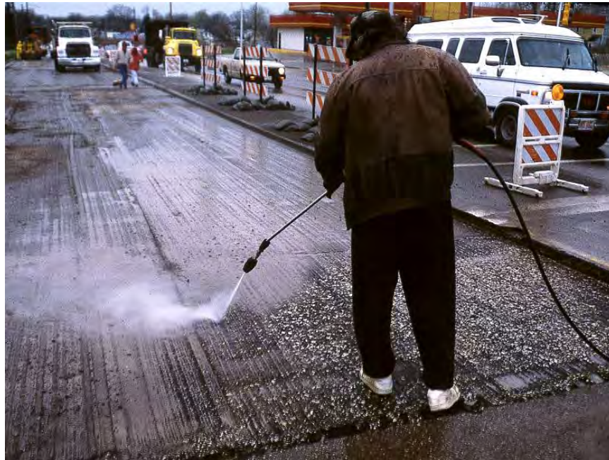
Figure 5.2: Cleaning the surface with hydrocleaning equipment
