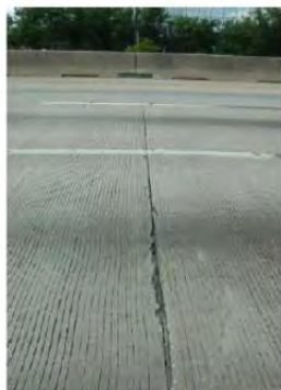
Joint damage
