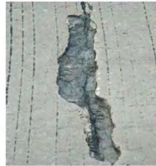
Fibers seen in spall
