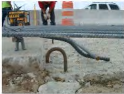
Close-Up of Reinforcement at Transition
