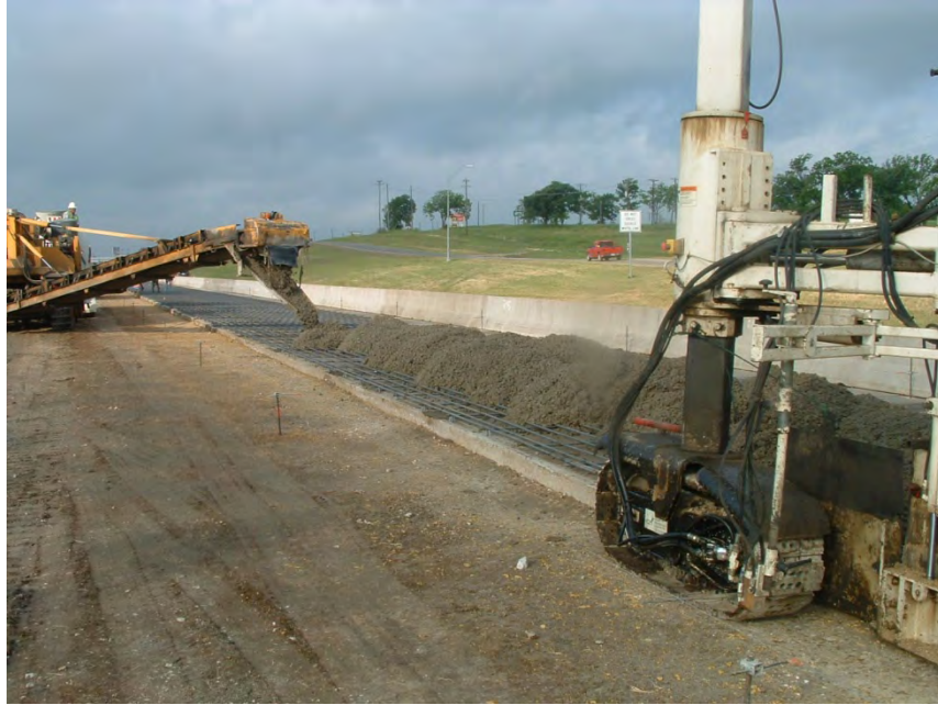
Figure 8.10: Concrete too far ahead of the paving machine
