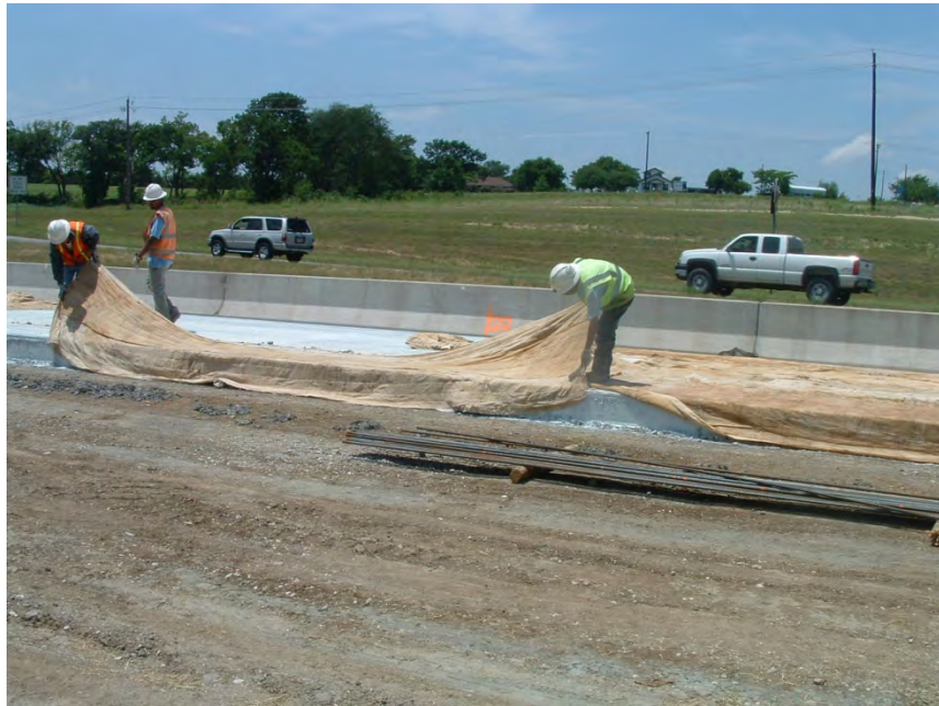
Figure 8.13: Laying down burlaps
