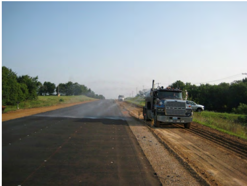
Figure 5.1: Cooling down the prepared surface before placement
