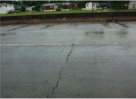
Wide transverse crack
