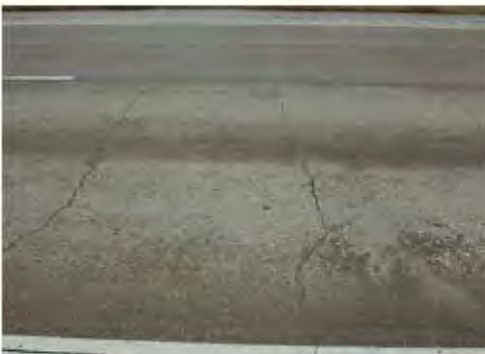
Picture 3 Transverse cracks
