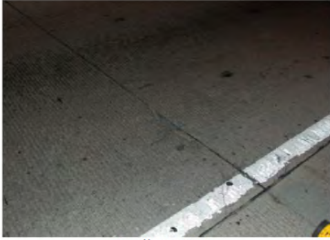
Spall at joint
