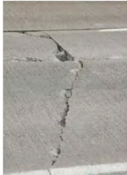
Wide crack and punchout
