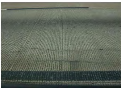
Longitudinal cracks Westbound
