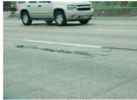
AC Patch, longitudinal cracks
