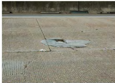
AC patch with failure
