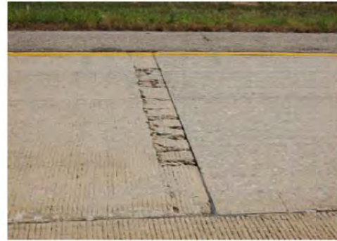
Punchout at joint (SB inside lane)
