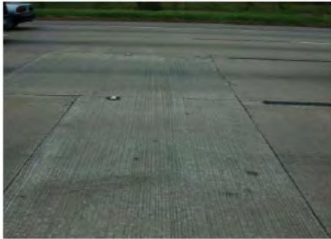
PCC Patches 1989-1990 Experimental sections (EB)
