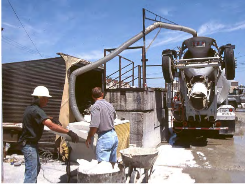
Figure 5.3: Blowing the fiber into the mixing truck
