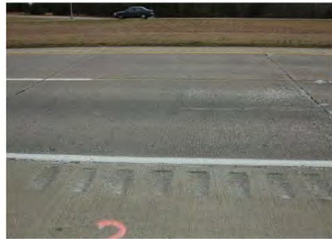
JCP slab in good condition
