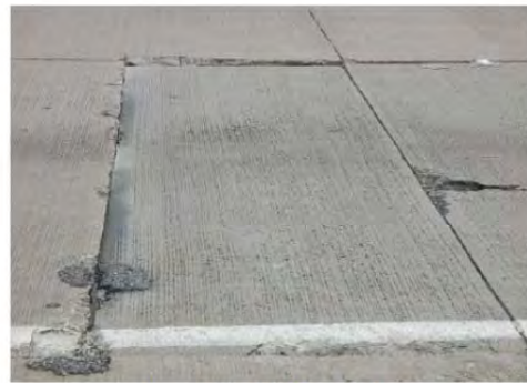
Damaged PCC patch
