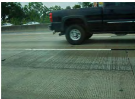
PCC patch with spall
