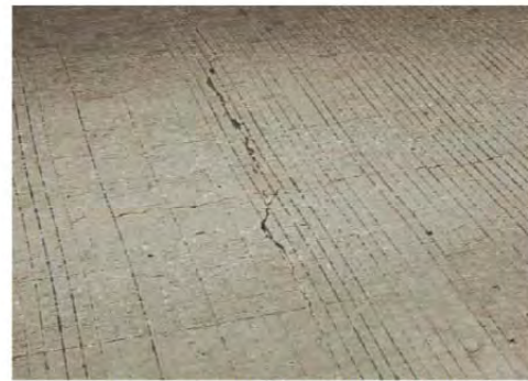
Transverse and longitudinal cracks
