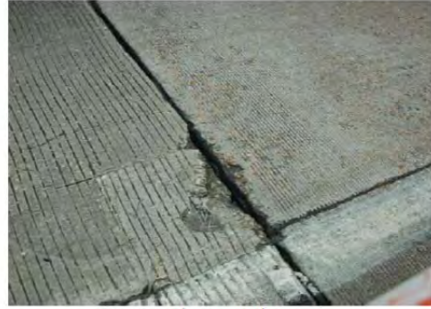
Corner damaged repair
