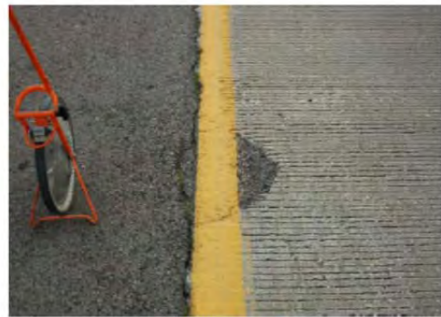
Small AC patch 1989-1990 Experimental sections (EB)
