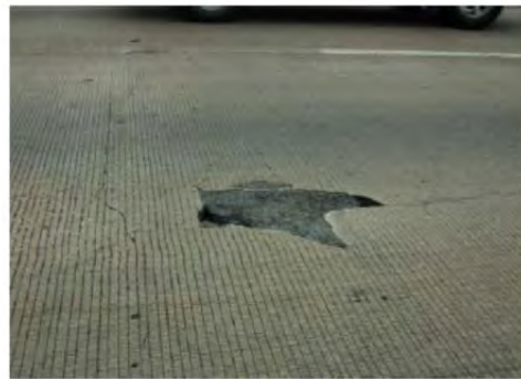
AC patch, longitudinal and transverse cracks
