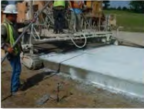
Spraying Curing Compound
