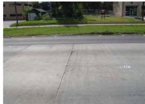
Patch with spall
