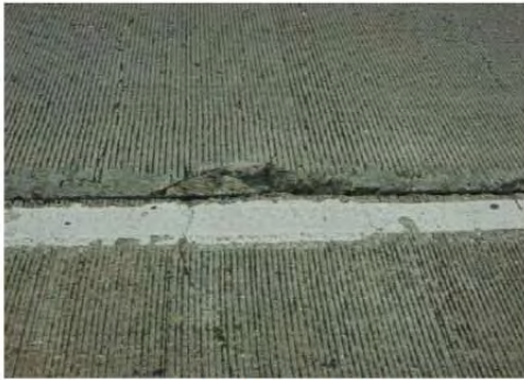
Longitudinal joint damage
