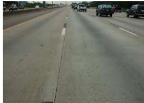
Longitudinal crack 1989-1990 Experimental sections (EB)
