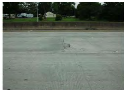
Patch with Failure
