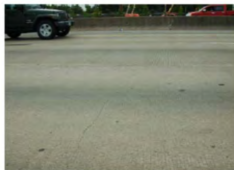
Transverse cracks
