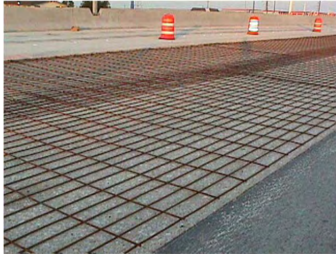
Figure 3.2: Steel placed directly on top of substrate
