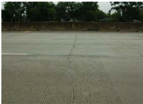
Transverse cracks
