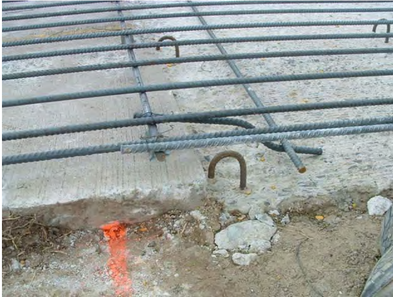
Figure 8.7: Transition reinforcement detail
