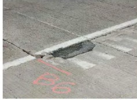
Areas to be repaired prior to BCO placement marked with spray paint
