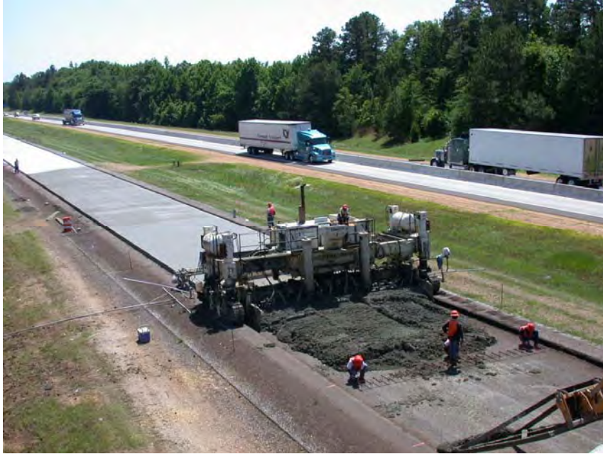
Figure 5.5: Prompt curing following the paver
