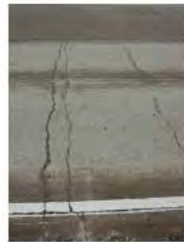
Picture 4 Area of potential punchout (RM 51 + 214 ft)
