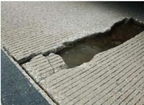
Punchout 1989-1990 Experimental sections (EB)
