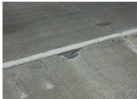
Shoulder joint damage
