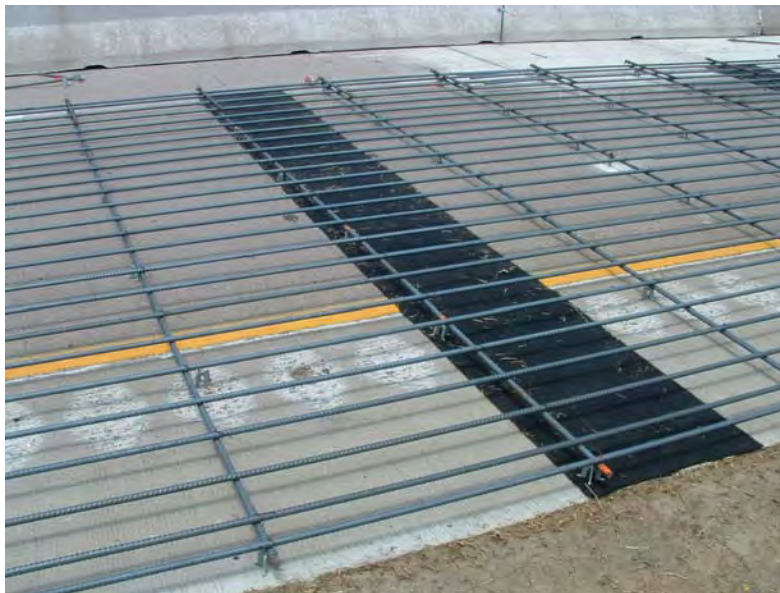
Figure 8.4: Prepared surface prior to the yellow stripe removal
