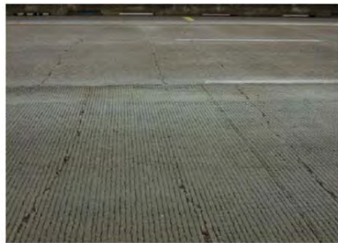
Closely spaced transverse cracks
