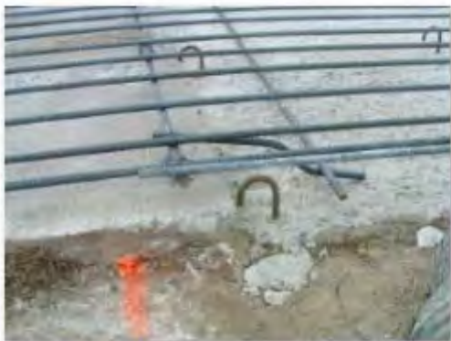
Reinforcement at Transition
