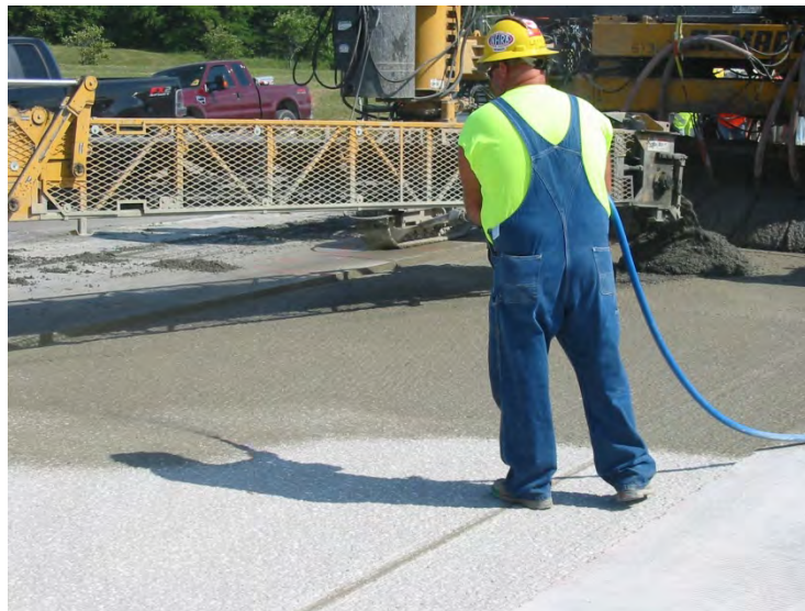
Figure 3.3: Spraying grout immediately ahead of paver
