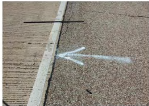
Delaminated area (edge of lane)
