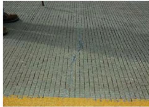
Small spalls 1989-1990 Experimental sections (EB)
