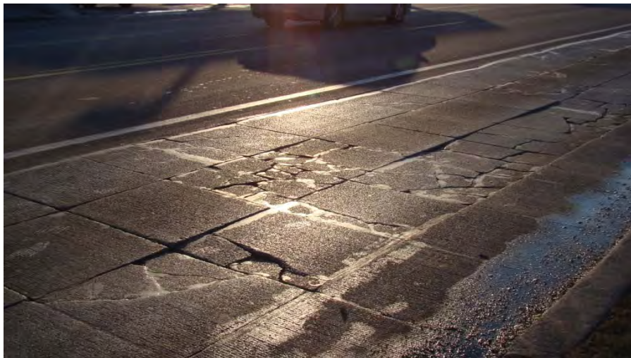
Figure 5.4: Failed joints in wheel path
