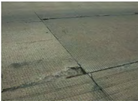
Large spall and patch
