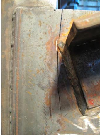
Figure 7.69: Typical Z Frame Double Angle Fatigue Crack (ZF\_DA\_2)
