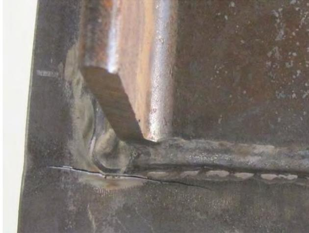
*Figure 4.58: Double Angle Connection Fatigue Crack (Gusset Plate)*
