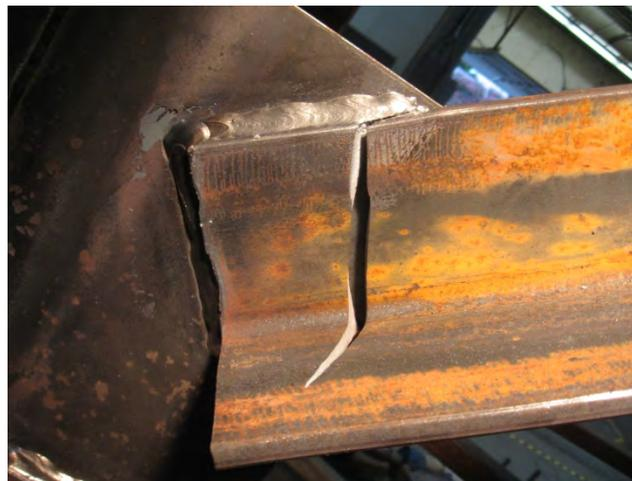
Figure 7.53: Fatigue Crack in Tension Diagonal (KF\_7)
