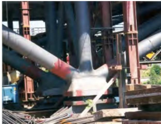
*Figure 2.26: Large Cast Steel Bearing in Tubular Arch Bridge [FHA 2001]*
