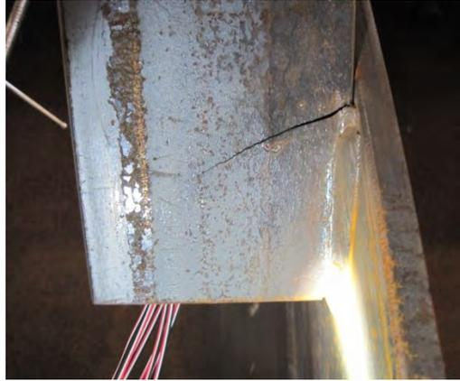
Figure 7.44: K Frame Fatigue Crack in Tension Diagonal (KF\_2)
