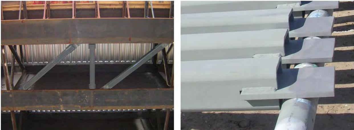
*Figure 2.27: Tubular Bracing Retrofit of Curved Steel Bridge in Wichita Falls, TX with Close-up of Connections [Turco 2009]*
