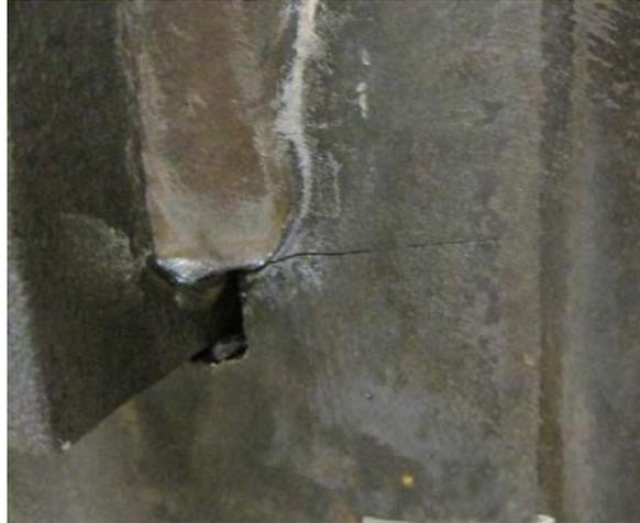
*Figure 4.52: Knife-Plate Connection Fatigue Crack (Torch-Cut Slots)*
