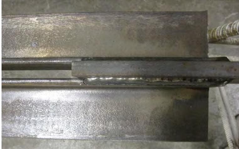
*Figure 4.53: Double Angle Detail*
