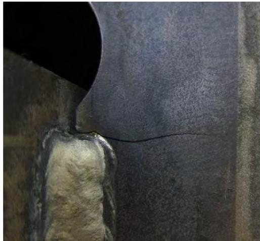
Figure 4.51: Knife-Plate Connection Fatigue Crack (Stress Relief Hole)
