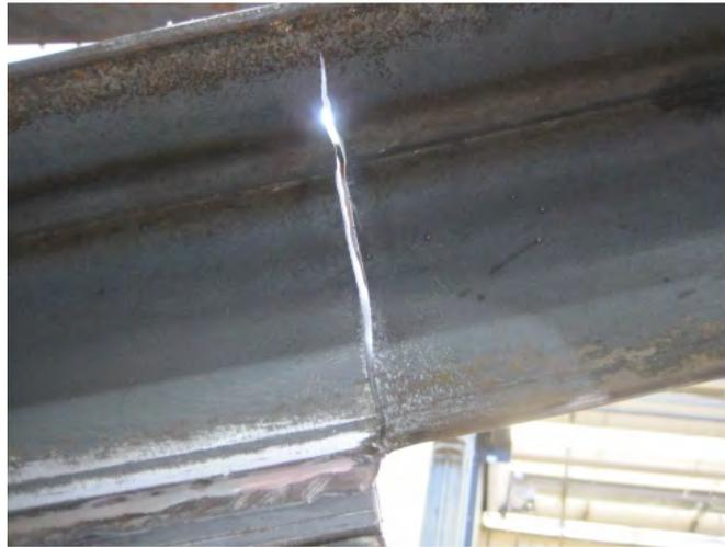
*Figure 7.35: Typical Unequal Leg X Frame Fatigue Crack (XF\_UL\_1,2)*
