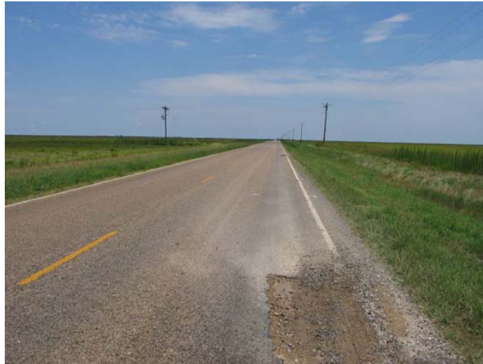
Figure 2.45: Damage on FM 97 Resulting from Windfarm Development
