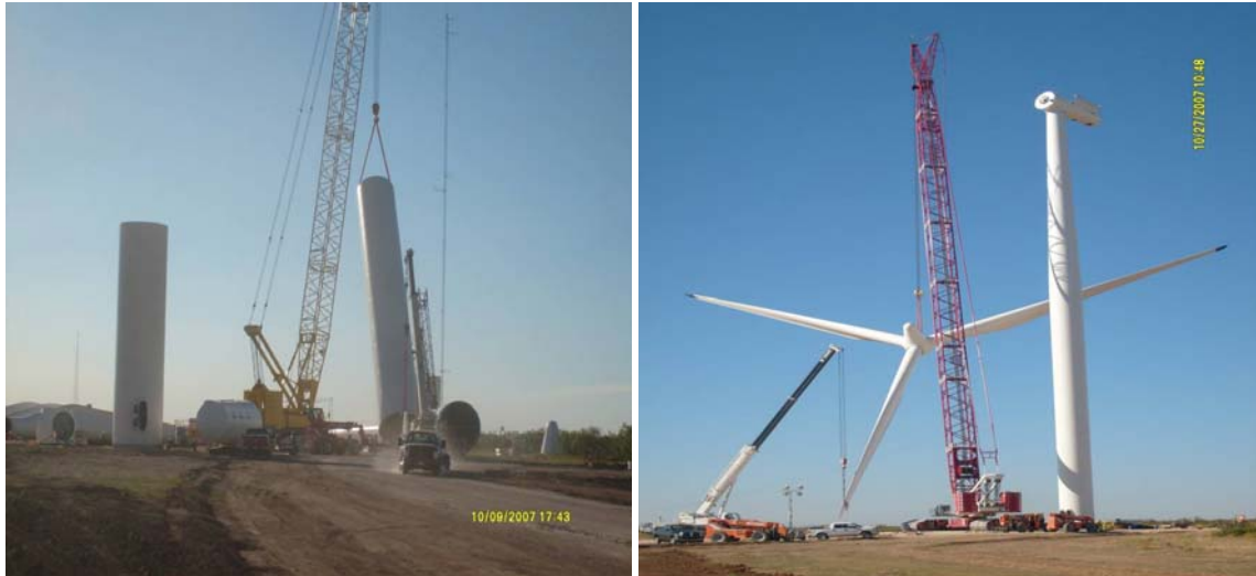
Figure 2.44: Assembly of a Wind Mill
