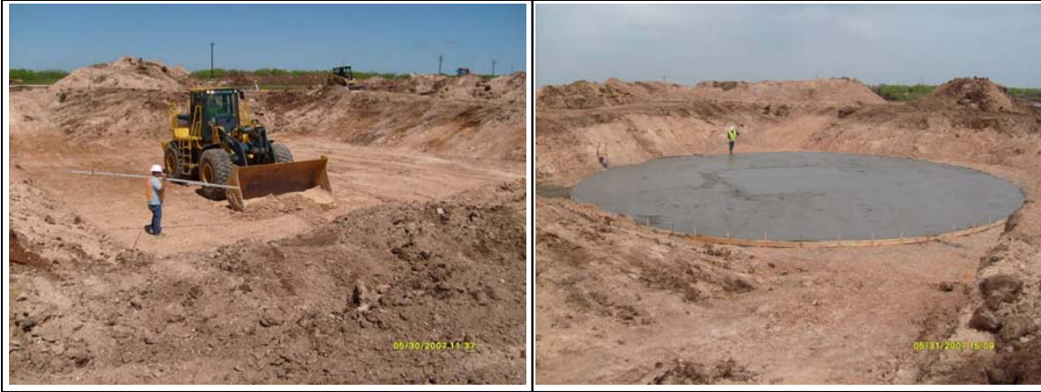
Figure 2.42: Site Preparation (Excavation and Mud Mat)
