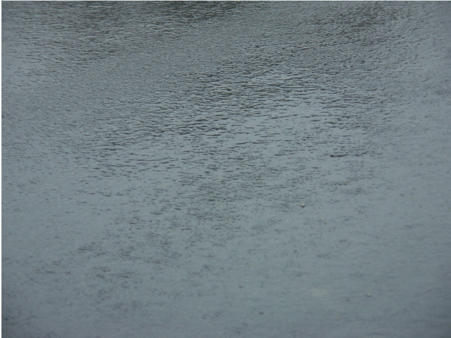
Figure A.7: CAM surface irregularities apparent on FM 60 in Bryan
