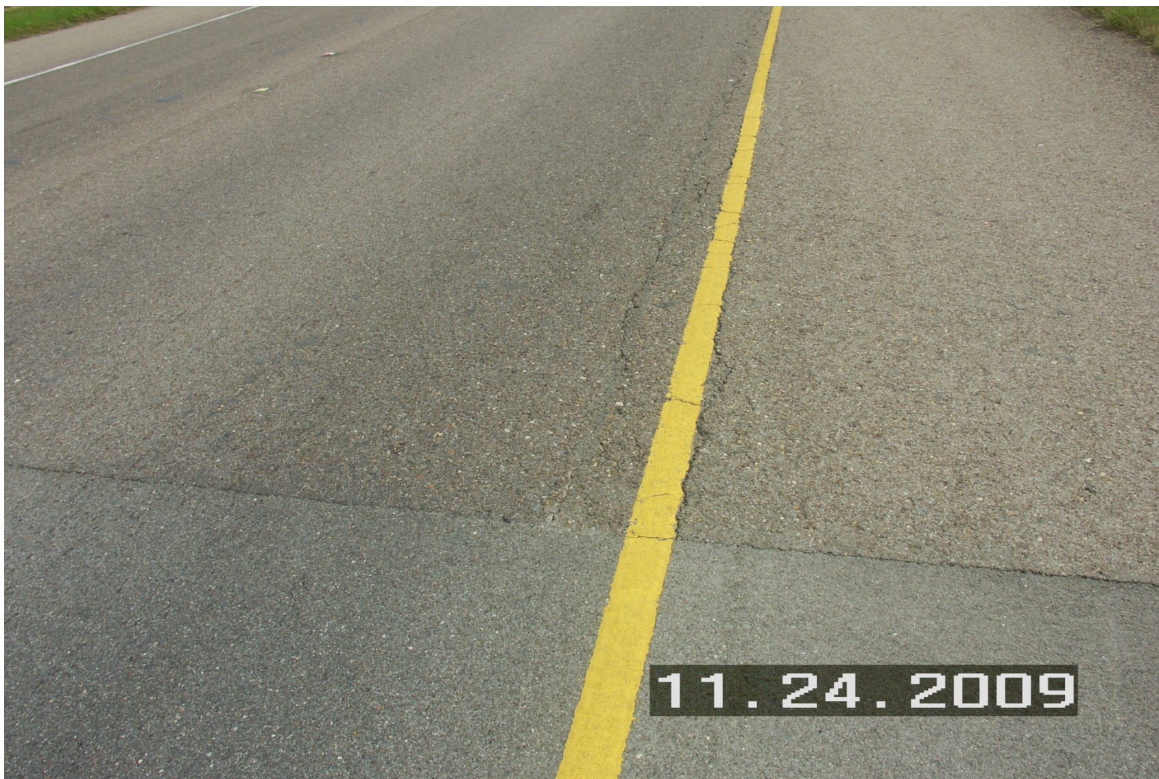
Figure A.3: Cracking on Loop 20
