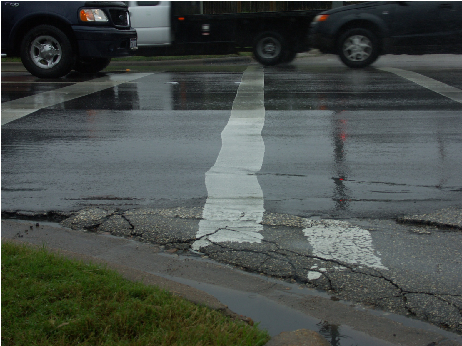
Figure A.11: CAM shoving at an intersection on FM 2154 in Bryan
