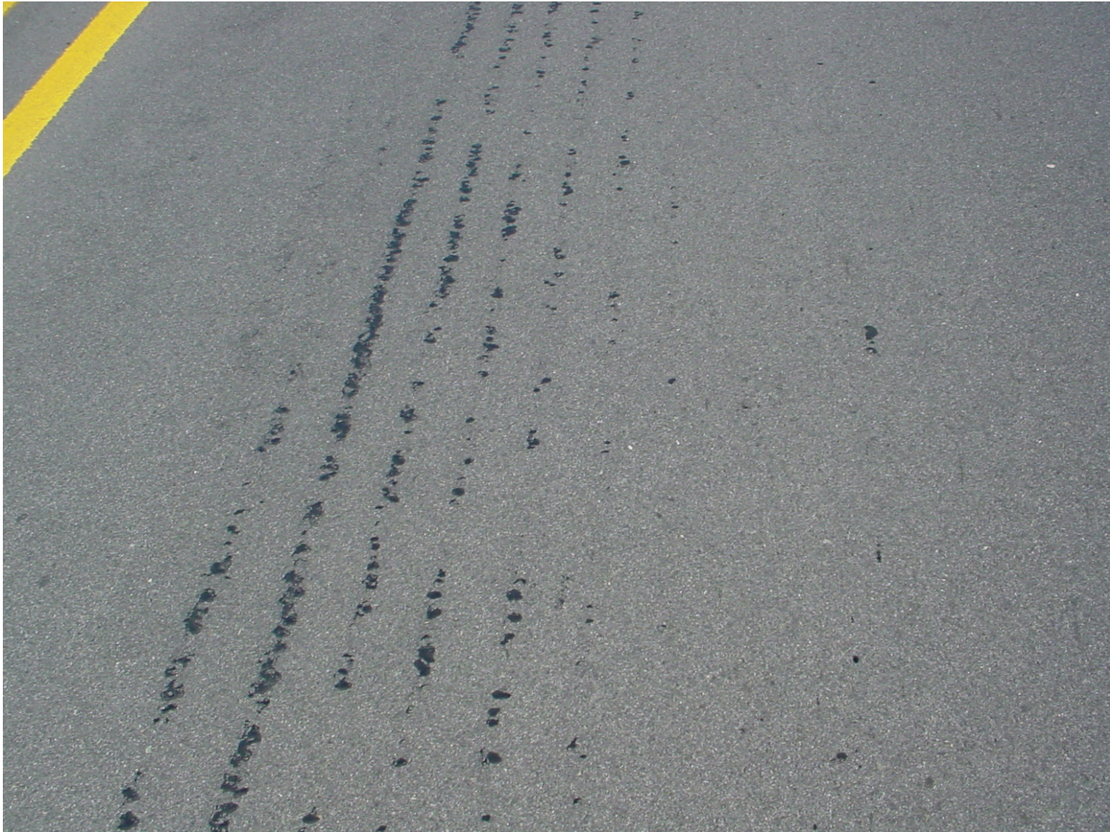
Figure A.25: Uniformity of bleeding patterns suggests tack coat striping
