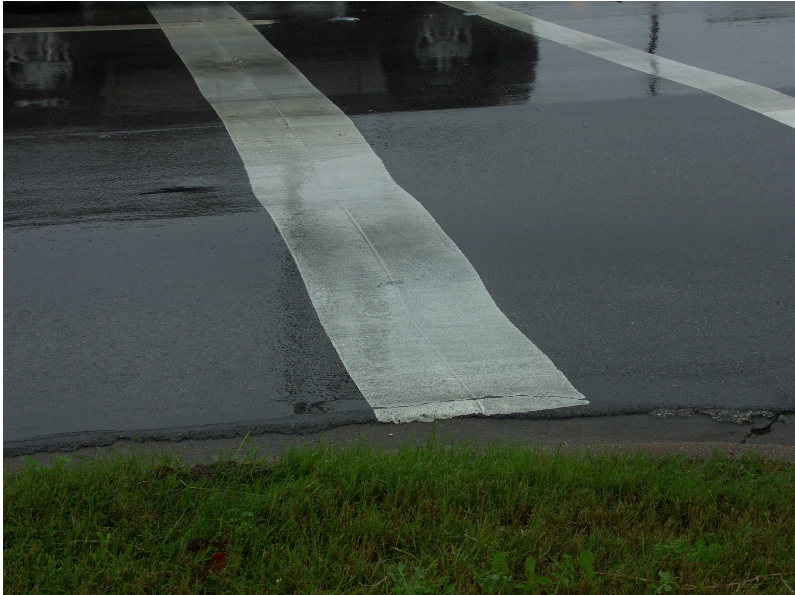
Figure A.10: CAM Rutting at an intersection on FM 2154 in Bryan
