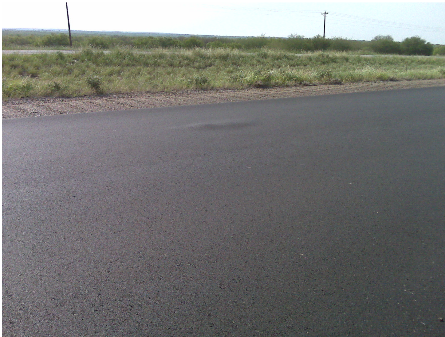
Figure A.1: CAM blistering (IH35, LaSalle, Laredo)
