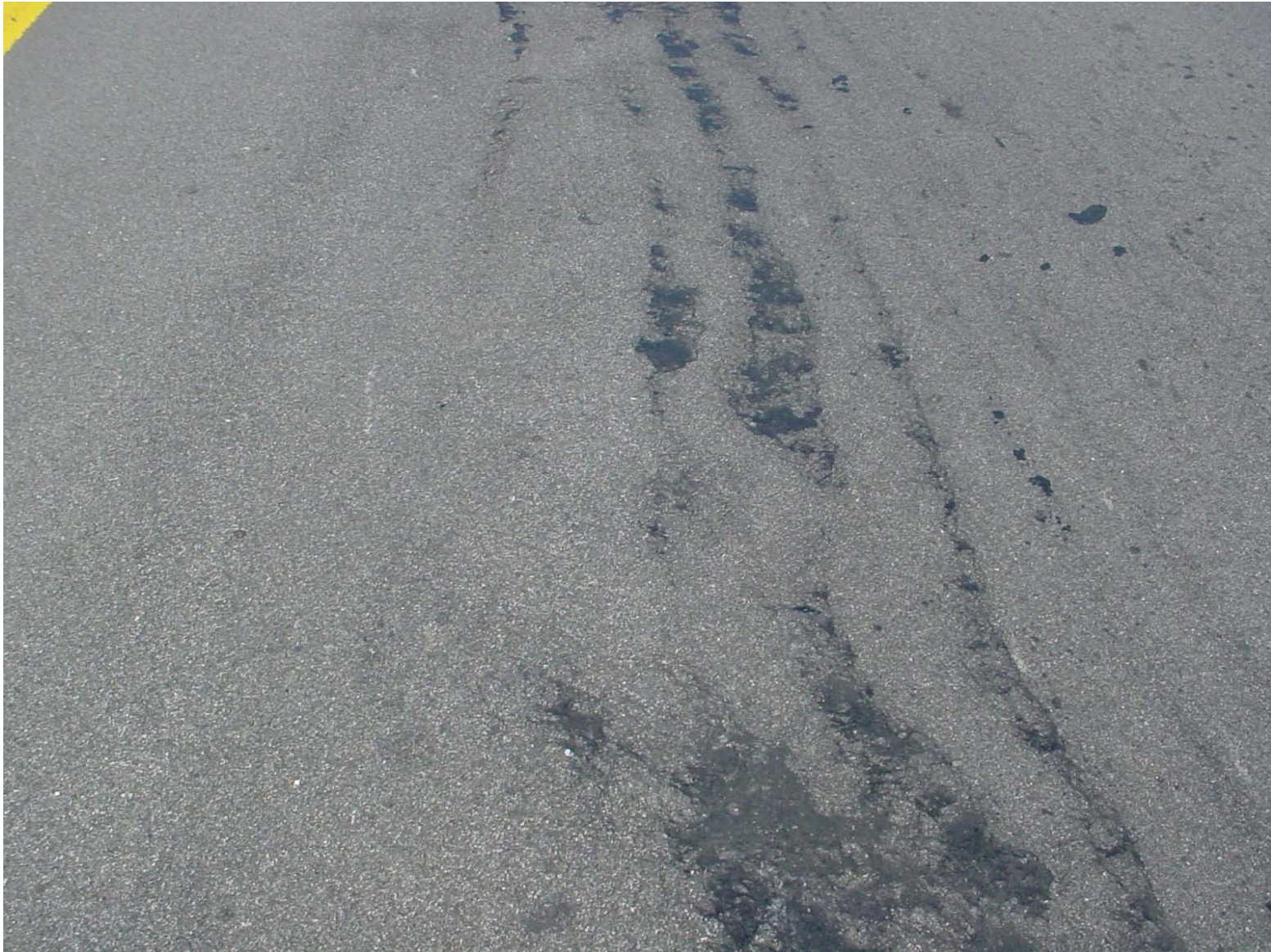
Figure A.24: Flushing of CAM paved on US 90 in Uvalde County
