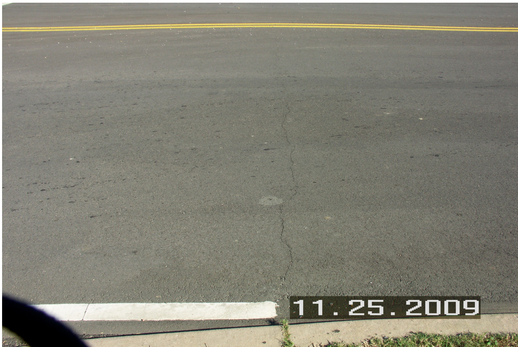
FigureA.22: Transverse cracking of CAM on US 69 in Denison
