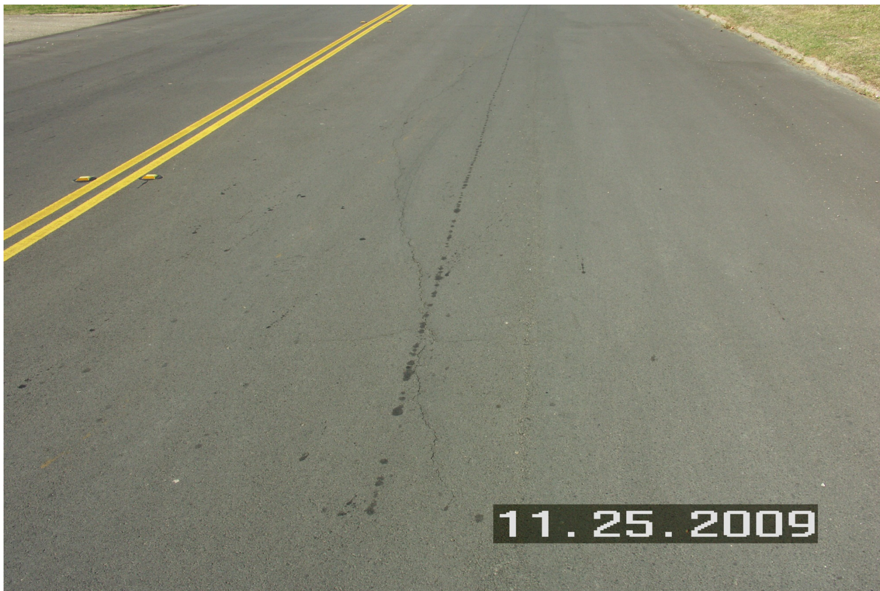
Figure A.21: Longitudinal cracking of CAM on US 69 in Denison
