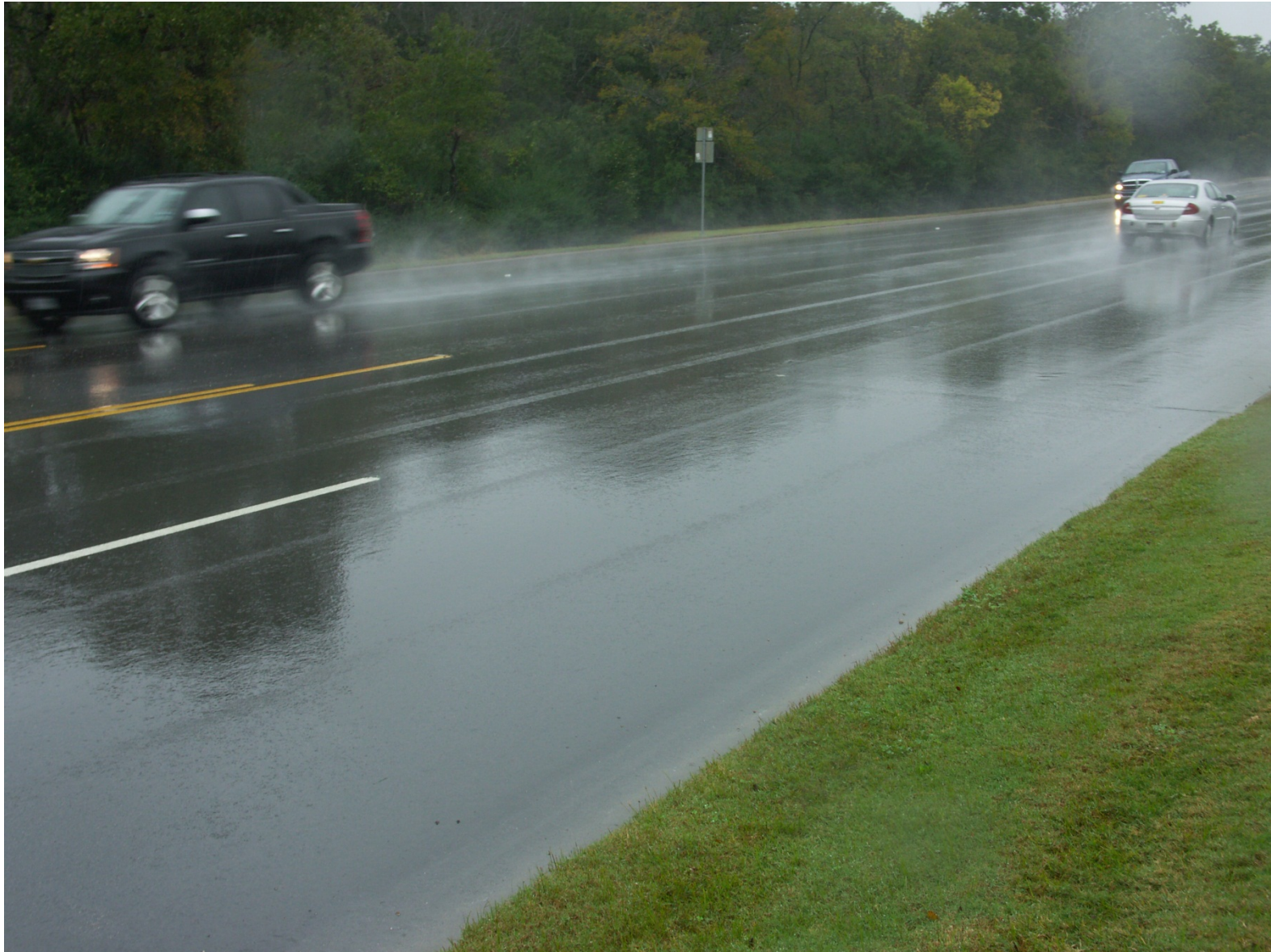
Figure A.8: Slick CAM surface and reflections on FM 60 in Bryan
