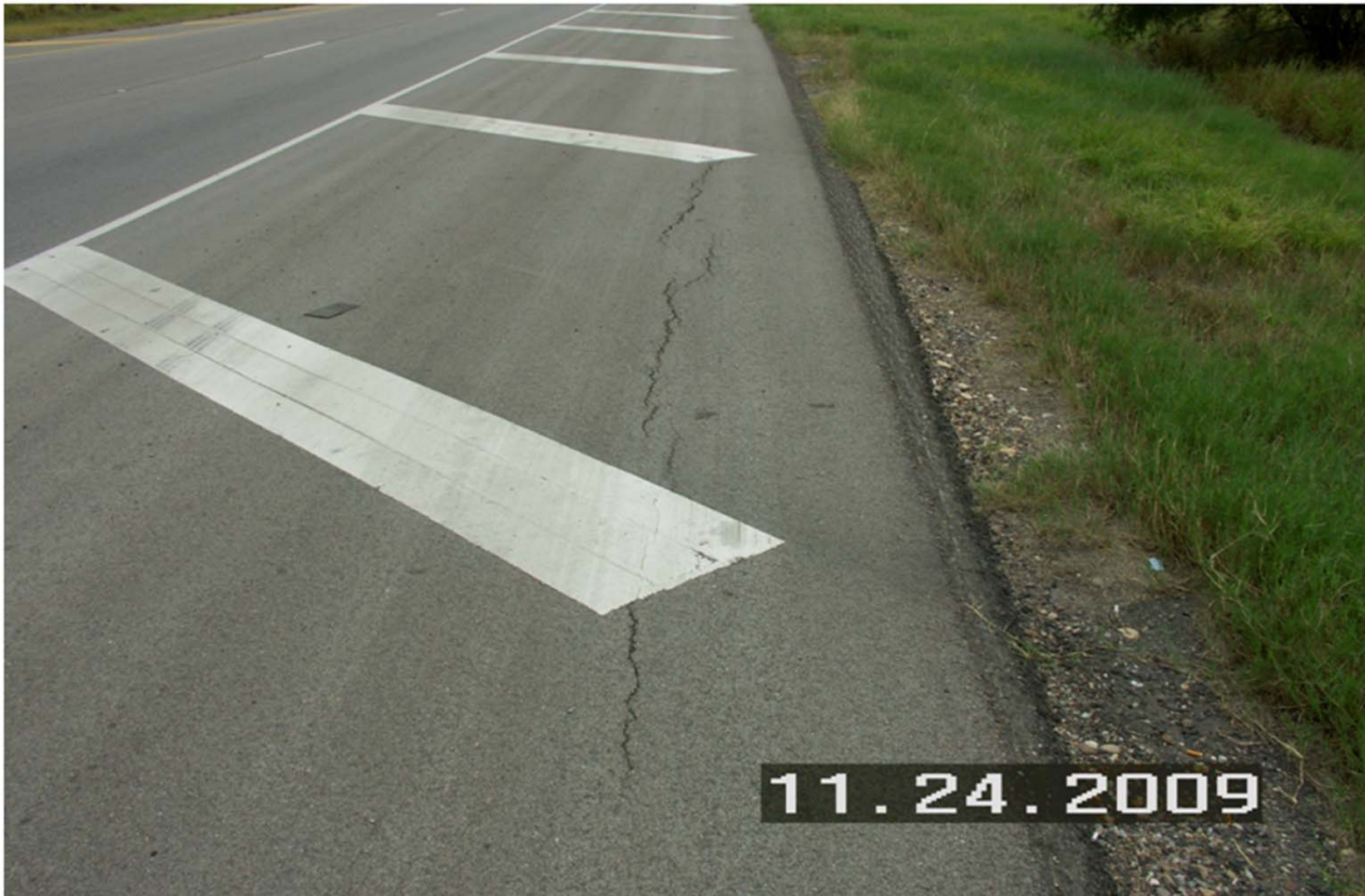
Figure A.4: Longitudinal cracking of CAM on Loop 20
