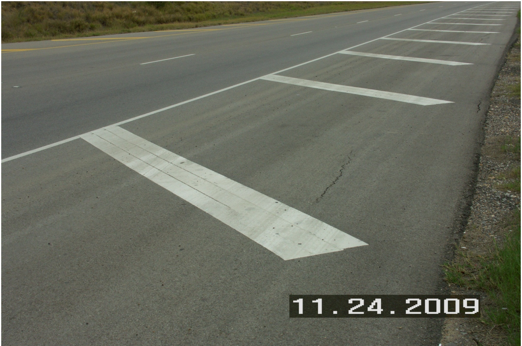
Figure A.5: Edge-related cracking on Loop 20
