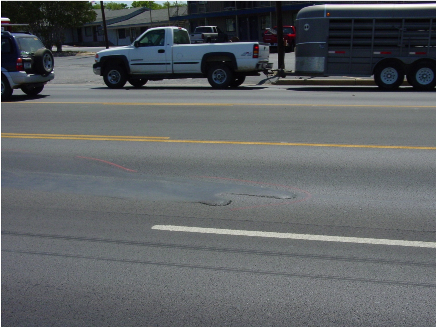
Figure A.27: Shoving and shear failure of CAM on US 281 in Burnett County, Austin
