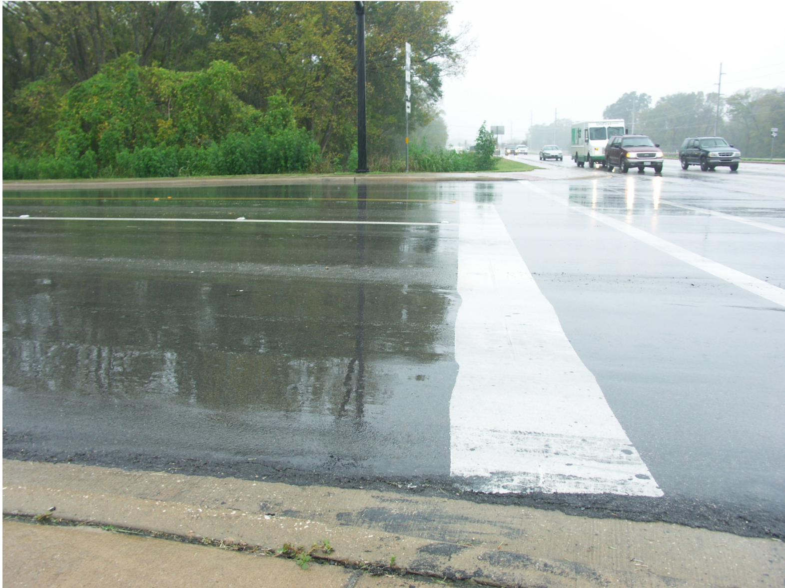
Figure A.16: Shoving of CAM at another intersection on FM 1179 in Bryan
