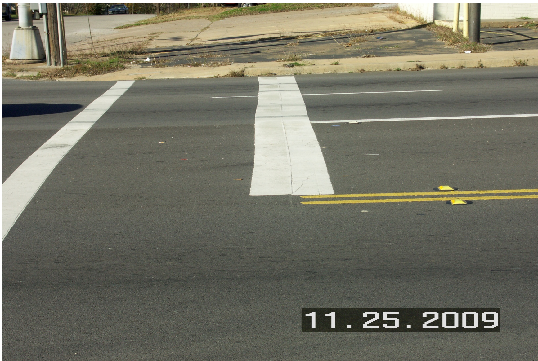
Figure A.23: Shaving of CAM at intersection on US 69 in Denison
