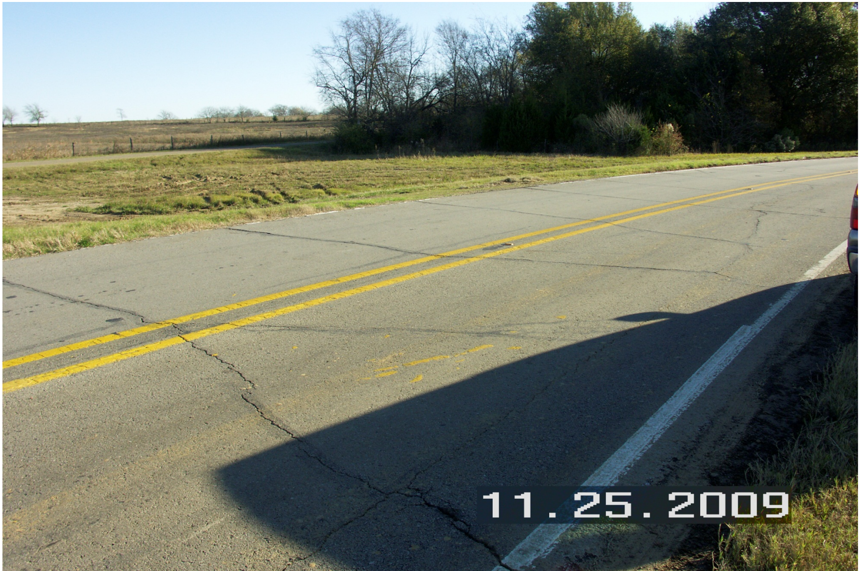
Figure A.18: Cracked surface on FM 499 overlaid with CAM (Hopkins County)
