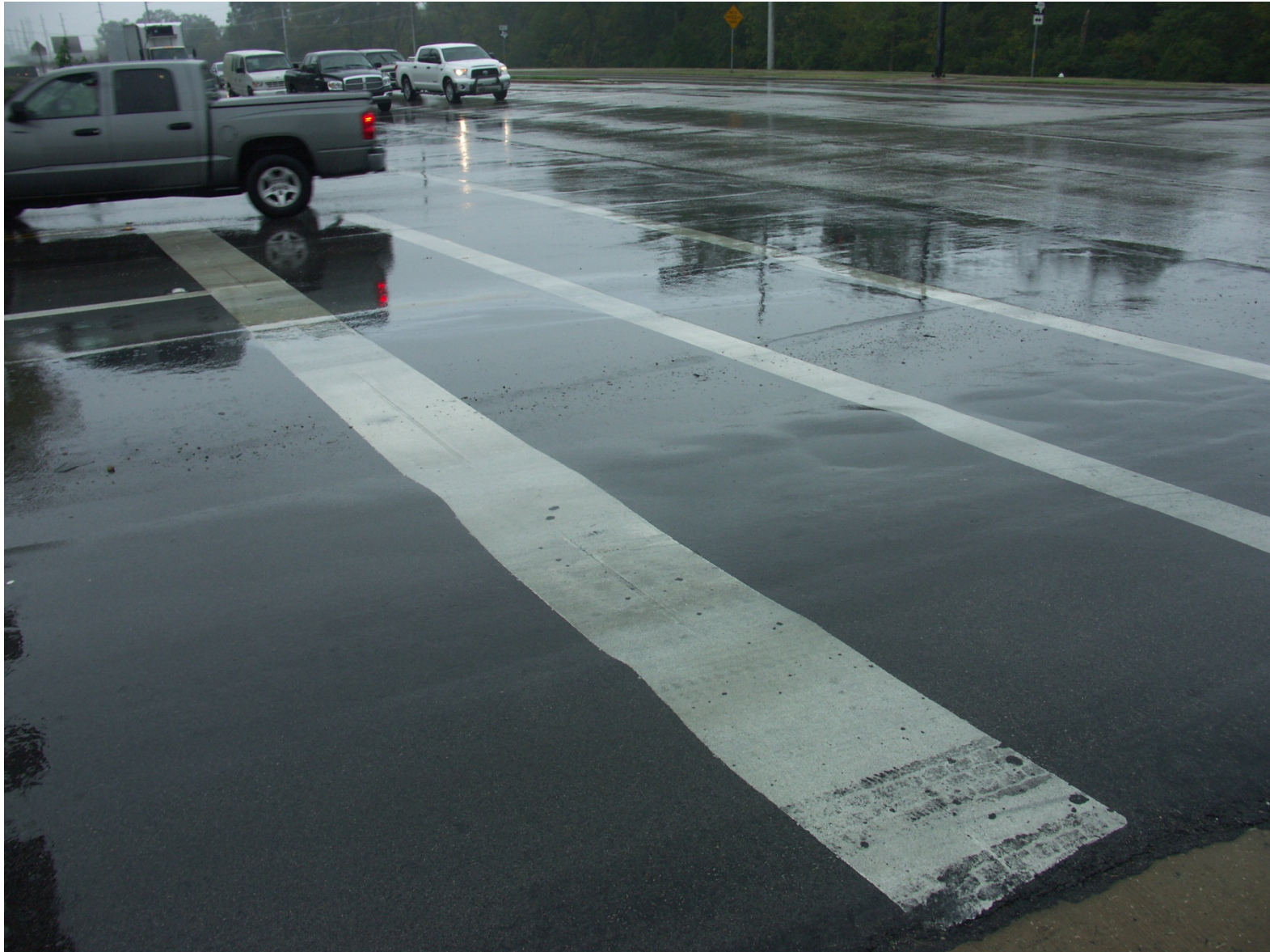
Figure A.15: Shoving of the CAM at an intersection on FM 1179 in Bryan
