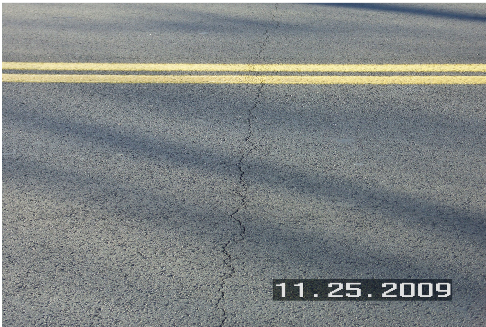
Figure A.19: Transverse reflection cracking of new CAM on FM 499 in Hopkins County
