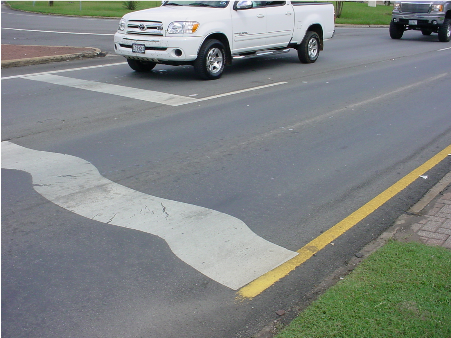
Figure A.26: Rutting of CAM on BU 59 in Angelina County, Lufkin
