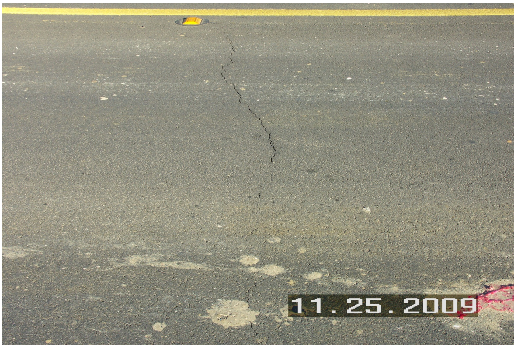
Figure A.20: More transverse reflection cracking of new CAM on FM 499 in Hopkins County
