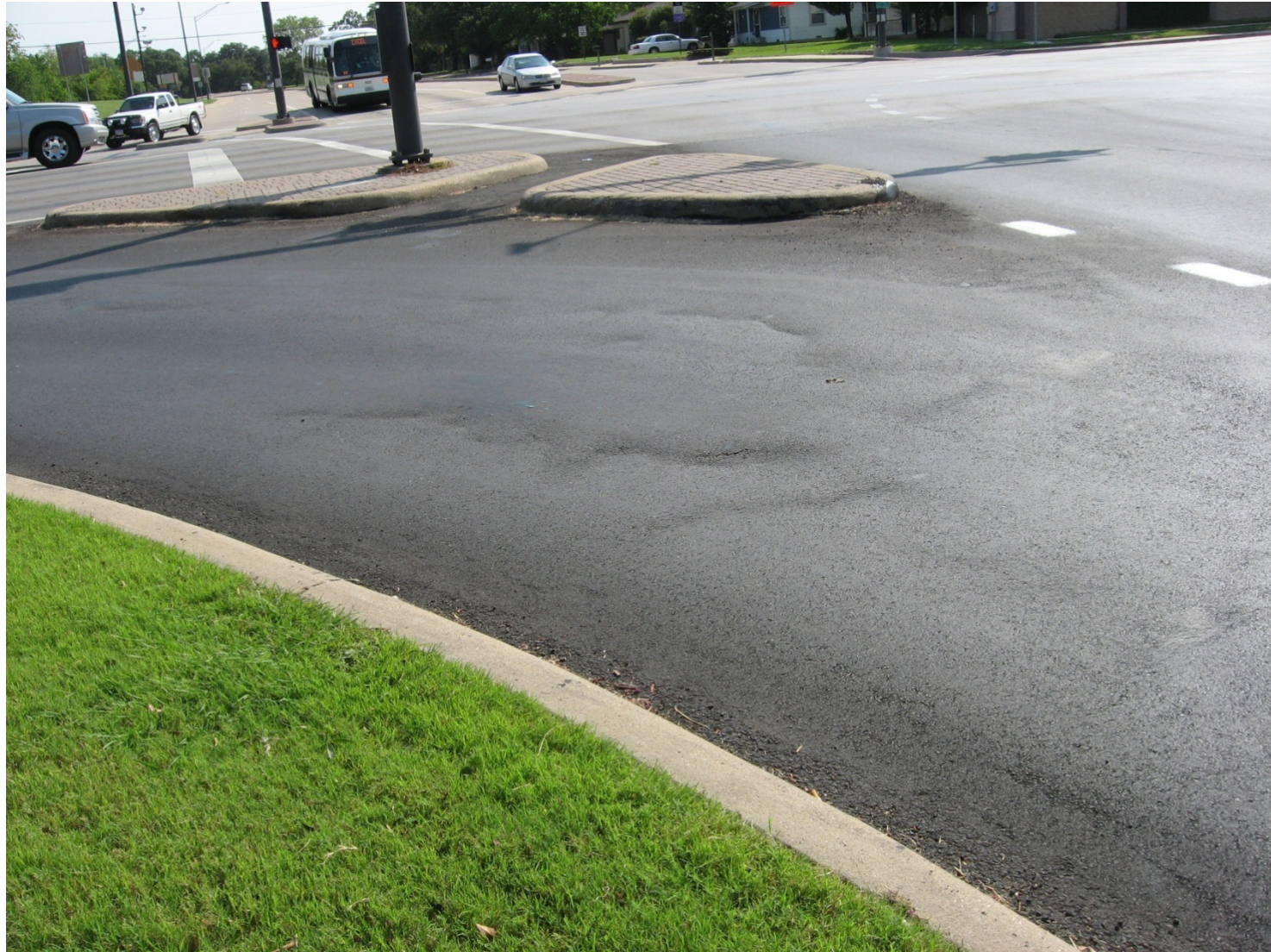
Figure A.14: Shoving of CAM on FM 2347 in Bryan
