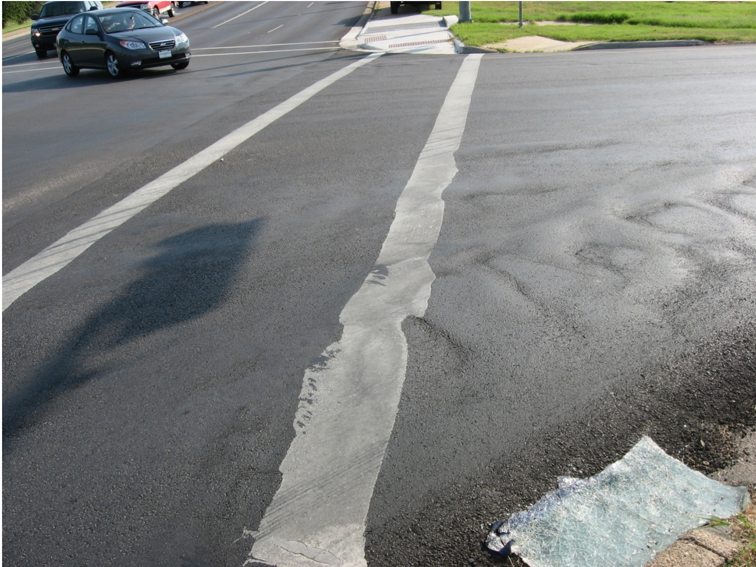
Figure A.13: Shoving of CAM on FM 1179 in Bryan
