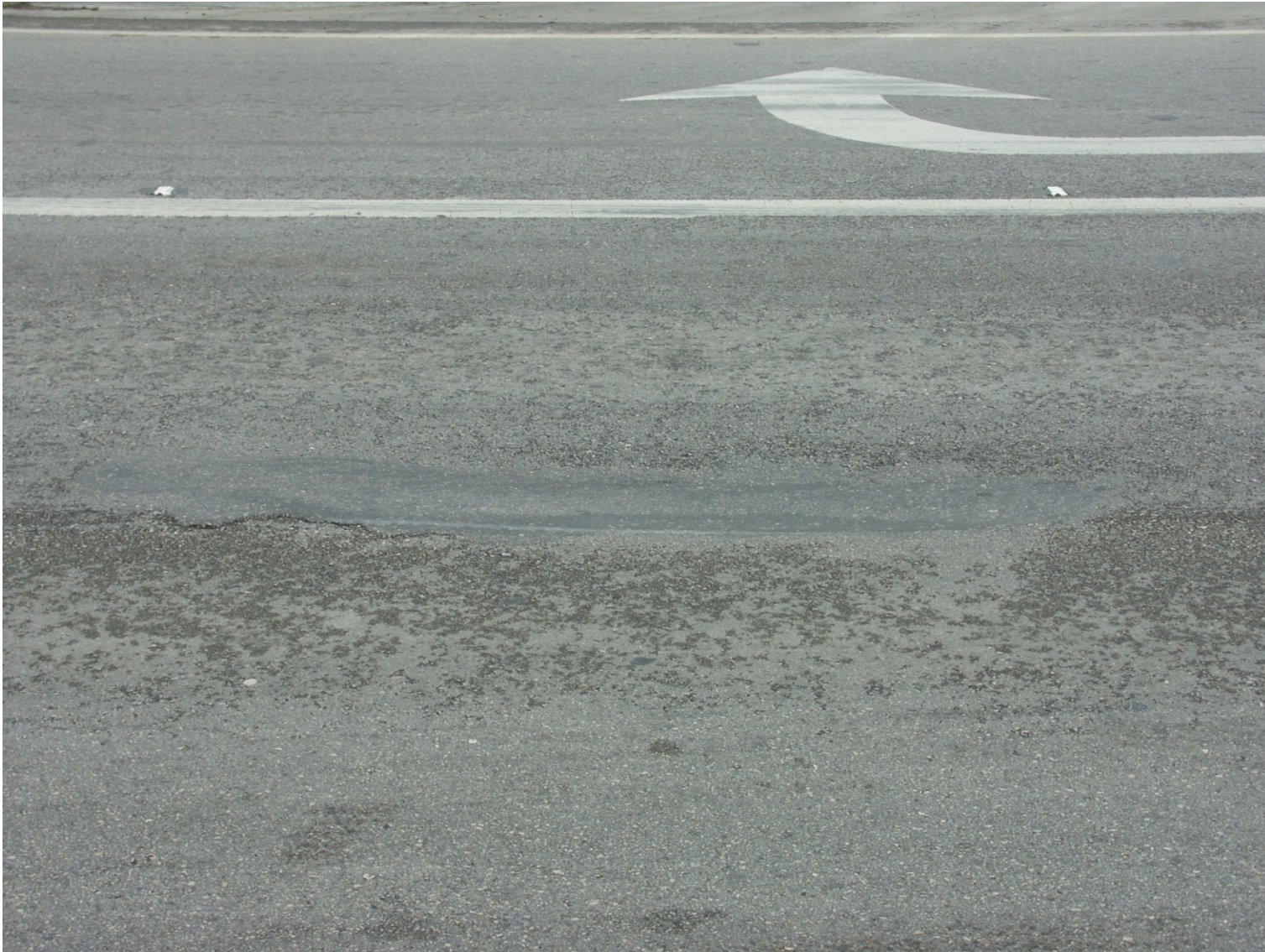
Figure A.6: Shoving of CAM underlayer at intersection between SH 21 and SH 6 in Bryan
