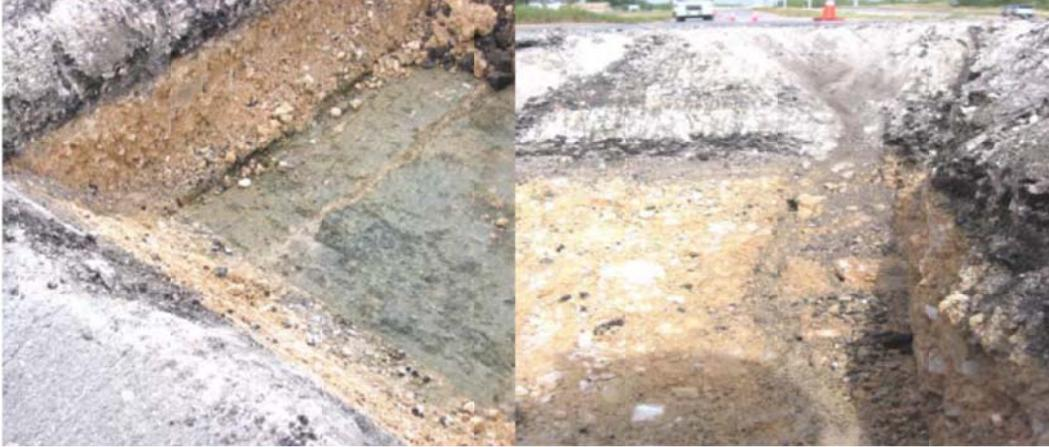
Figure 2.9: Reflective shrinkage cracking seen in test pit
