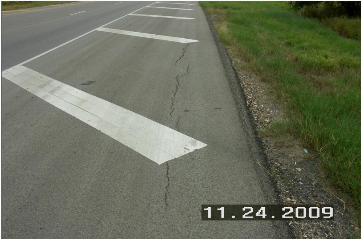
*Figure 8.3: Cracking along pavement shoulder in CAM section on Loop 20, Laredo*
