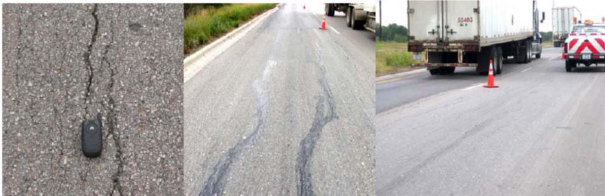
*Figure 2.8: Shrinkage cracking distress on FM 734*
