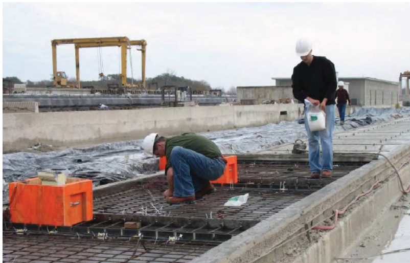
Figure 3.2: Casting Instrumented Panels at Plant A, February 2009
