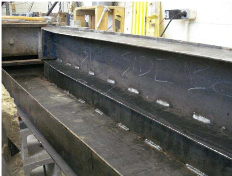
Figure C.5: Fitting of steel formwork.
