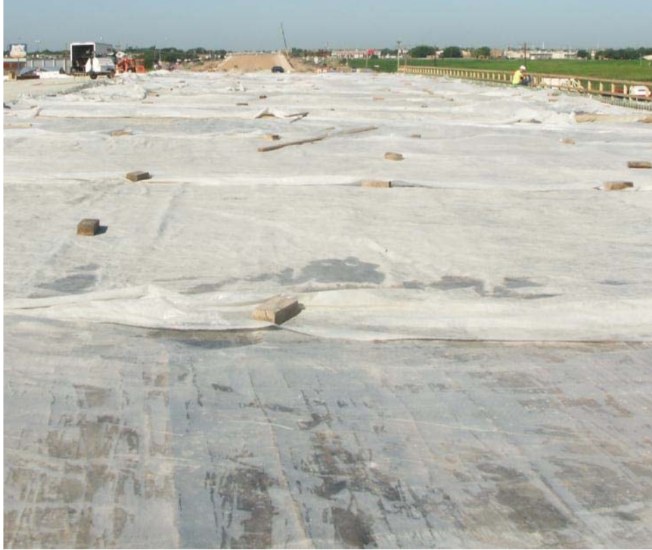
Figure 7.36: Curing method for Lubbock bridge deck.
