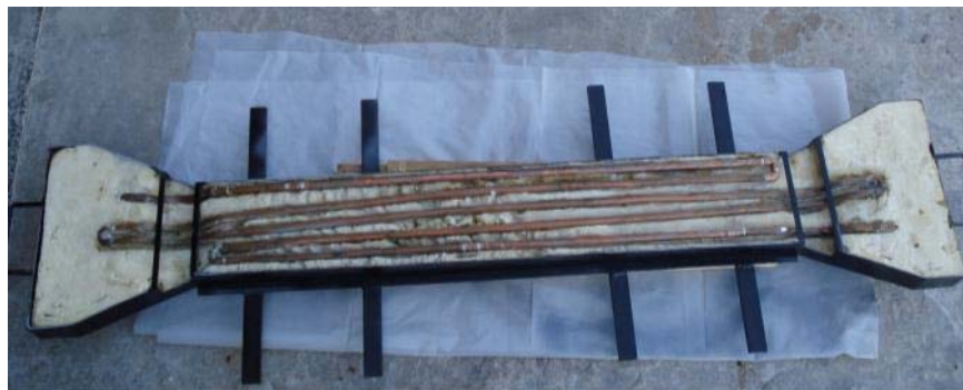
Figure C.10: Bottom formwork before application of flashing.
