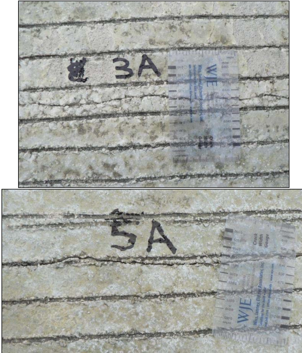
Figure 7.7: Crack-like lines on San Antonio bridge deck.
