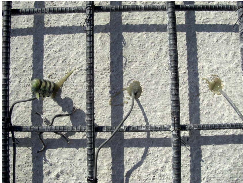
Figure 7.42: Completed bridge deck instrumentation.
