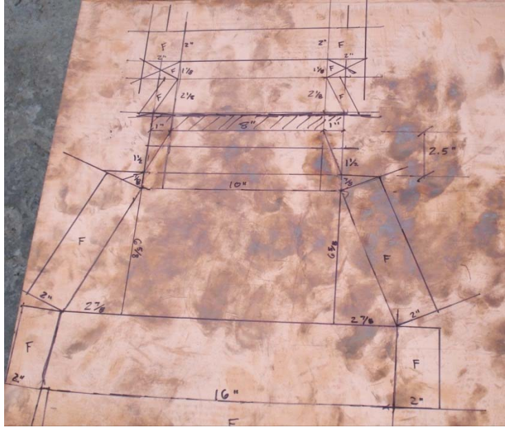
Figure C.6: Measurements for cutting new flashing with fold-over flaps.
