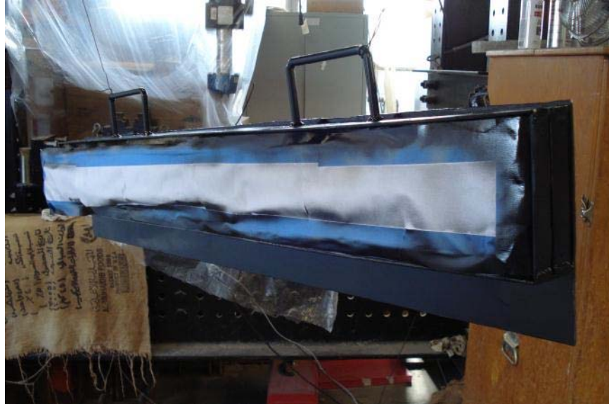
Figure C.8: Painting of steel formwork.
