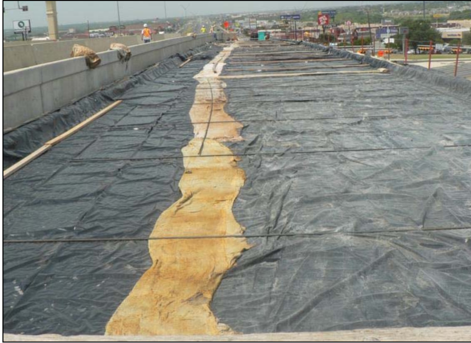
Figure 7.6: Curing method for San Antonio bridge deck.
