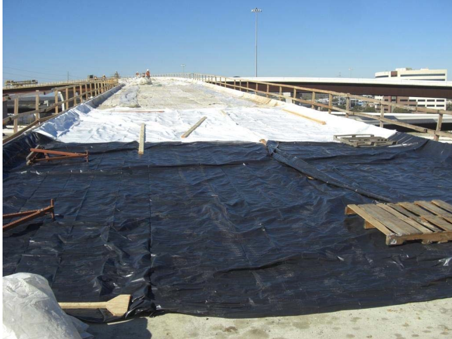
Figure 7.49: Bridge deck during removal of curing
