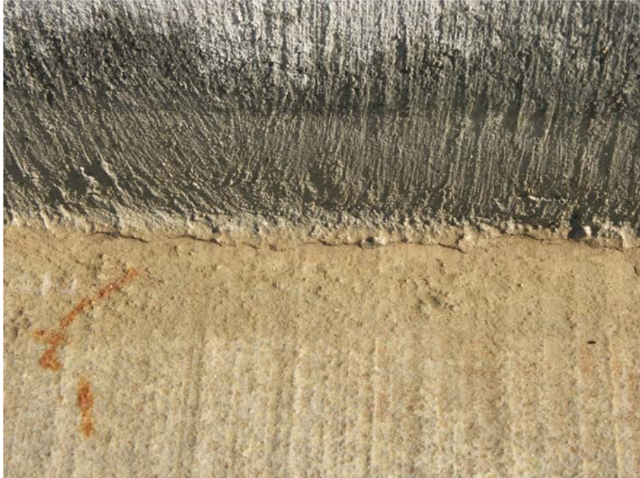
Figure 7.26: Cracking between bridge deck and sidewalk concrete.
