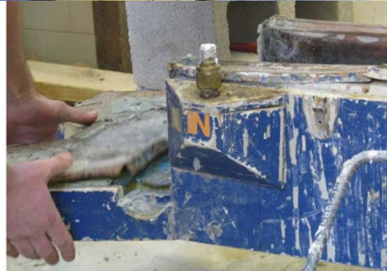
Figure C.2: Separation of copper flashing.
