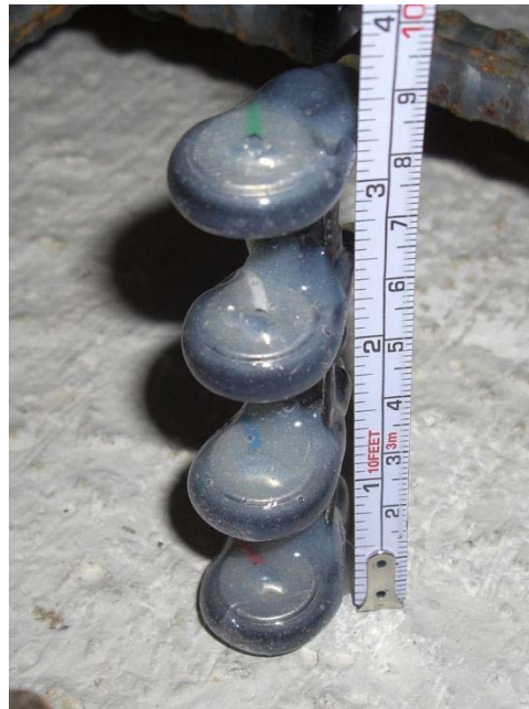
Figure 7.48: Installed temperature sensors.
