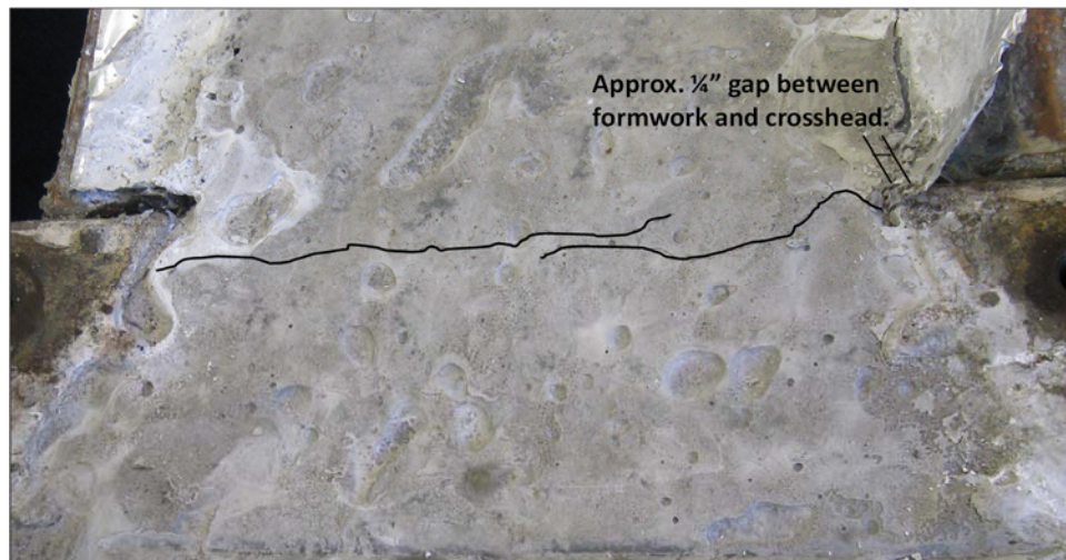
Figure C.1: Stress concentrations from formwork fatigue.
