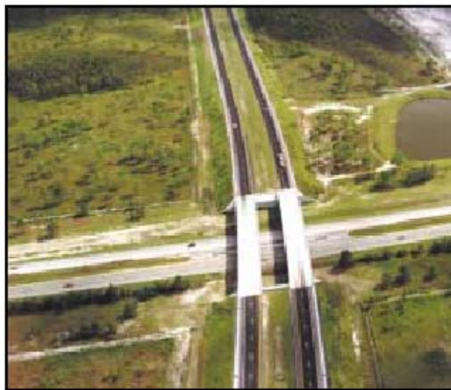
Figure B7: View of Intersection of the Turnpike and the Southern Connector
