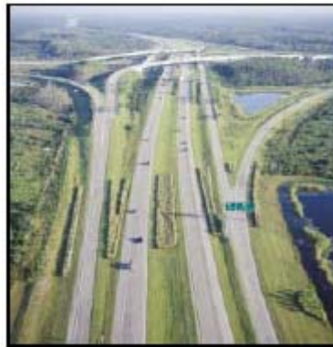
Figure B5: Aerial Photograph of Completed Southwestern Beltway
