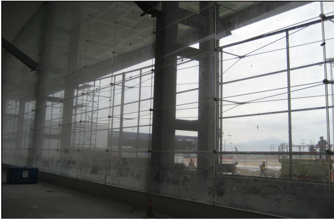
Figure 4.88: Terminal B large glass walls for natural lighting.
