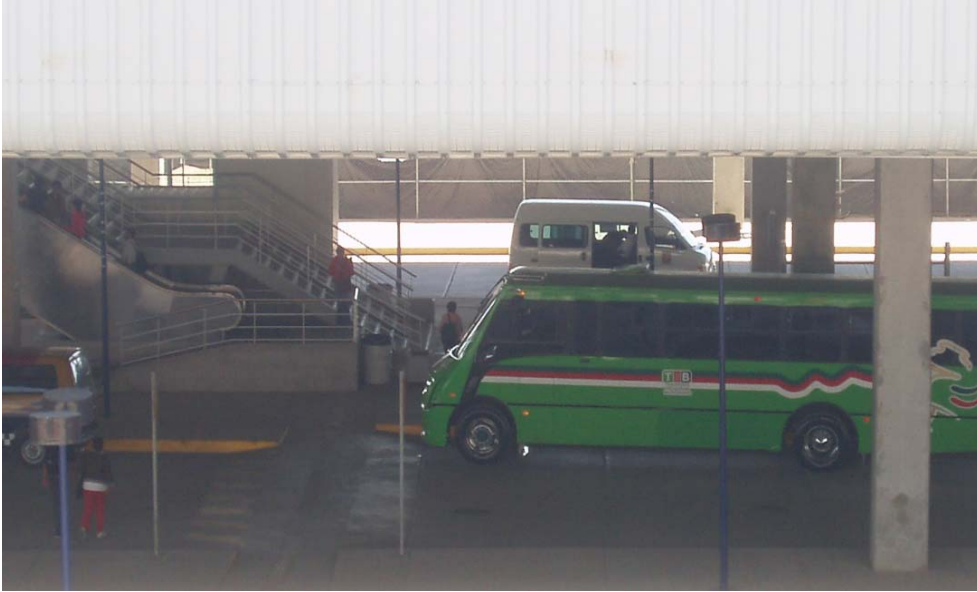
Figure 4.67: Transfer Station (Centro de Transferencia Modal, CETRAM)
