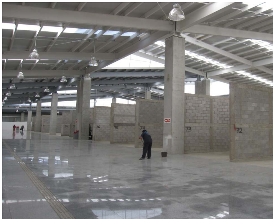
Figure 4.68: Figure: Commercial Space under Construction
