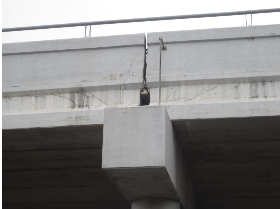
Figure 6-1: Diagonal cracks in box beams over central bent cap in bridge over IH35.
