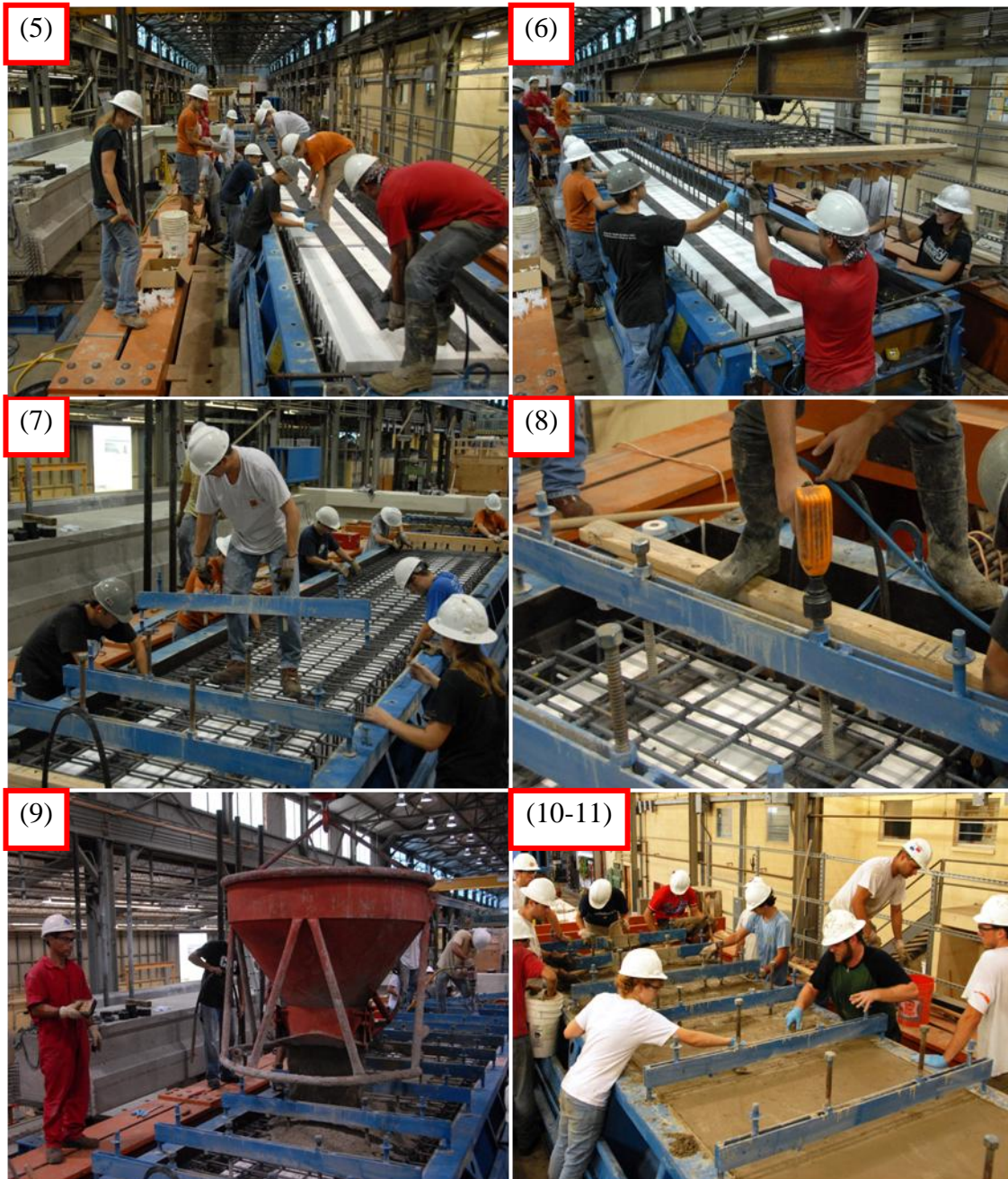
Figure 3-17: Step-by-step Box Beam fabrication process (continued)
