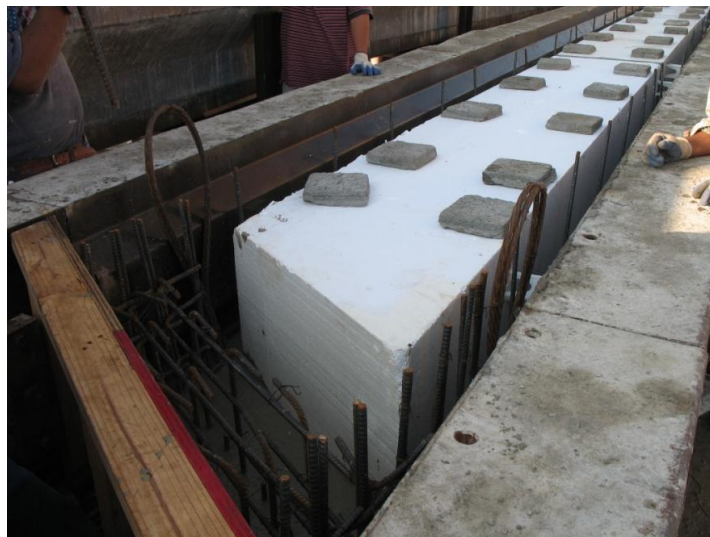
Figure 3-4: Skewed void at 30° skewed end of 4B28 Box Beam.
