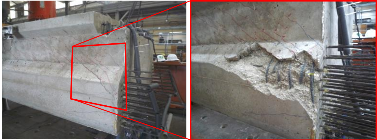
Figure 6-16: Spalling of cover at end of beam. Square end of 5B40-1 is shown.
