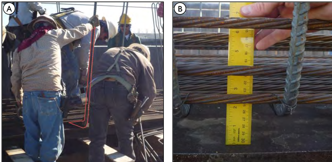
Figure 5-10: Workers using a 1.5 in. pry bar (outlined) to lift bottom strands; (B) resulting strand locations.
