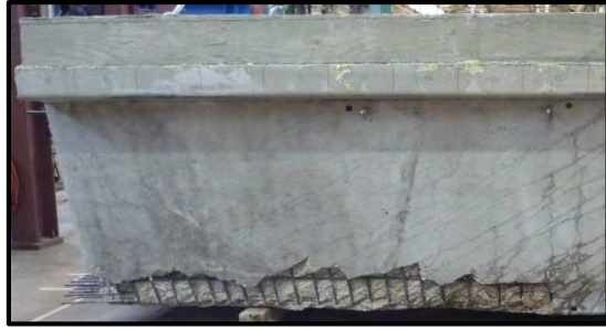
(B) Horizontal shear failure in Texas U54
