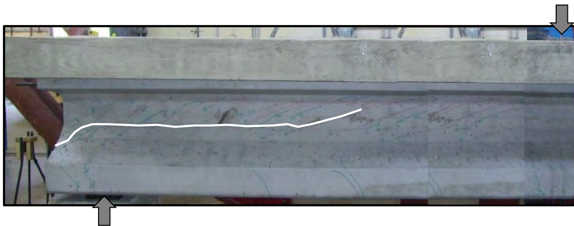
Figure 7-18: Tx28-I-D cracking observed at failure.
