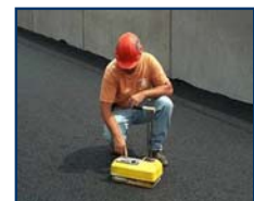
After Compaction is Complete
