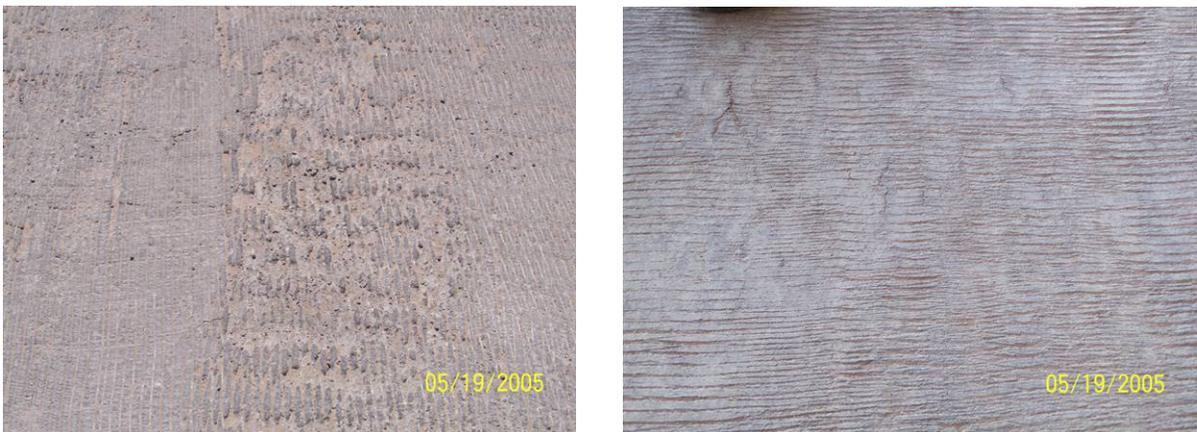
*Figure 1.1: Concrete pavements with 50% slag exhibiting longitudinal cracking (M. Won)*
