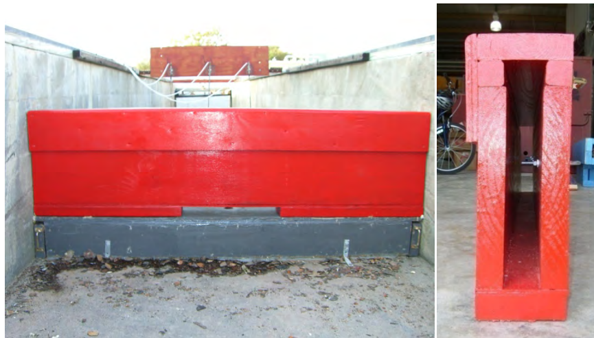
Figure 3.15: T221 Bridge Rail
