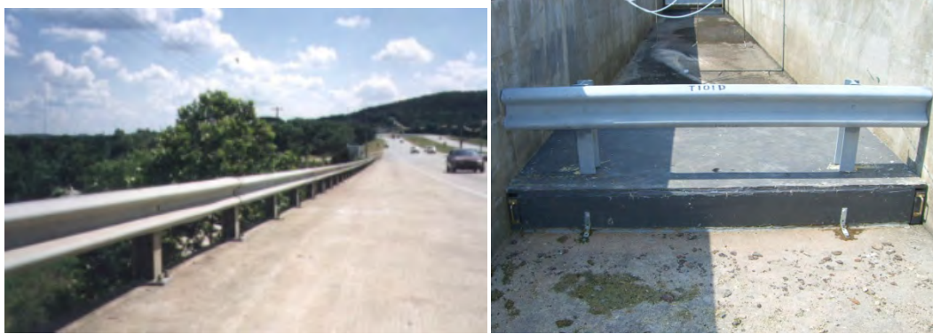
Figure 3.12: T101 Bridge Rail
