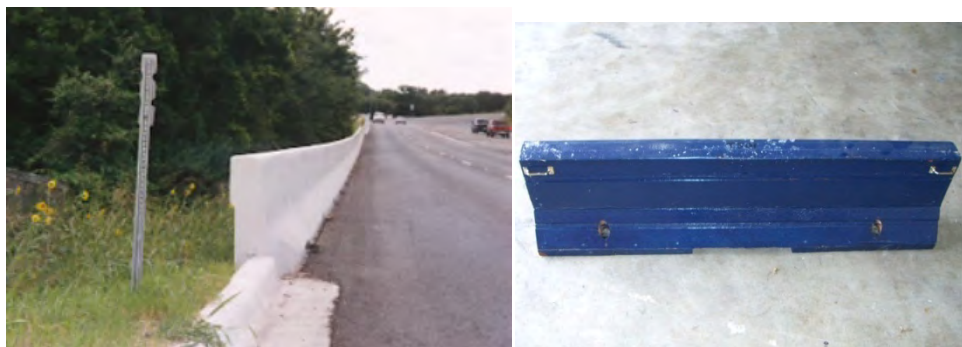
Figure 3.13: T501 Bridge Rail
