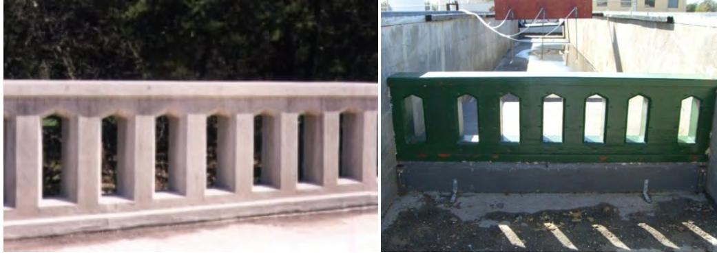
Figure 3.17: T411 Bridge Rail
