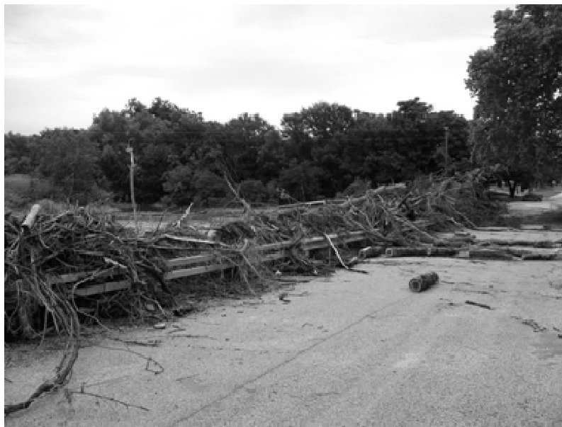
Figure 6.1: Example showing debris accumulation at a bridge crossing
