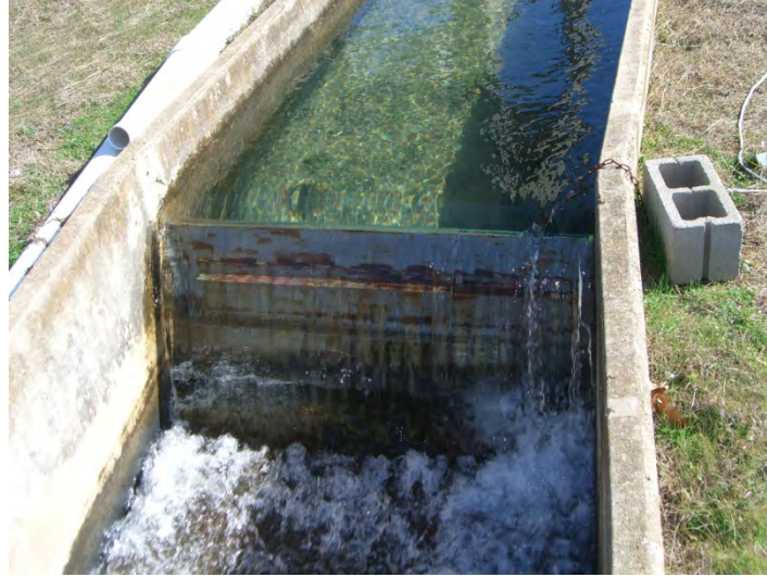
Figure 3.8: Discharge Weir
