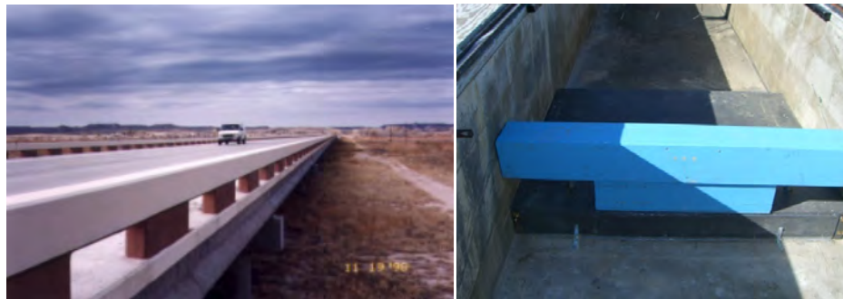
Figure 3.11: T203 Bridge Rail
