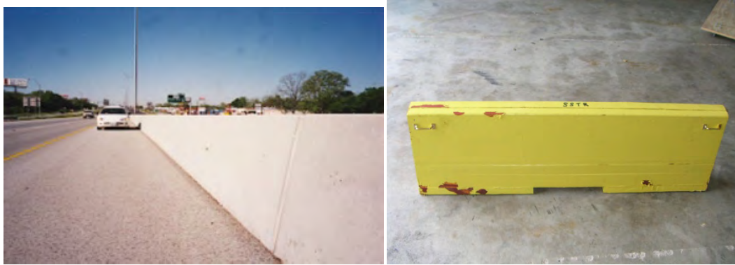
Figure 3.14: SSTR Bridge Rail
