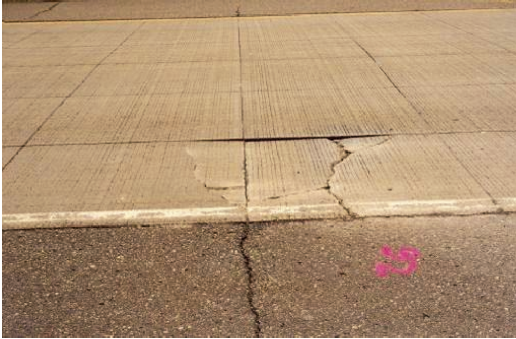
Figure 2.10: Load-related cracking and surface depression (punchout) near existing transverse crack of test cell 93
