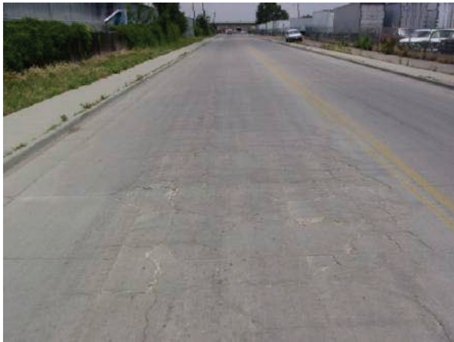
Figure 2.18: Distressed Area at Stop Sign Approach
