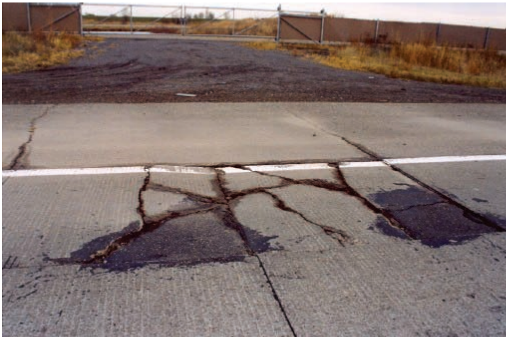
Figure 2.11: Load-related cracking and large surface depression of test cell 93 driving lane
