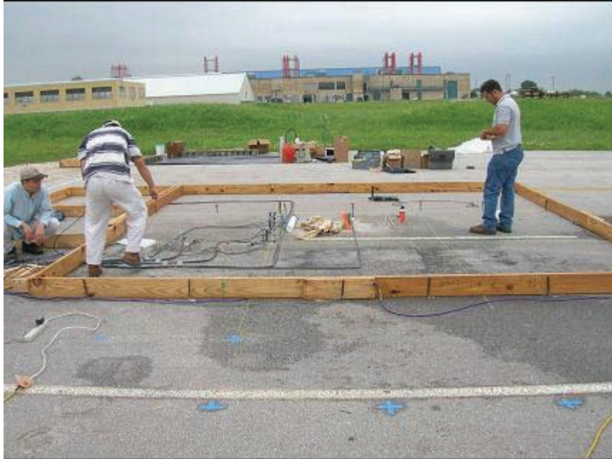
(a) Installation of instrumentations before slab casting
