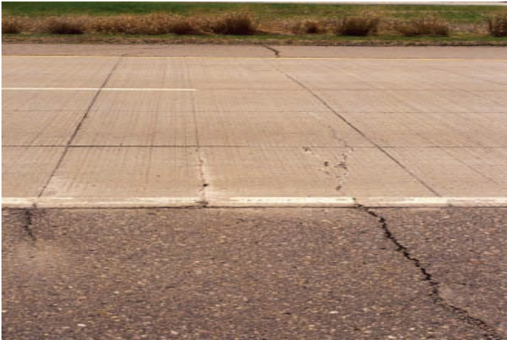
Figure 2.9: Cracks from underlying asphalt layer reflected through UTW overlay in test cell 93
