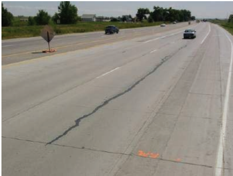
Figure 2.20: Slab Cracking Filled with Asphalt Sealant
