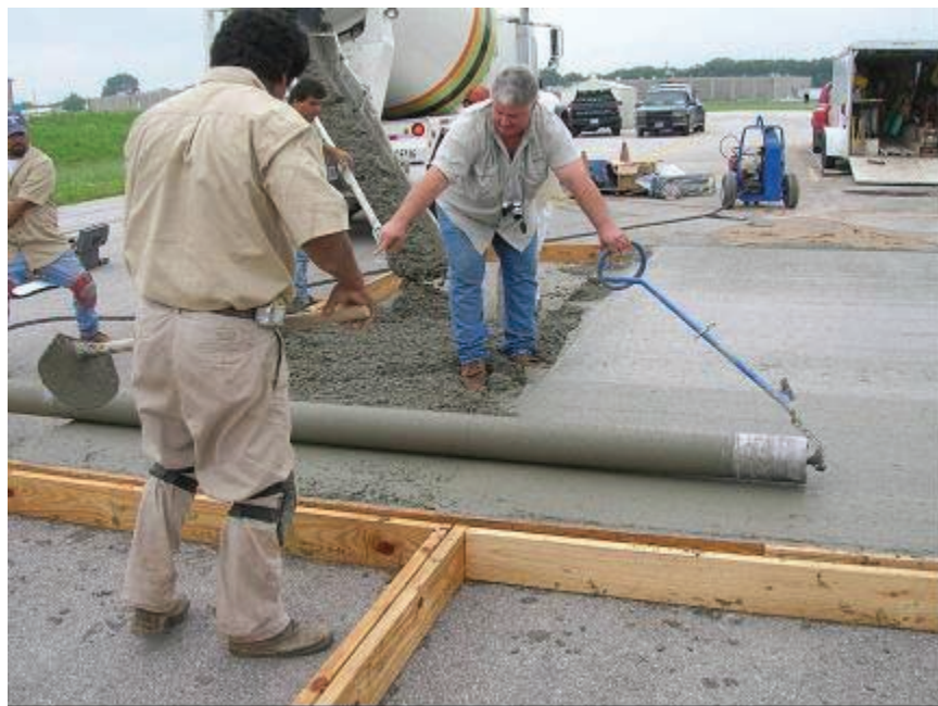
(b) Concrete placement and compaction
