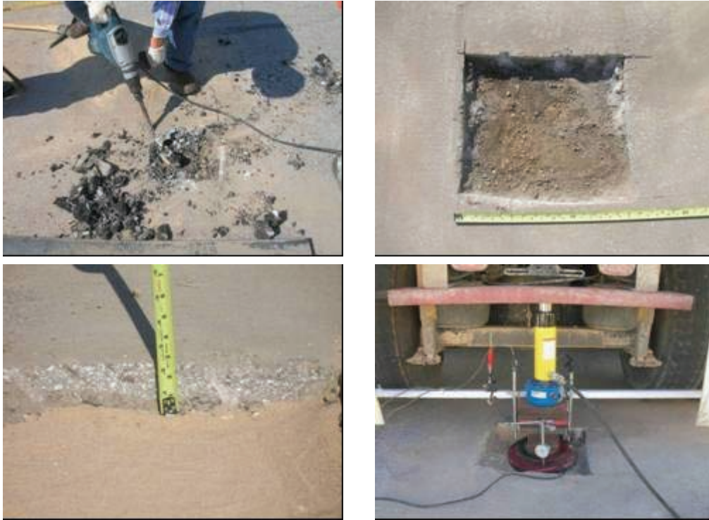
Figure 4.12: Removal of asphalt surface
