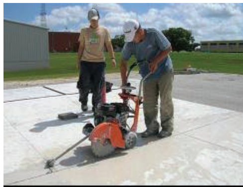
(a) Additional saw cut work
