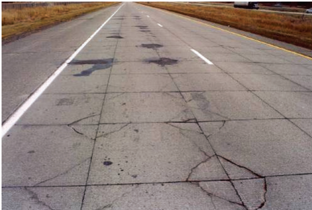
Figure 2.6: Corner cracked areas beginning to punch out in test cell 94
