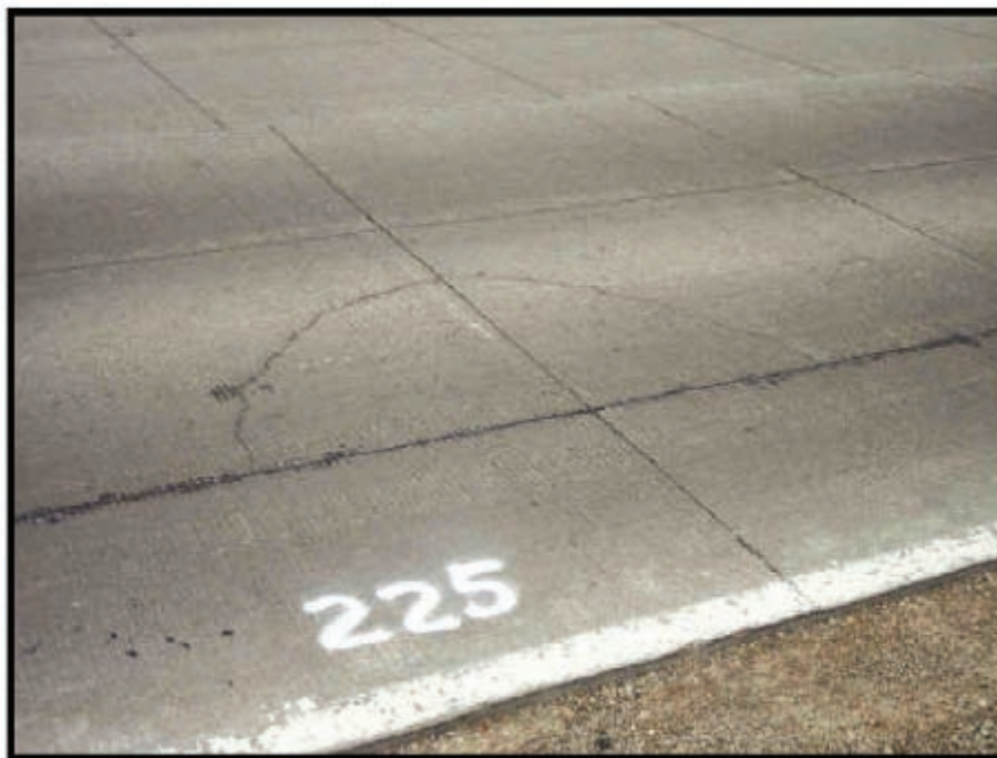
Figure 2.2: Panel Corner Break for Project 4
