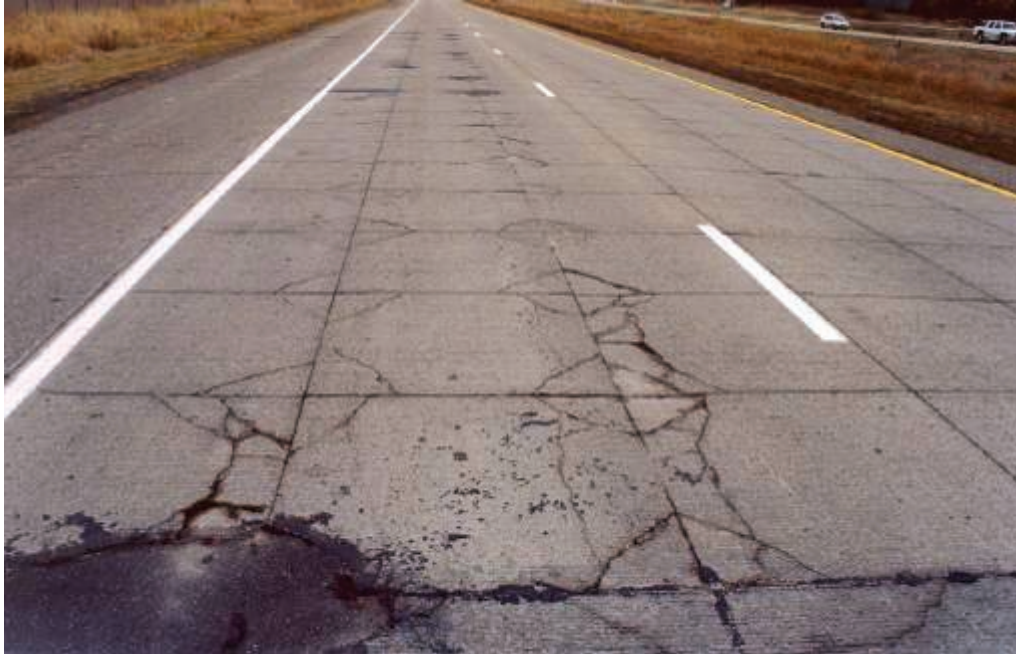
Figure 2.12: Extensive corner cracking of test cell 94, November 2003
