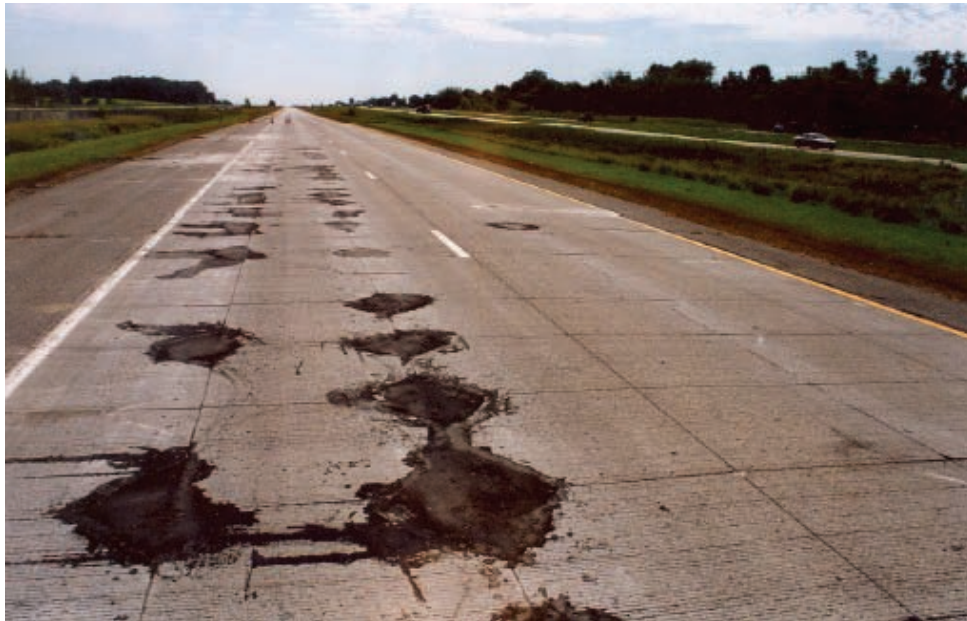
Figure 2.13: Asphalt patching on nearly every panel in the driving lane of test cell 94, September 2004
