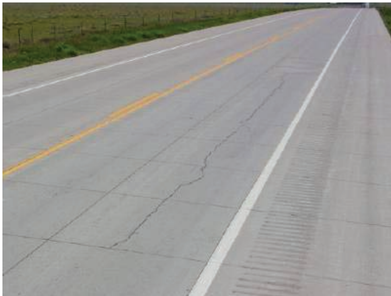
Figure 2.22: Cracked Slabs
