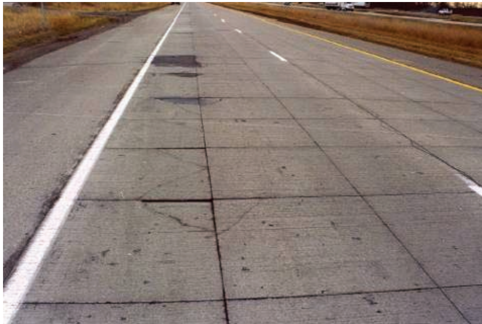
Figure 2.7: Corner cracks near outside wheelpath in test cell 93
