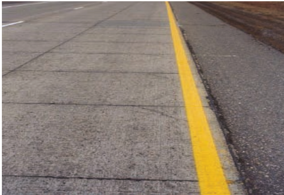
Figure 2.16: Corner cracking on the outside edge of test cell 95, for passing lane, November 2003
