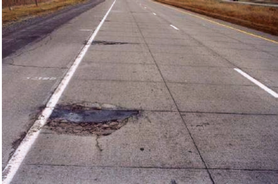
Figure 2.15: Corner cracking on the outside edge of test cell 95, for driving lane, November 2003
