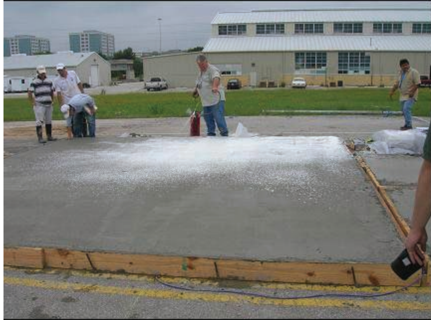
(c) Application of curing compound
