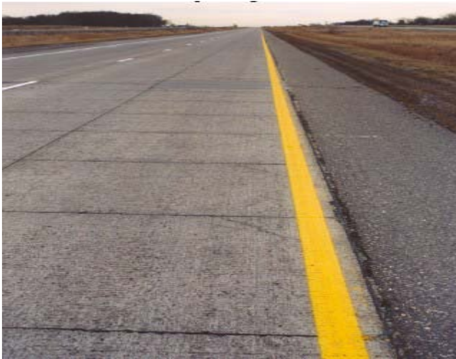
Figure 2.16: Corner cracking on the outside edge of test cell 95, for passing lane, November 2003
