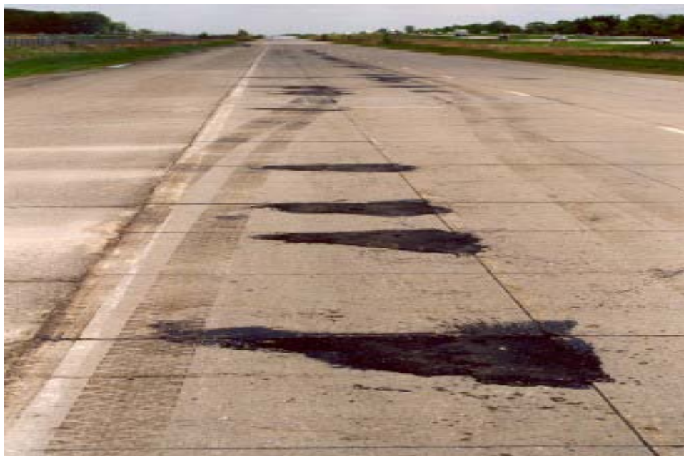
Figure 2.8: Patched corner crack areas near outside wheelpath of test cell 93 driving lane
