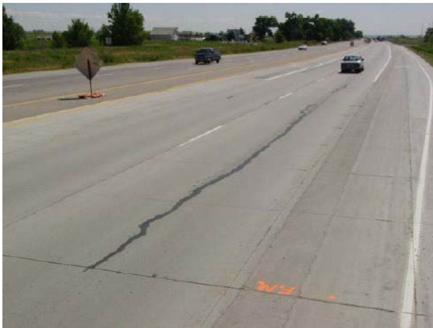
Figure 2.20: Slab Cracking Filled with Asphalt Sealant
