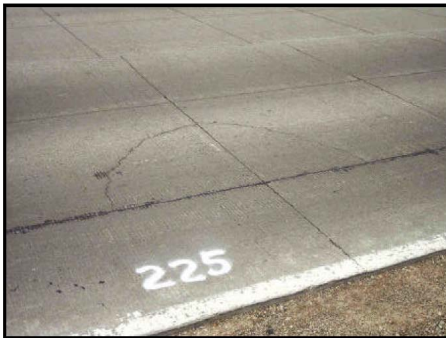
Figure 2.2: Panel Corner Break for Project 4
