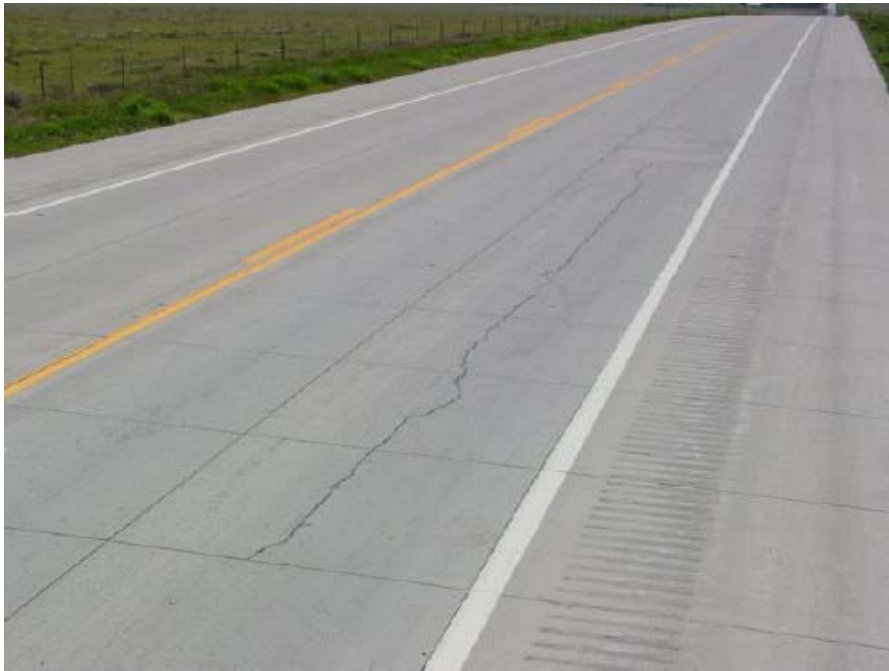
Figure 2.22: Cracked Slabs
