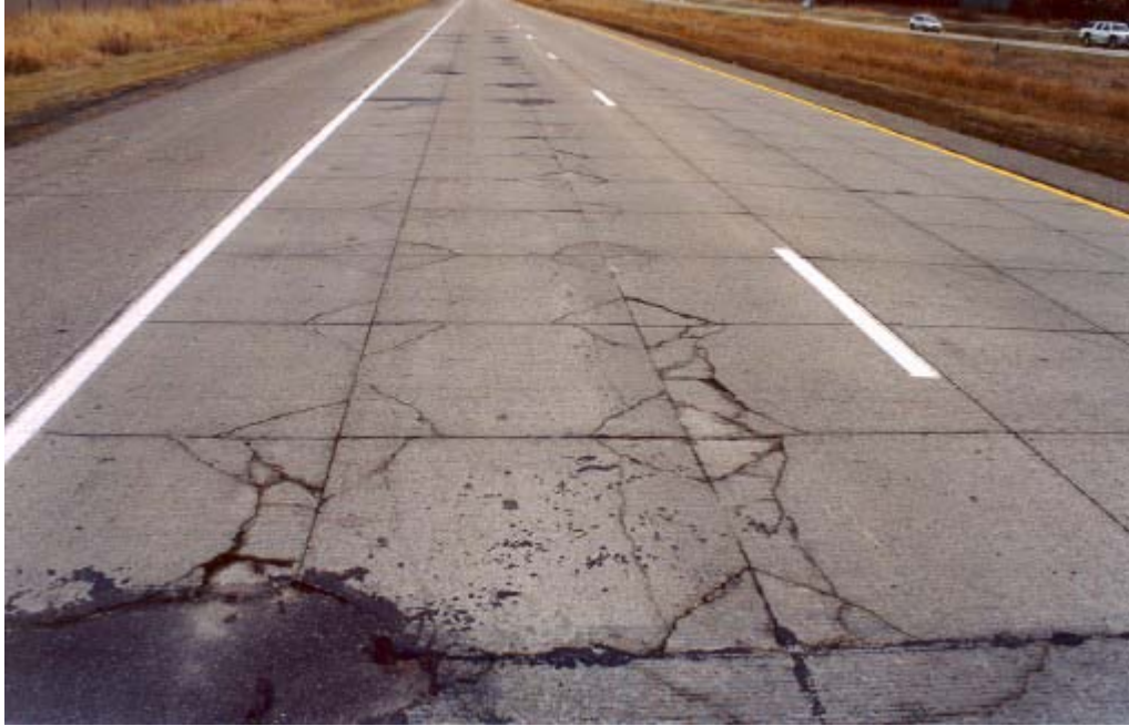
Figure 2.12: Extensive corner cracking of test cell 94, November 2003.
