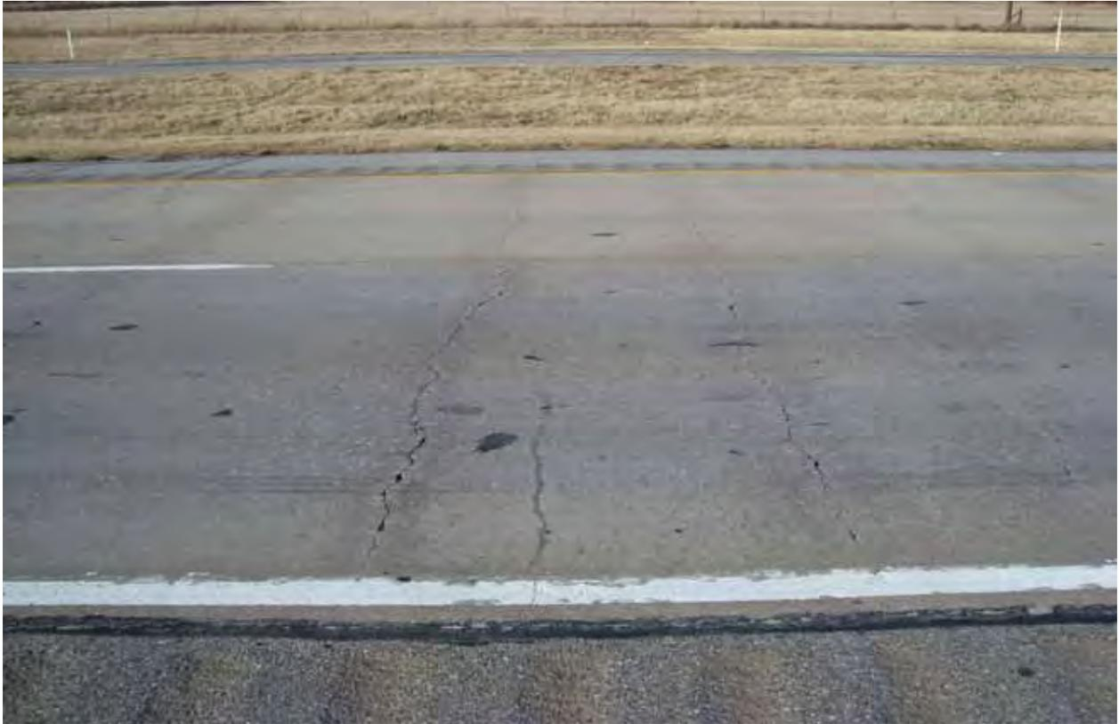
*Figure 4.11: Transverse fatigue crack formed between two old transverse cracks*
