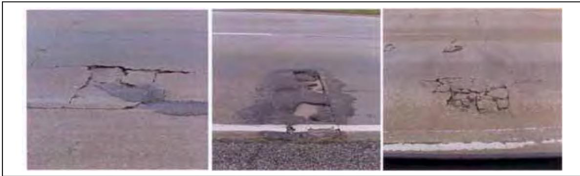
*Figure 4.1: Examples of punchout in TxDOT PMIS Rater's Manual*
