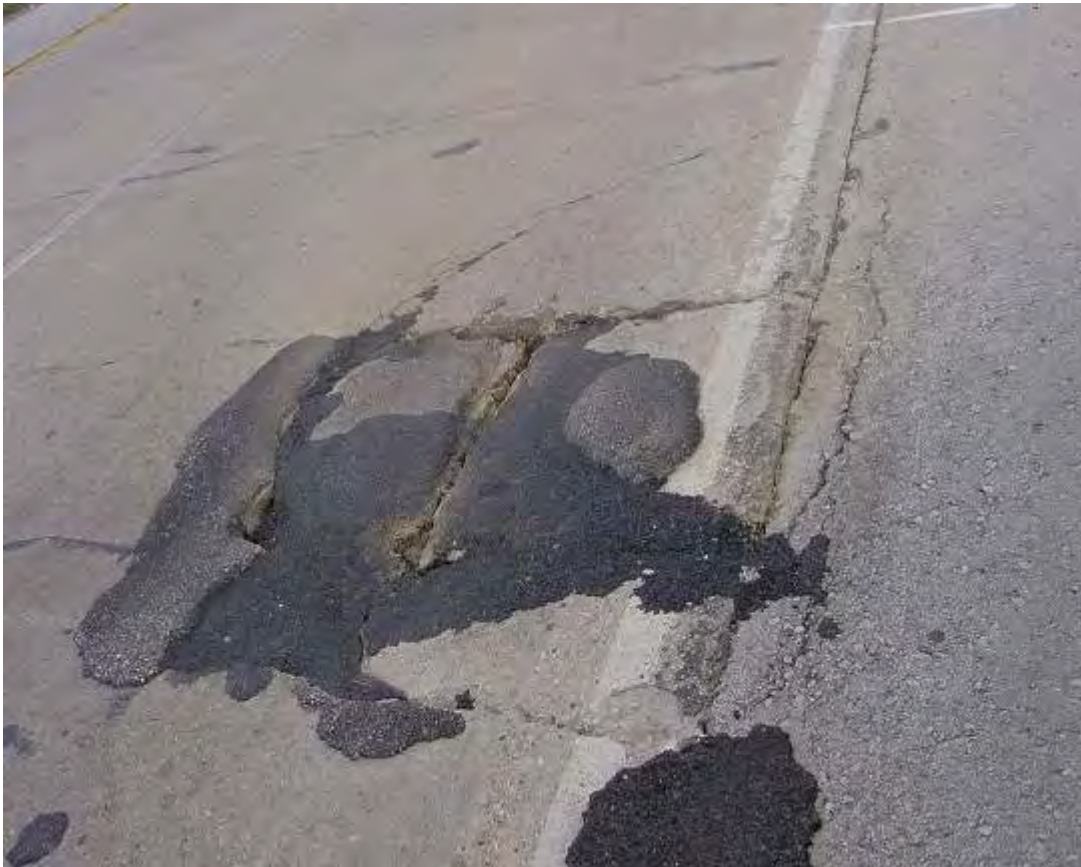
Figure 2.19: Typical edge punchout
