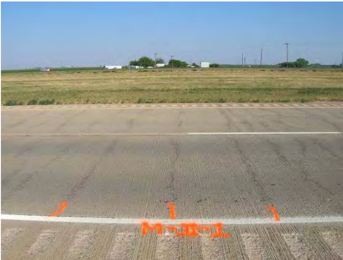
Figure 3.1 Crack M-II-1
