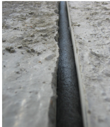
Figure 4.14: Backer Rod between Adjacent Panels
