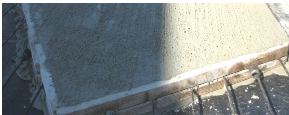
Figure 4.10: Broom Finish Produced in Casting Yard
