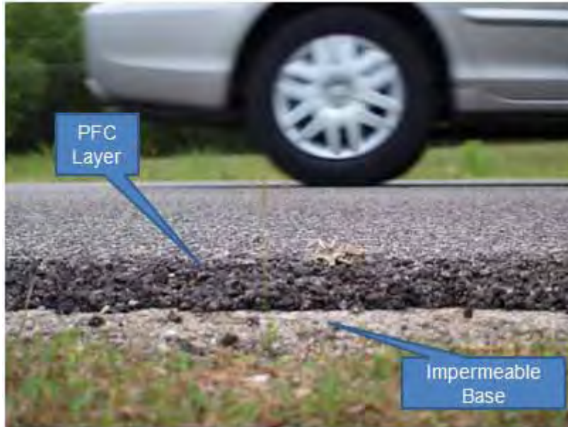
Figure 5-1: Photograph of PFC layer on Loop 360, Austin, Texas
