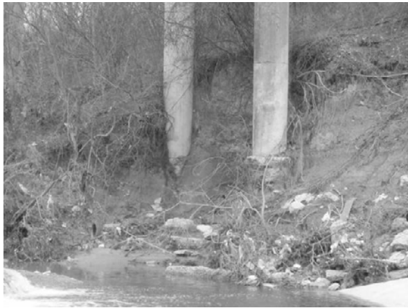
Figure D.26 Exposed foundation (North foundation 2005)
