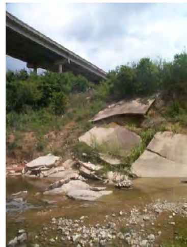
Figure D.19 Failing concrete cover (Northeast bank 1999*)
