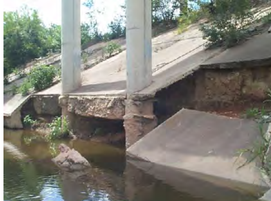
Figure D.23 Partially exposed foundation (South foundation 1999*)
