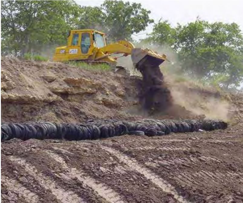
Figure D.43 Placement of soil layer 2001
