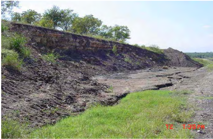
Figure D.39 Failed Slope 2001
