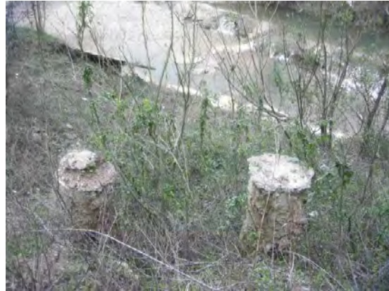
Figure D.25 Exposed drilled shafts (Northeast - southward 2005)
