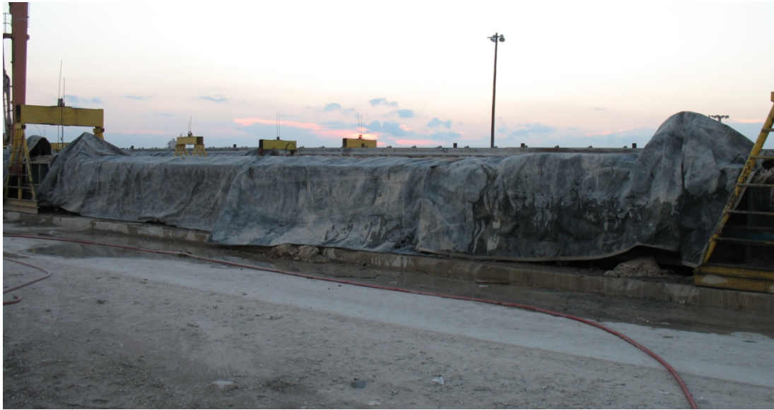
Figure 3.11 Typical Tarp on Beam during Curing Process
