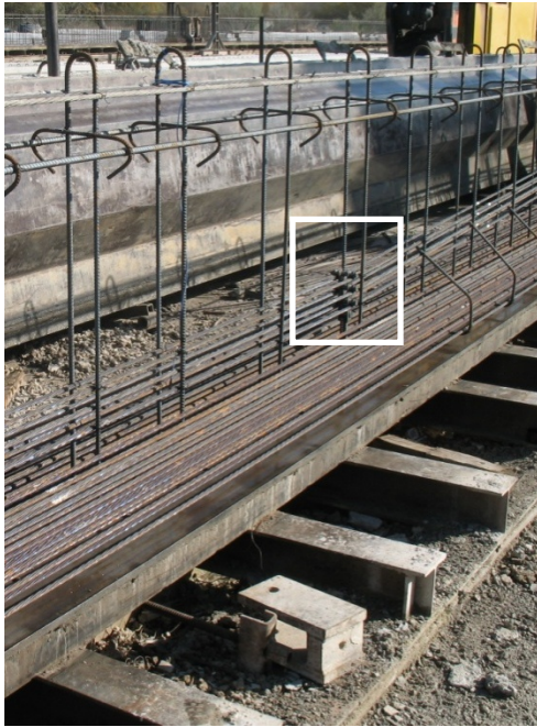
Figure 3.9 Typical Deflected Strands at Precast Plant C
