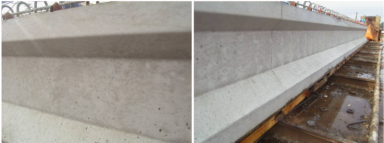
Figure 9.18 Formed Surface Finish of SCC Beam
