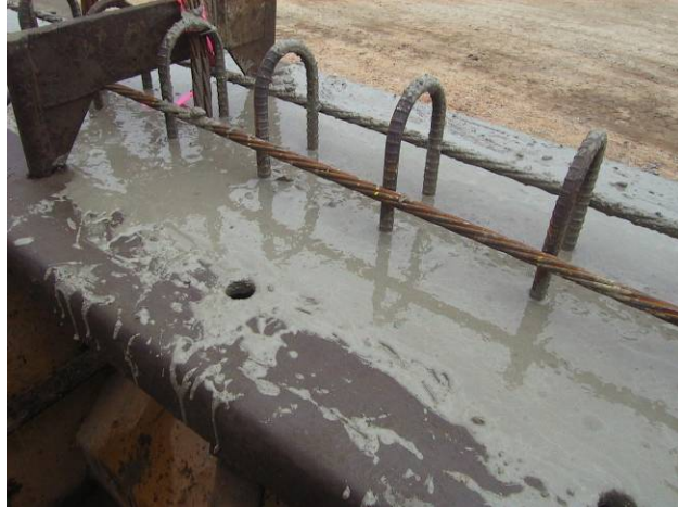
Figure 9.15 Top Surface of SCC Mixture in Form Immediately After Placement
