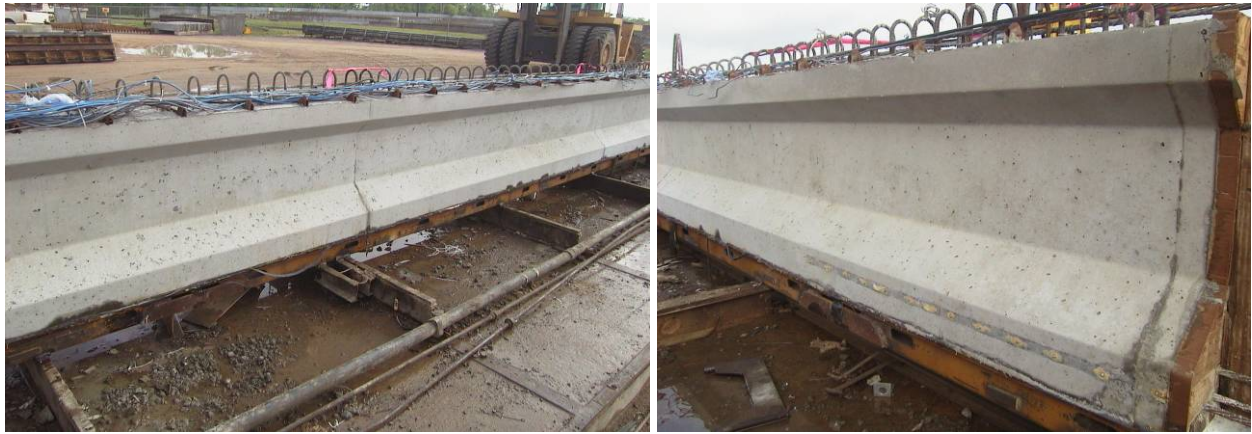
Figure 9.17 Formed Surface Finish of Conventional Placed Concrete Beam
