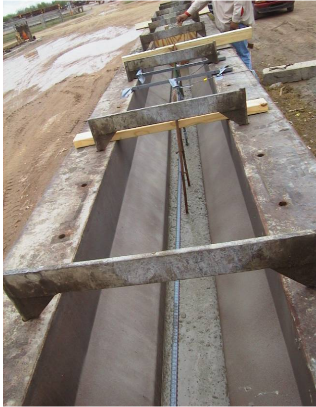
Figure 9.8 First Batch of SCC in Form
