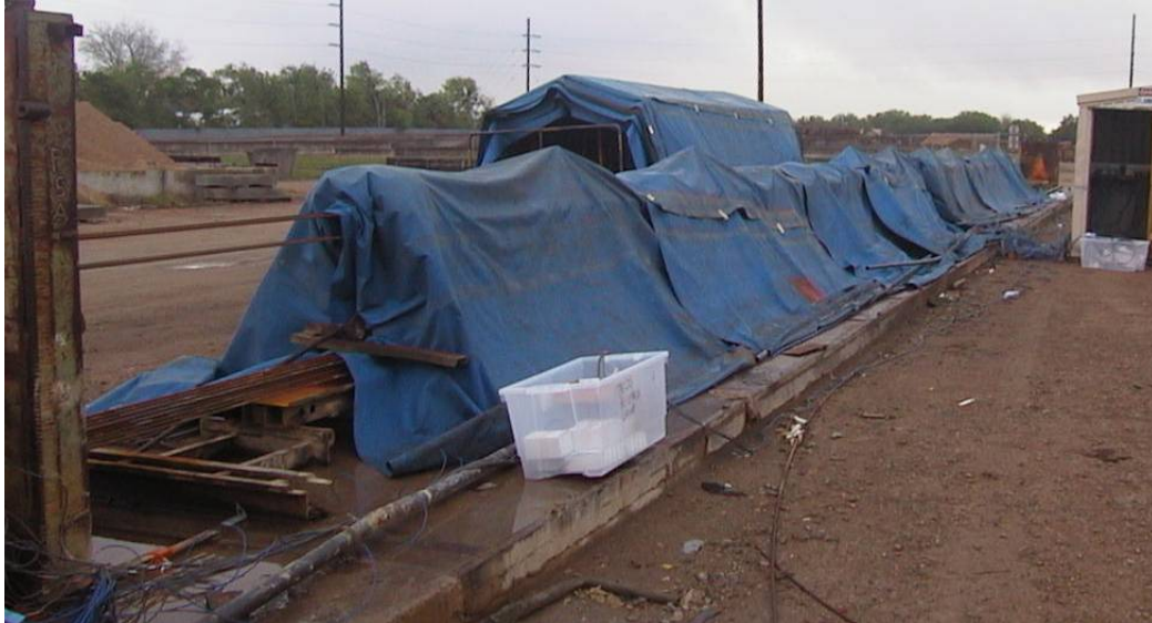
Figure 9.6 Tarp Covering Forms After Placement (Type A Beams)
