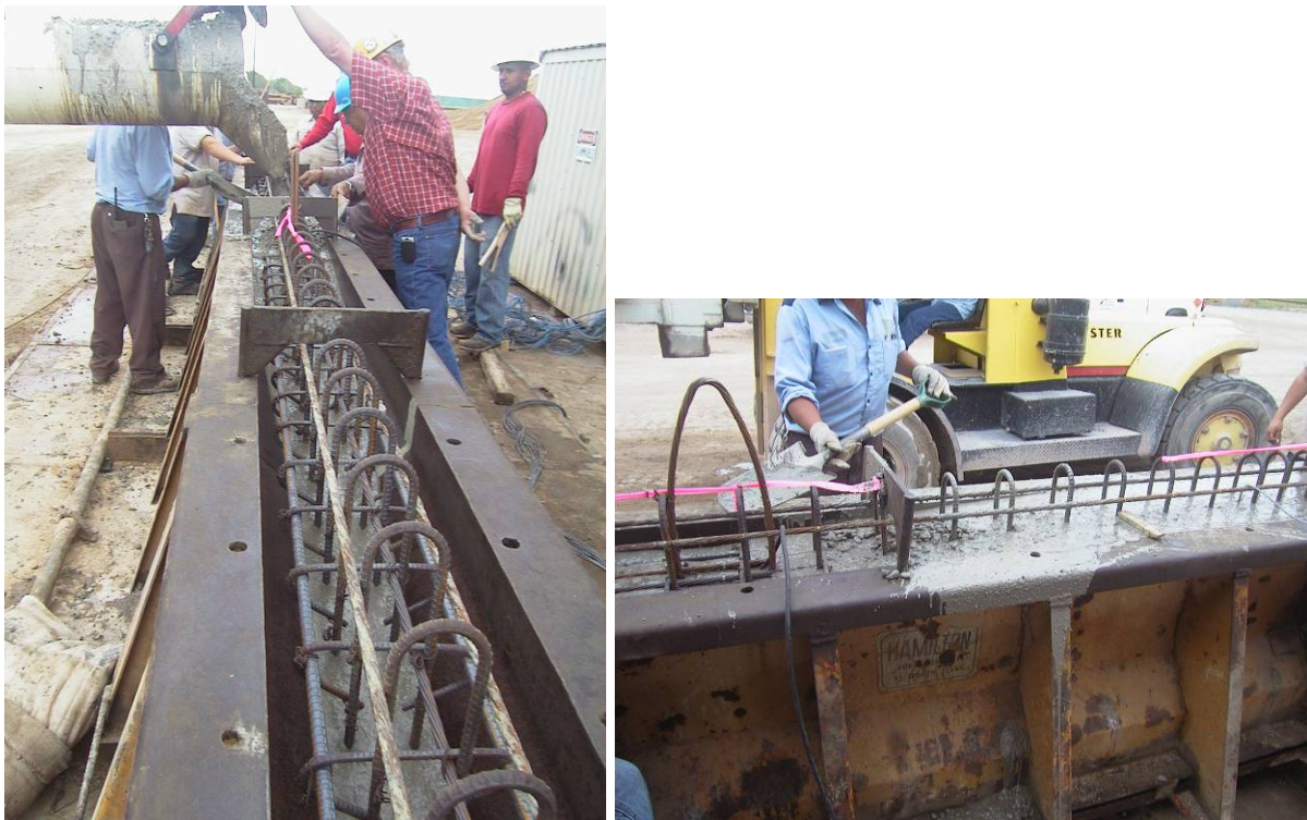
Figure 9.14 Placement of SCC Mixture
