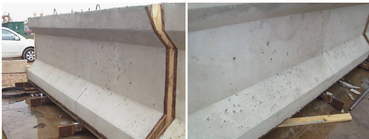
Figure 9.10 Formed Surface Finish of SCC (Left) and Conventional Placed Concrete Beams
