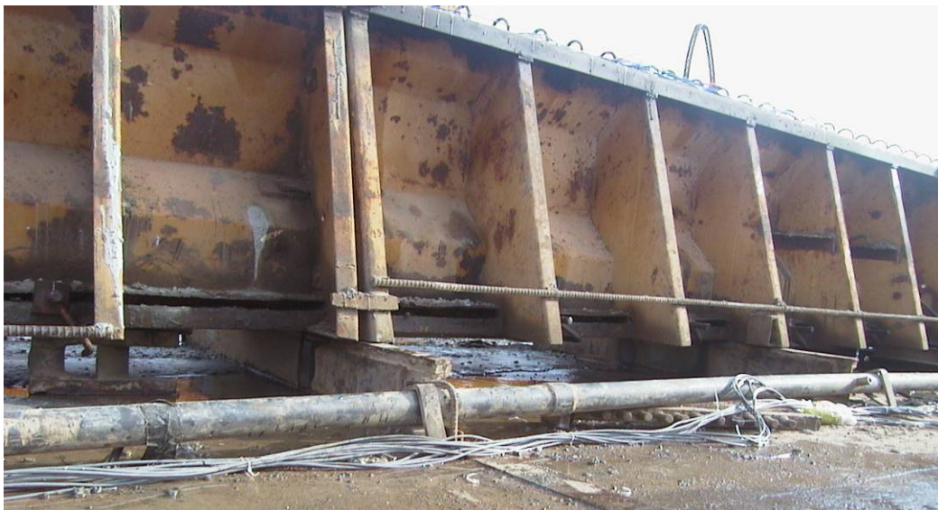
Figure 9.7 Typical Air Space beneath Forms (Type A Beams)
