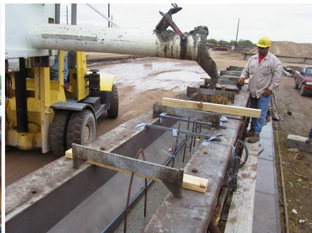
Figure 9.5 Placement of Conventional Placed Concrete (Left) and SCC
