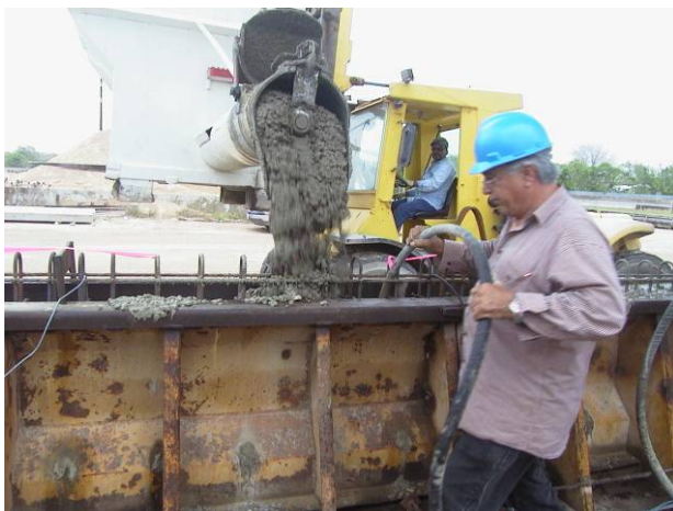
Figure 9.5 Placement of Conventional Placed Concrete (Left) and SCC
