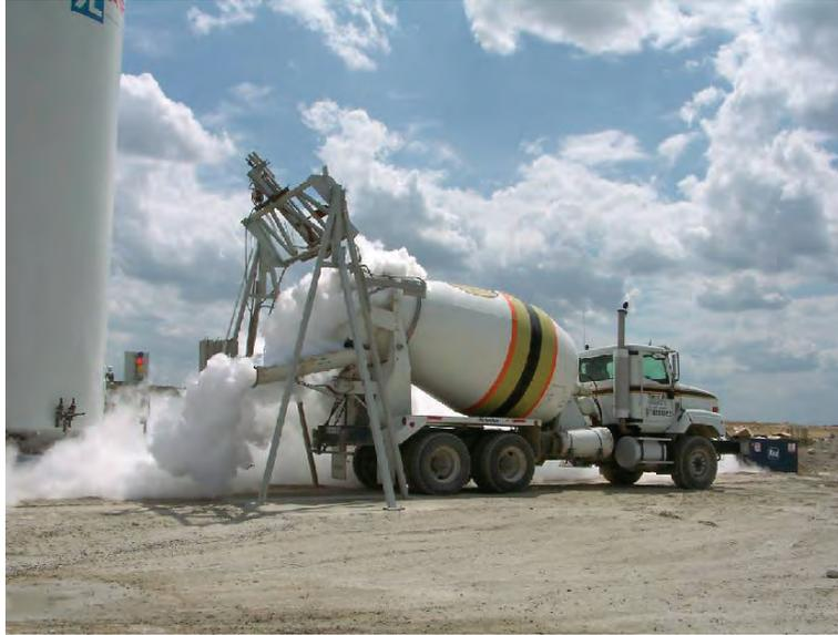
*Figure 2.3 Cooling fresh concrete with liquid nitrogen*
