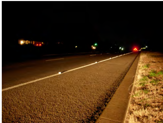
Figure 2.10: Application of RRPM to Supplement Edge Line on Test Section
