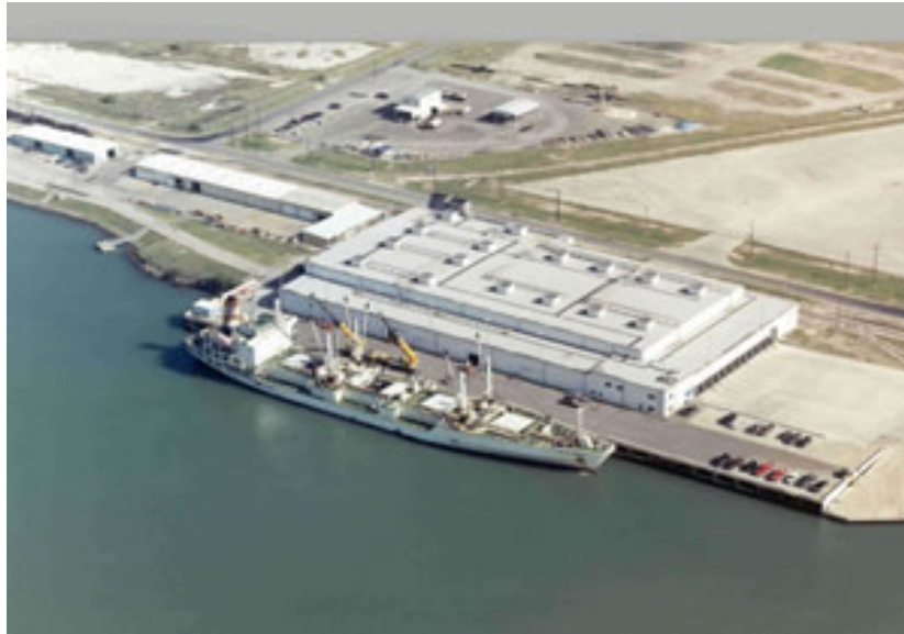
Figure 4.1. Photo of Corpus Christi Cold Storage Facility
