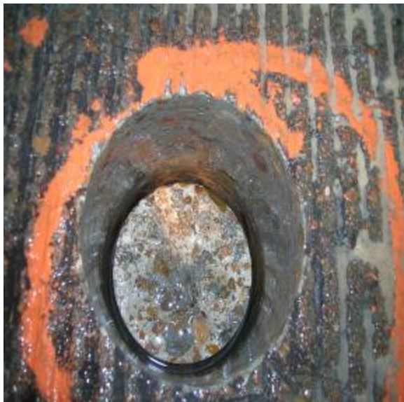
Figure 3.3: (a) Top of the existing concrete showing delamination
