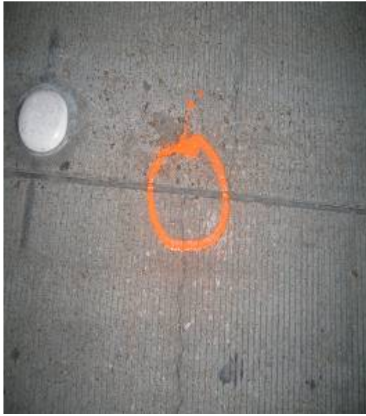
Figure 3.1: (a) Location of coring at delaminated longitudinal warping joint
