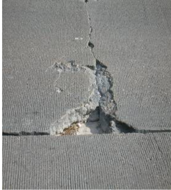
Figure 2.5: Delaminations and severe spalling near longitudinal construction joint
