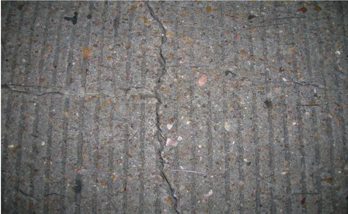
Figure 3.2: Longitudinal cracks and wide transverse crack
