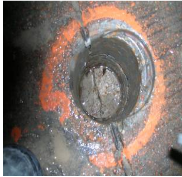
Figure 3.1: (b) Delaminations at the interface between BCO and existing slab
