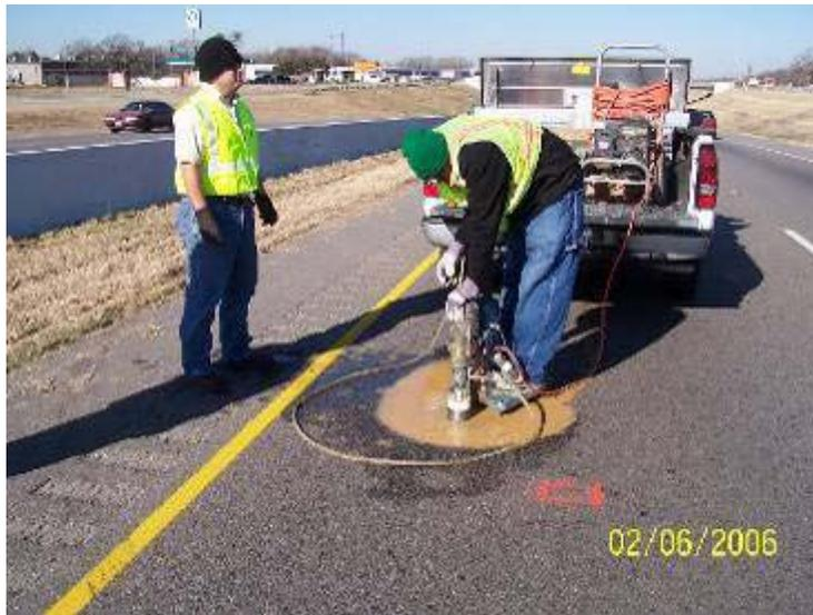
*Figure 2.23 Coring of pavement, WB lanes*
