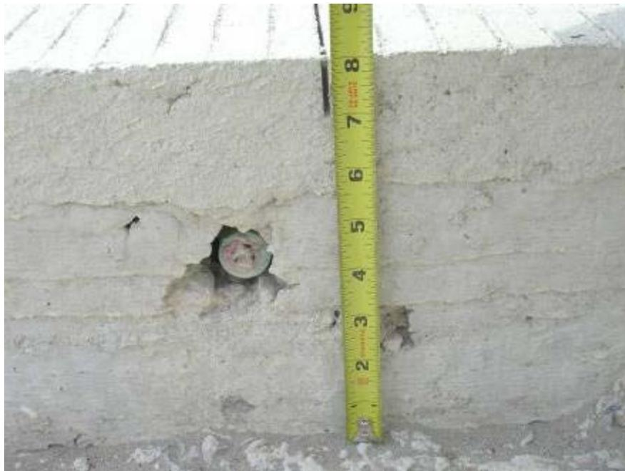
Figure 3.4 Saw cut to induce transverse crack at new CRCP overlay
