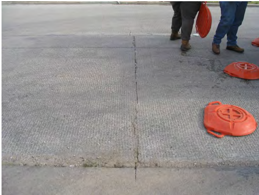
Figure 3.3 Propagation of transverse crack from the curb to the overlay
