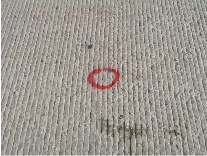
Figure 3.2 Area in good condition, indicating the location of a core sample
