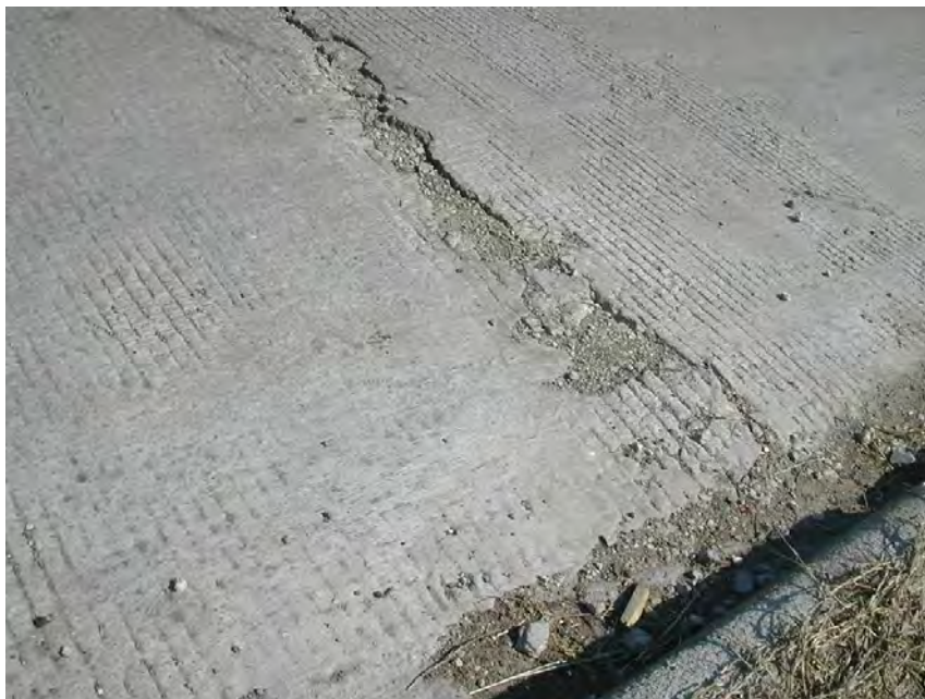
Figure 3.5 Spalled crack
