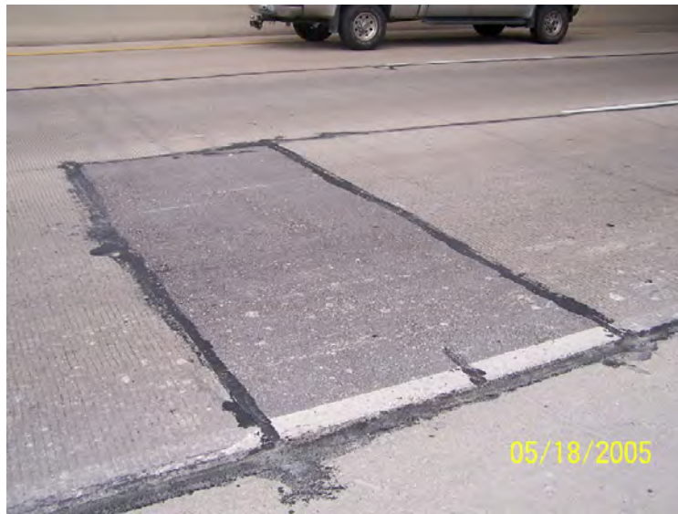
Figure 3.12 AC patch found in pavement section under study
