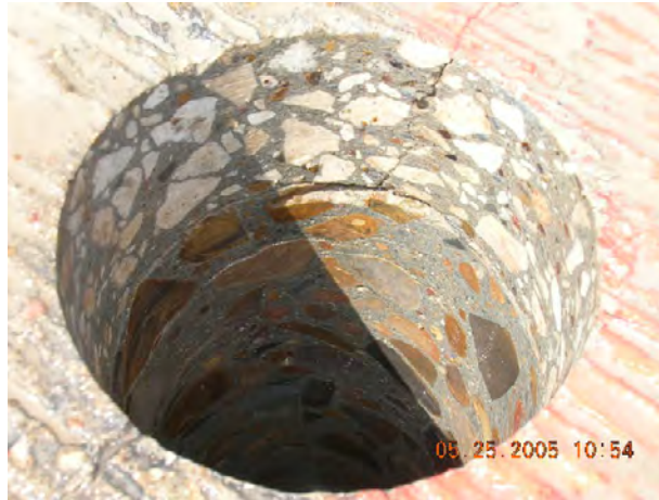
Figure 3.17 Hole in the Beltway 8 pavement after a core was drilled
