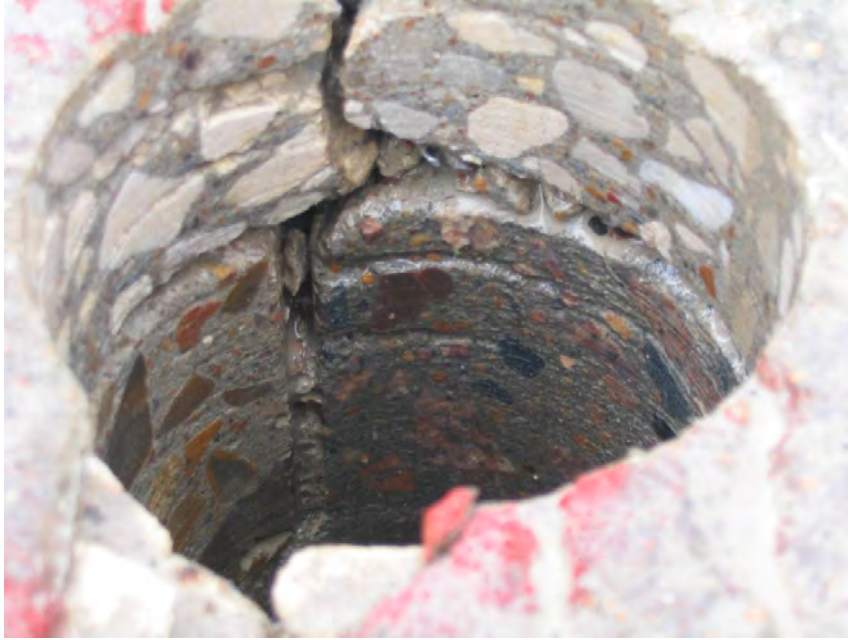
Figure 3.6 Crack reflected from old CRCP to the BCO
