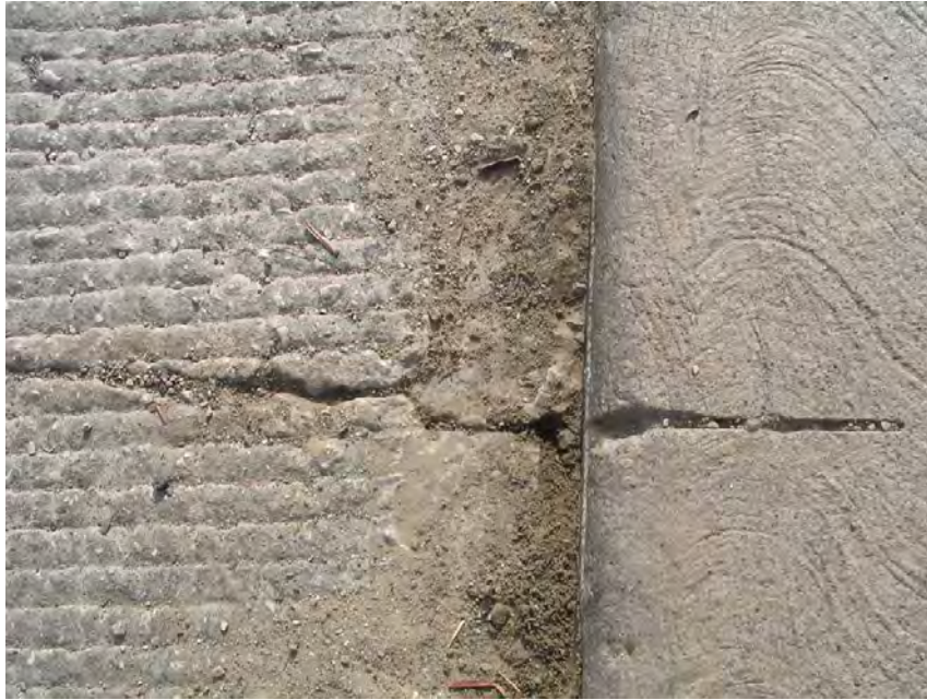
Figure 3.4 Detail of crack propagation from curb to overlay
