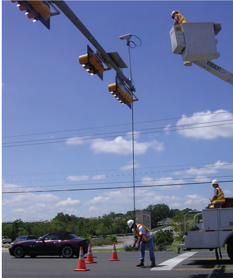
Figure 4.1: Static Load Test
