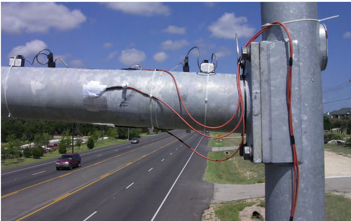
Figure 3.7: Strain Gauges Attached to Mast Arm and Shielded Cables
