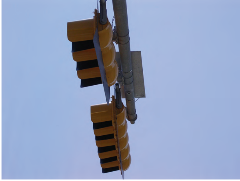
Figure 4.10: The traffic signals have rounded backs and are below the mast arm
