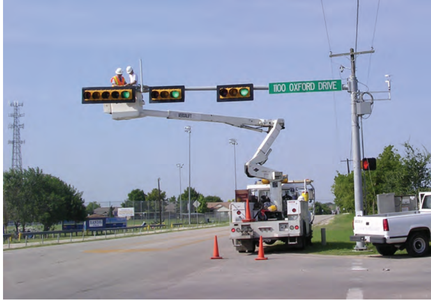
Figure 4.11: A bucket truck is utilized to pluck the structure
