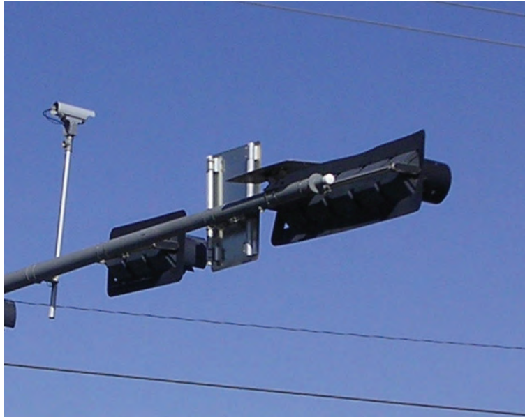
Figure 4.43: Traffic signals with V-shaped backs attached to mast arm
