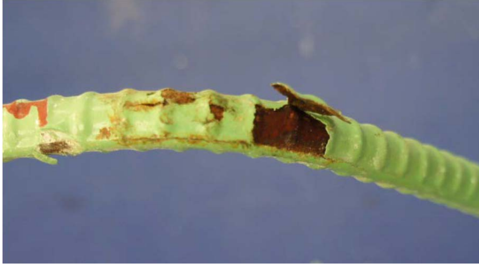
Figure 5.14 – Epoxy-Coated Mild Steel Reinforcement Corrosion
