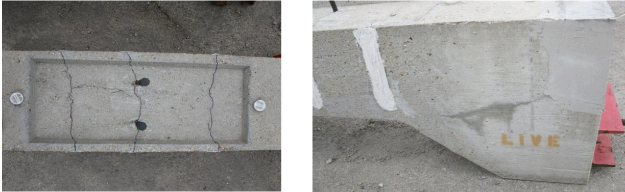
Figure 5.11 – Cracking across Ponding Region (left) and at Corbel (right)
