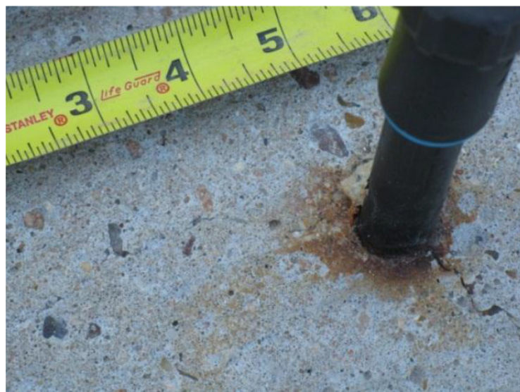
Figure 5.10 – Staining at Grout Vent
