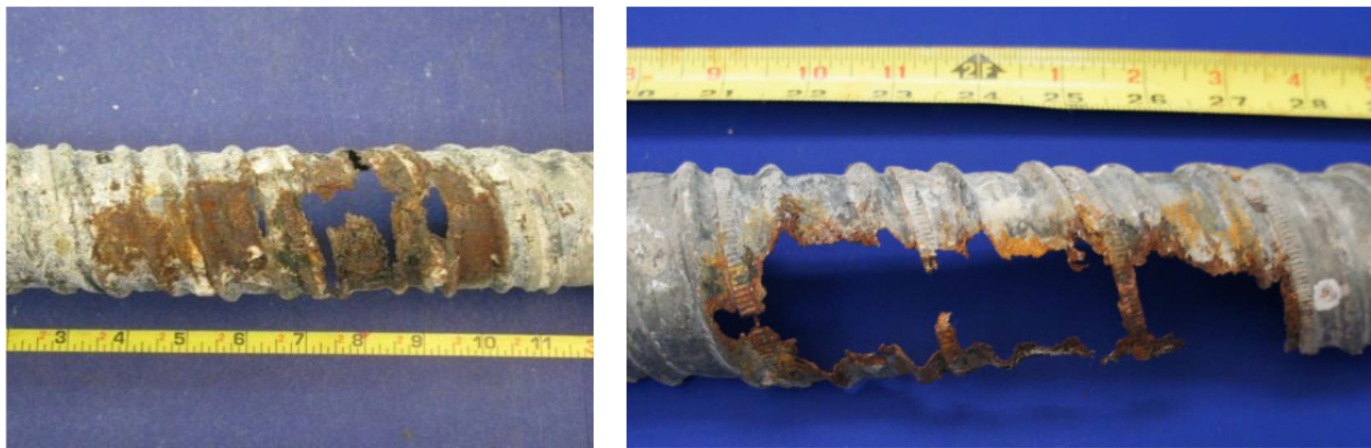
Figure 5.16 – Galvanized Duct Corrosion with Severe Pitting
