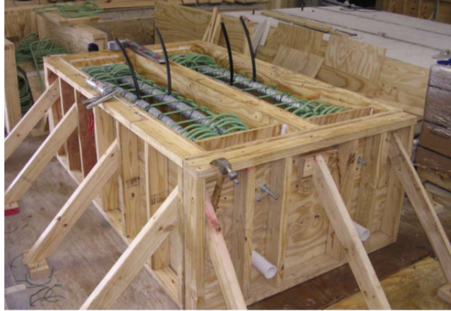
Figure 2.21 – Specimen Reinforcement Cage Prior to Concrete Placement
